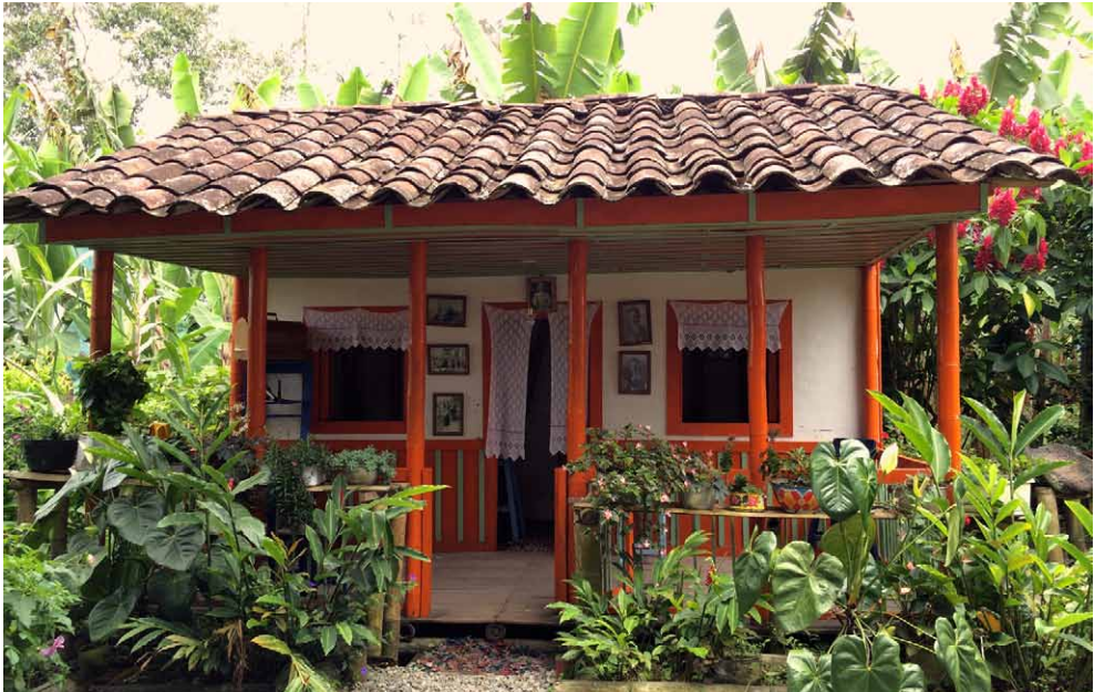
Figure 10.2. A restored coffee pickers house in Colombia's western coffee region. After coffee prices went down in the late 1980's, regional governments, together with the well organized coffee sector, aimed to stay afloat by investing in innovation in the sector itself, but also by broadening it and making it part of a tourism development strategy. Photo: Monica Gruzmacher. © ZEF/University of Bonn, Germany.
