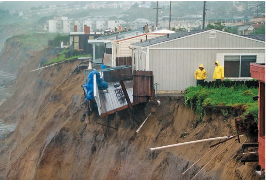
When soil erodes, major destruction can occur, as can be seen here. The backyards of these cliff homes have fallen into the sea in Pacifica, California.
