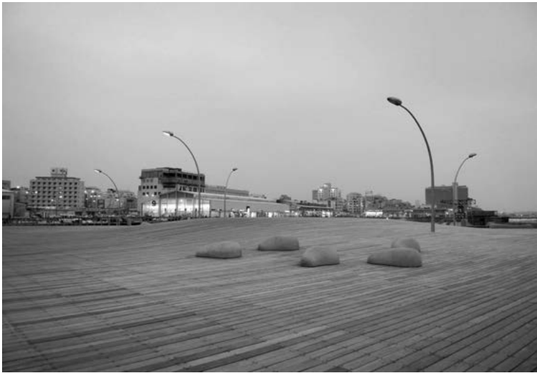
Figure 4.9 Renovation of the Tel Aviv port and promenade by Mayslits Kassif, Architects. (Photo by Adi Brande)
