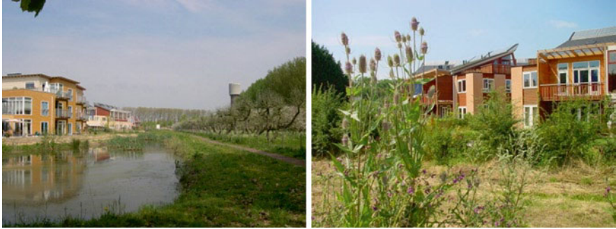
Fig. 12.10 Lanxmeer district with orchard, drinking water extraction area, retention ponds and helophytes ( left ) and housing cluster organised around semi-open court yards ( right ); for more information (Dutch only): www.eva-lanxmeer.nl Accessed March 2011
