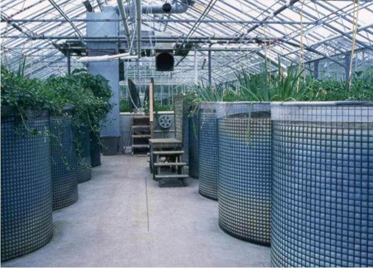
Fig. 2.22 The interior of part of a living machine system: Tanks with rafted plants on the water surface (Photo: H. van Bohemen. Used with permission)
