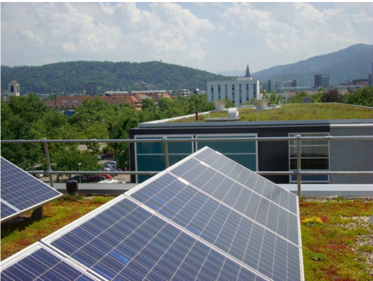
Fig. 2.24 Example of a green roof with solar cell panels (Photo: H. van Bohemen. Used with permission)
