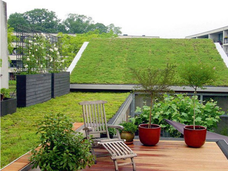
Fig. 2.23 Example of a green roof (Photo: Mrs. T. v.d. Weijer. Used with permission)
