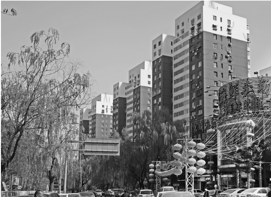
Plate 2.3 The planned residential district of Fangzhuang in Beijing. The residential area was the largest planned development in the 1980s. Although it was built after the economic reform, its building principles followed those of the socialist period.
