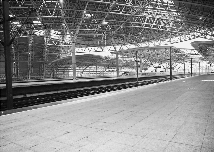
Plate 4.1 The high-speed railway station at Kunshan.
