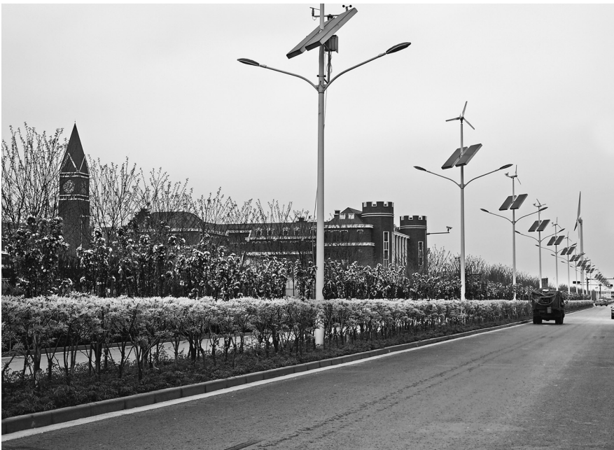
Plate 6.11 The streetscape of Sino-Singapore Tianjin Eco-city, showing that solar panels have been used for street lights. The eco-city presents various technological fixes to advance the low-carbon agenda. The photo shows the buildings of an estate called 'British Land' which is designed in the style of a British market town and British castles.
