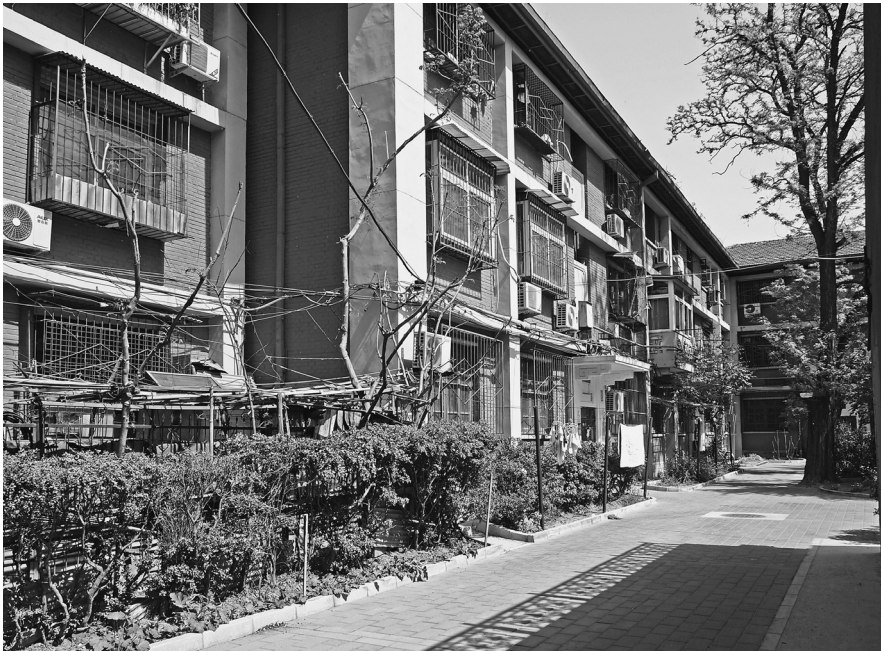
Plate 2.2 Baiwanzhuang residential district in Beijing. It was designed on the principle of the Soviet ‘superblock,’ which located large extended buildings along the streets; there is an internal space encircled by the residential buildings at the edge. Owing to its convenient location and solid building structure, Baiwanzhuang was developed as one of the staff living quarters of the central government. In 2014, the district was demolished.
