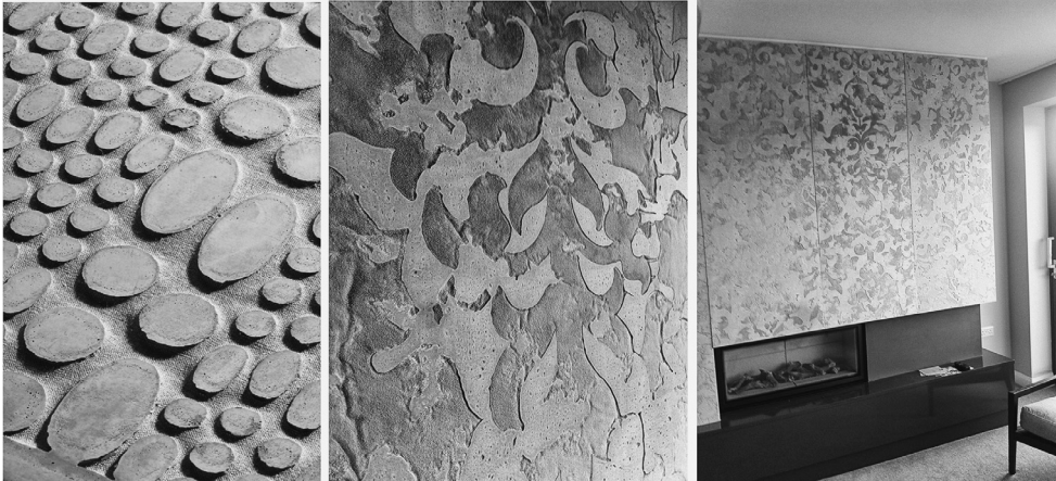
Figure 35.1 Linen concrete. This shows linen permanently co-forming the surface with concrete. This has become known as 'vinegar and chips' (left); close up of Velvet concrete surface (Damask design) (middle); Velvet concrete panels installed in private residential setting (right)
