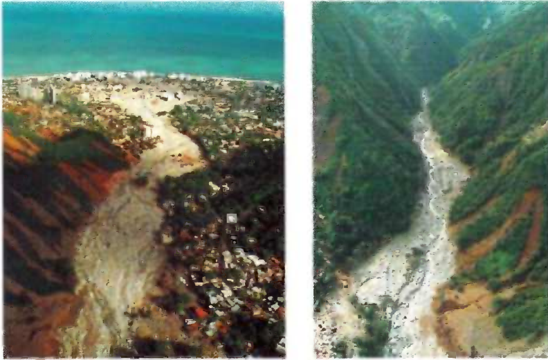
Figure 1 (Chapter 36) Quebrada San Julián upstream of Caraballeda showing evidence of recent debris flows and flash floods. Note the high slope angles, large numbers of debris flow scars, and abundance of new alluvium and colluvium in the channel bed and fan surface.
