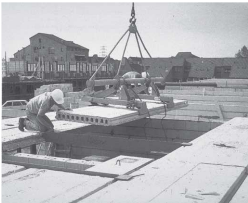
362 Building on the site
