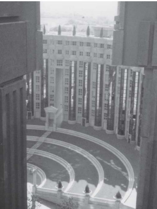
179 Circular residential building by Bofill in Marne-la-Vallée, near Paris. Noises in the heart of the circle are amplified many times by the circular construction (Photograph: Author)
