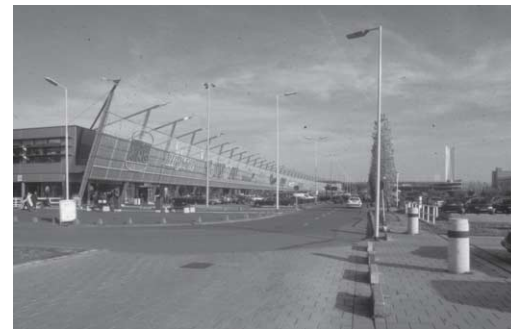
287 Large-Scale Retail Establishment Alexandrium II in Rotterdam North East
