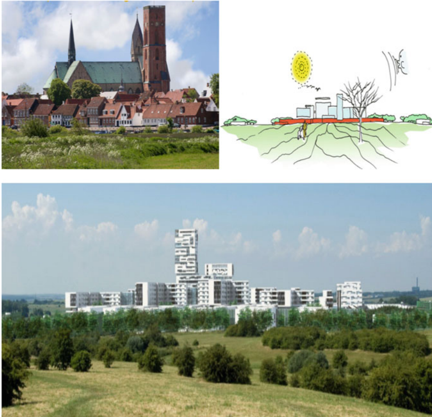
Fig. 4.3 New Aarhus University Hospital, Denmark—Design concept in the image of the Hospital City (Source Møller 2012)
