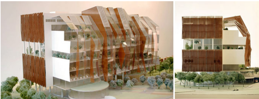
Fig. 4.117 National Heart Centre, Singapore—The hospital has two distinctive façades: the dynamic façade emphasises the public areas as large portions of the skin seem to be peeled back to reveal the inner programmes of the gardens ( Source Broadway Malyan Singapore 2012)
