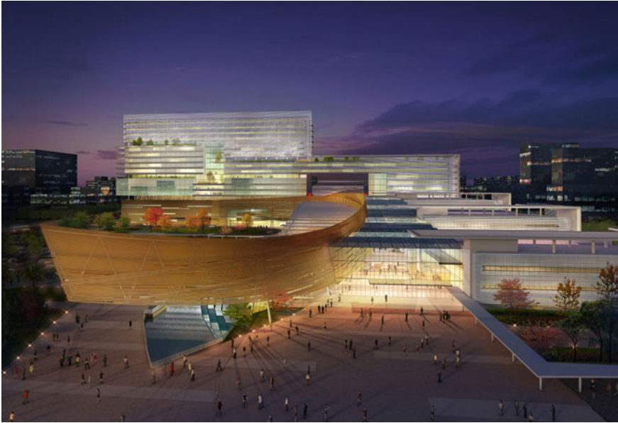
Fig. 4.60 First People's Hospital of Shunde, Foshan District—Main entrance (Source HMC Architects + Foshan Shunde Architectural Design Institute 2012)
