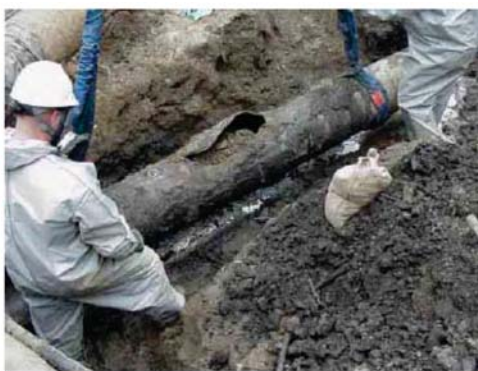
Removal of ruptured pipe section
