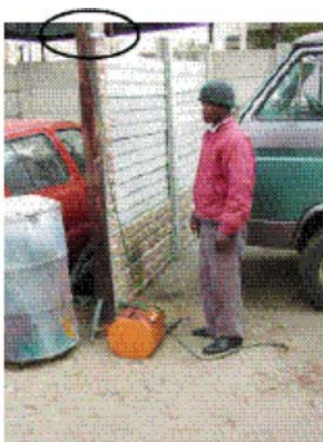
A reconstruction of the scene as it was before the explosion. The welding assistant, the drum, and the welding machine in position. Circle denotes welding position
