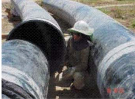
Position of the injured person at the worksite
