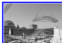
Figure 4. Assembling of an arch segment.
