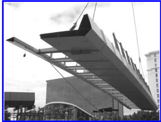
Figure 1. Photograph of box section during the main span erection.
