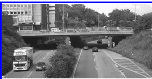
Figure 1. Photo of the bridge.
