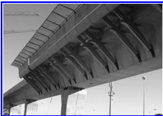
Figure 1. Viaduct under construction at ORTIA airport, showing elevated station platform.
