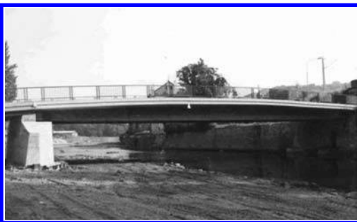
Figure 1. Terrain level side view on the post-tensioned concrete road bridge span and pier in Klodzko after modernization.
