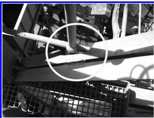
Figure 1. Member Cut-out to accommodate Handrail.
