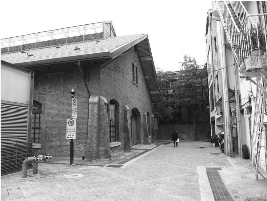
Figure 5.2 The buttresses of the Red House. (Source: the author)
