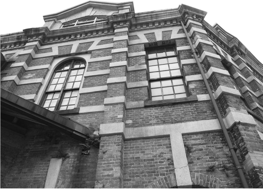
Figure 5.3 The horizontal bands and keystones of the Octagon Building. (Source: the author)
