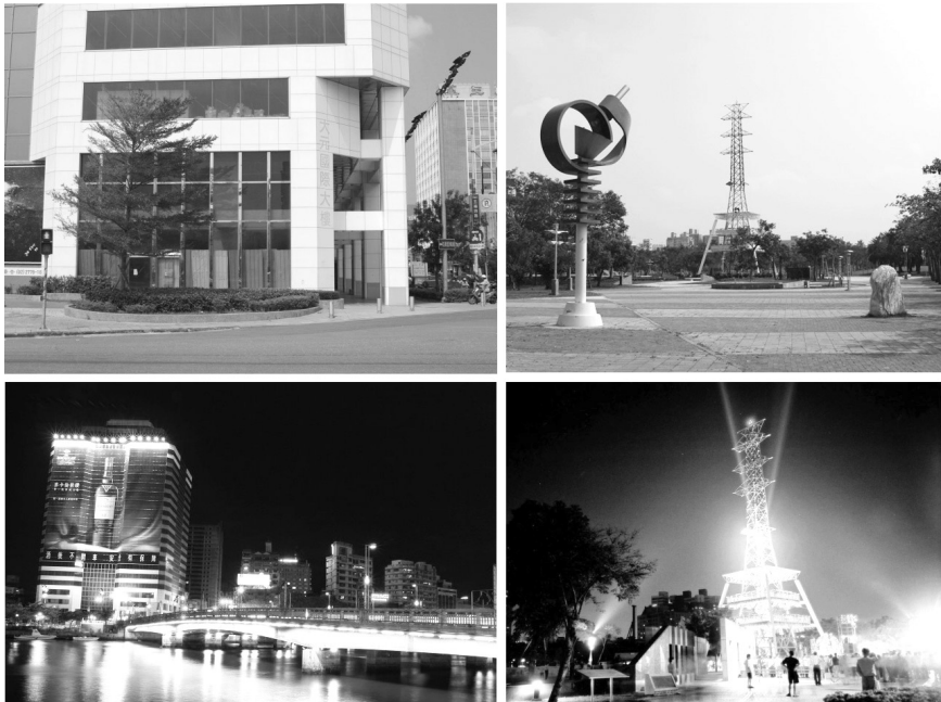
Figure 7.4 Ta Yuen Building, Kaohsiung, Taiwan, 2010, and the Tower of Light, Kaohsiung, Taiwan, 2014. (Source: the author)
