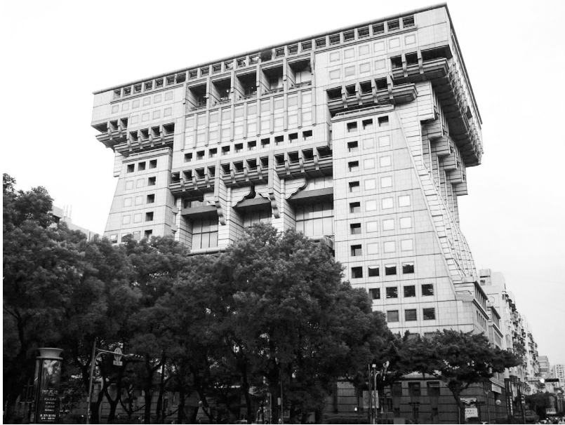
Figure 1.2 Hung Kuo Building, Taipei, Taiwan. (Source: the author)
