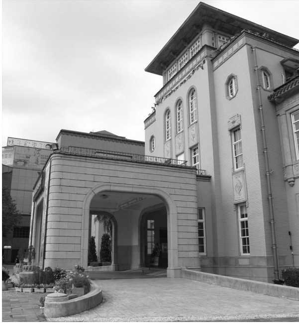
Figure 5.11 The portico at the main entrance of the old City Hall building, Kaohsiung, Taiwan, 2014. (Source: the author)
