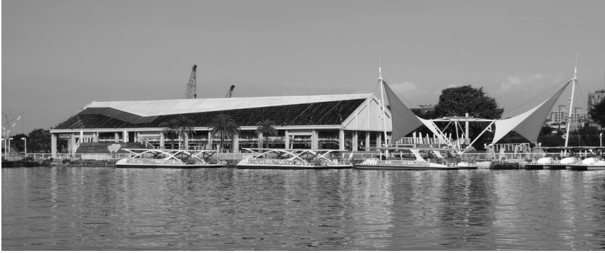
Figure 7.6 Wharf 12, Kaohsiung, Taiwan, 2014. (Source: the author)
