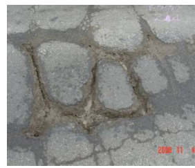
Fig. 4. Massive cracks
