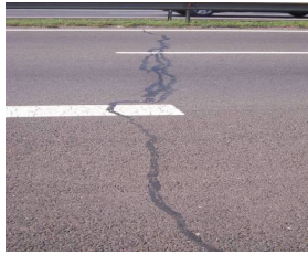
Fig. 5. Surface cracks
