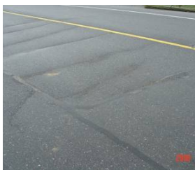
Fig. 2. Transverse cracks
