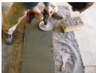
Fig. 2. Equipment used to trowel the slabs
