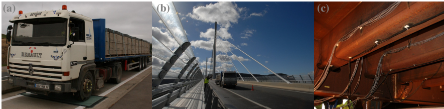
Fig. 6. Pictures of the Millau Viaduct during the experimental measurements. (a) loading truck during weighing; (b) loading truck on the Millau Viaduct; (c) stiffeners and crossbeam with gauges
