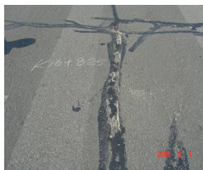
Fig. 3. Massive cracks
