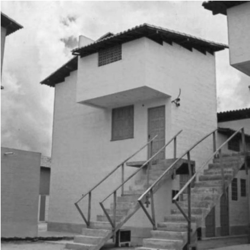
Figure 3.2 Vertical terrace units of the Nova Primavera Estate
