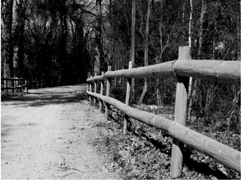
Figure 4.5a Typical Use Class 3 location – fence rails
