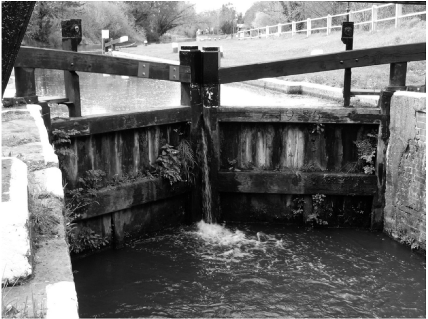
Figure 4.7b Typical Use Class 4 location – lock gates
