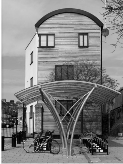
Figure 4.6 Western red cedar used as external cladding (photo courtesy of Canada Wood UK)
