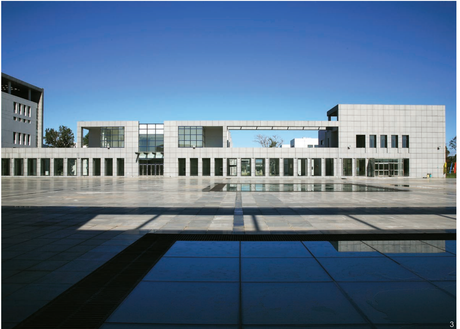
3. Linking vestibule viewed from library roof
