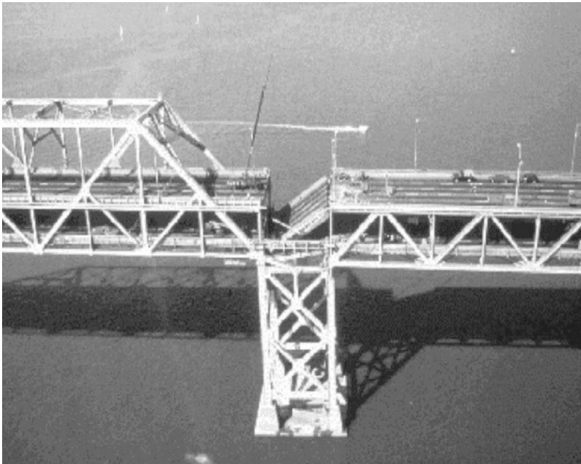
Fig. 1.2. Analysis of San Francisco Bay Bridge. a Photo of East span of Bay Bridge; b Photo of slab that failed during earthquake
