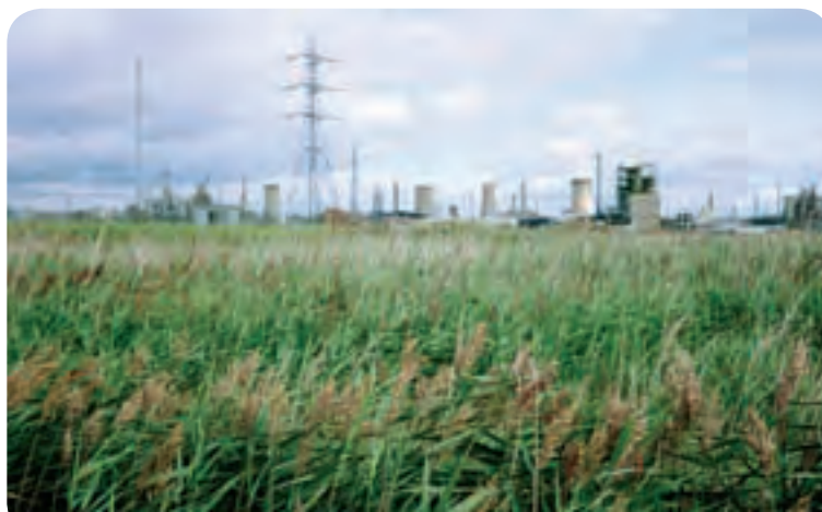
■ Figure 5.22 Chemical waste from an industrial complex is being treated using reed beds. Bacteria and fungi in the reed beds transform a wide range of pollutants into harmless substances.
