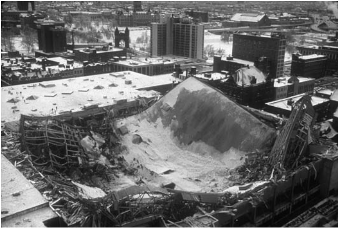
Figure 12.4 The Hartford Civic Center Collapse. Aerial view of collapsed Coliseum roof. Copyright © The Thornton Tomasetti Group and ASCE
