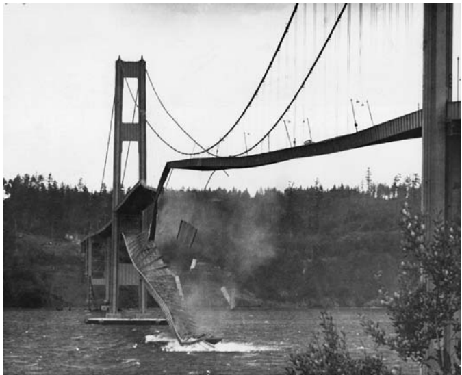
Figure 12.2 Tacoma Narrows Bridge. Bridge midsection crashing into the waters of the Tacoma Narrows — November 7, 1940. Copyright © University of Washington Libraries.
