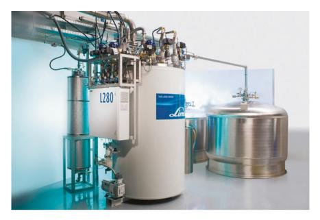
**Fig. 1.3** Modern plant for liquefying the noble gas helium. On the *left* we see the controls and the cold box of the liquefier, on the *right* the storage vessel for liquid helium (*photo* Linde AG)
