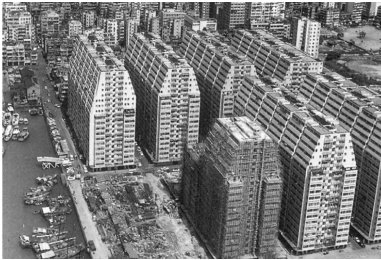
Figure 12.10. High density means very tall buildings built very close together. The street width to building height ratio in this case is 1:3. The tapering at the top of the towers follows the 71.5^\circ obstruction limiting angle based on the Building Regulations of Hong Kong
