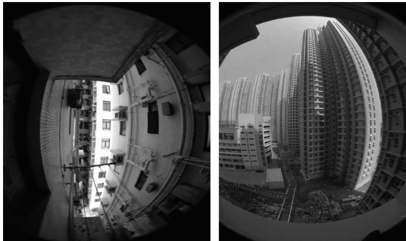
Figure 12.11. A window facing a restricted space that is legal under the Building Regulations. The bit of remaining sky that is otherwise available is blocked by the air conditioners' shelf (left). A window with a tall tower directly opposite does not satisfy the Building Regulations. This is despite the availability of plenty of daylight from one side (right)
