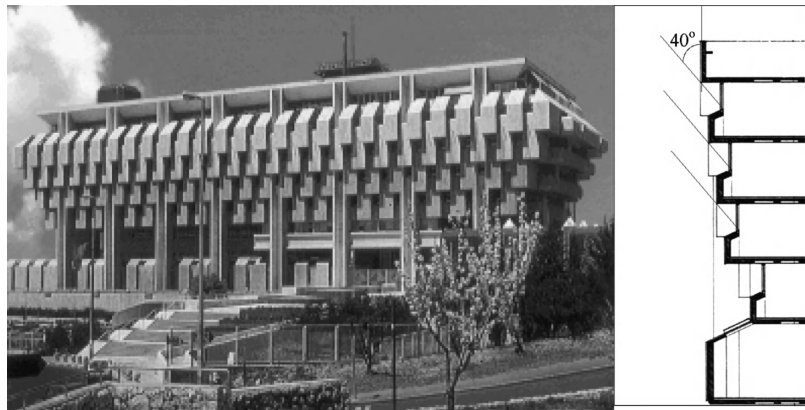
Figure 13.9. Bank of Israel, Jerusalem: Free view (left) and section (right). (A. and E. Sharon Architects)
