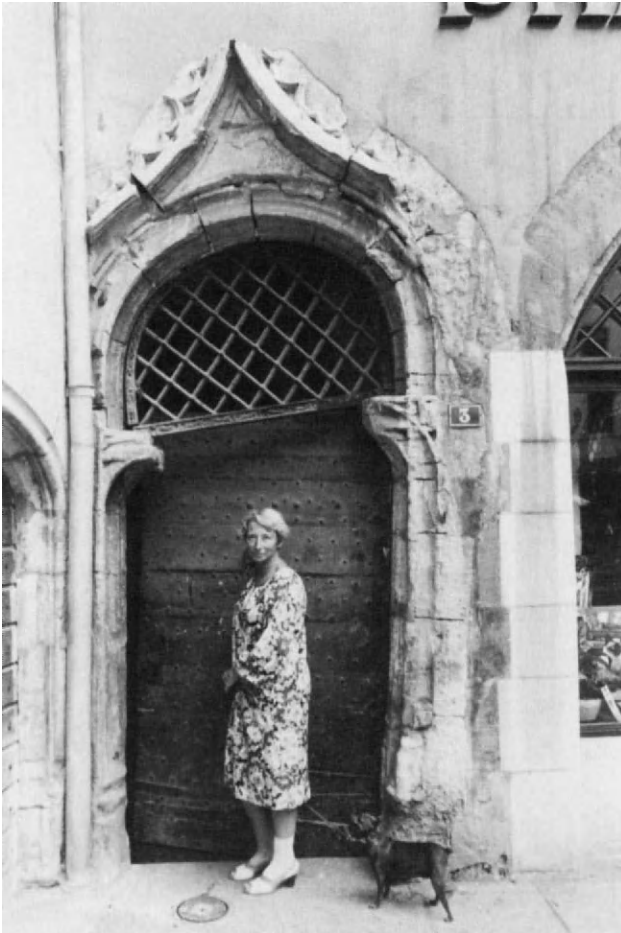
Fig. 3.38. Different settlement below a 16th century old building in Lyons, France.
