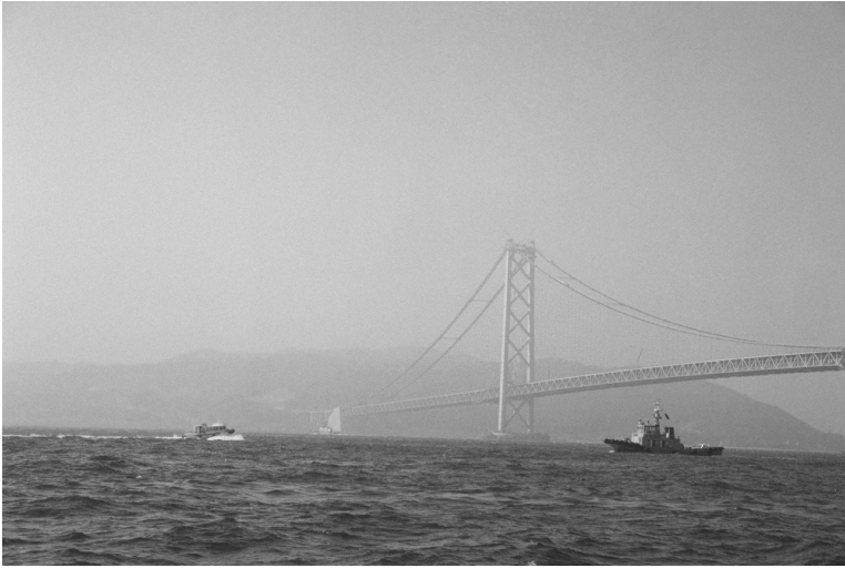
Figure 12.1 Akashi-Kaikyo Bridge, Japan.
