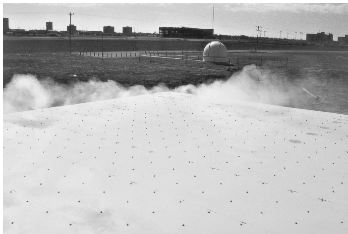
Figure 8.8 Corner vortices generated by quartering winds. (From the Texas Tech Field Experiment.)
