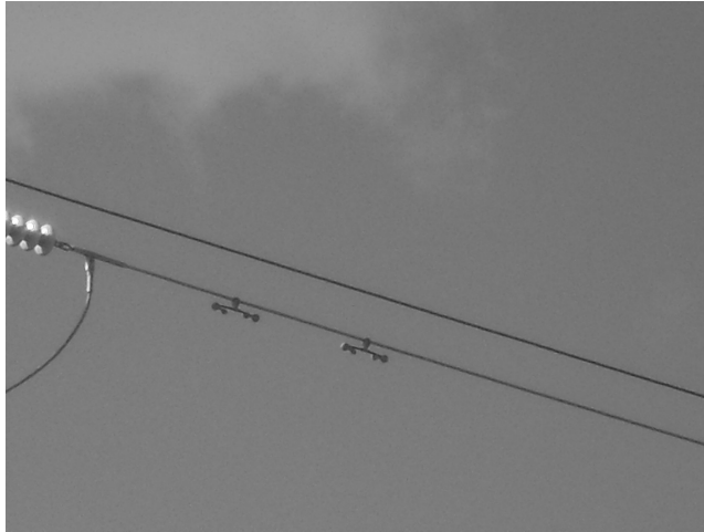
Figure 13.8 A pair of 'dogbone' dampers.
