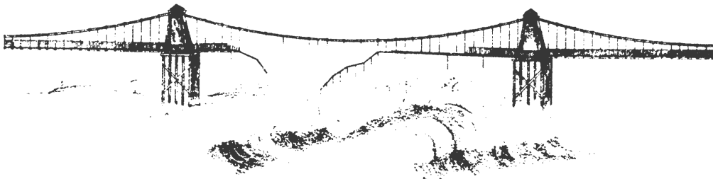
Figure 1.10 Failure of the Brighton Chain Pier, 1836.
