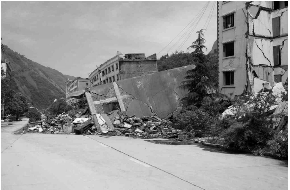
Fig. 9.28. Buildings damaged due to strong shaking
