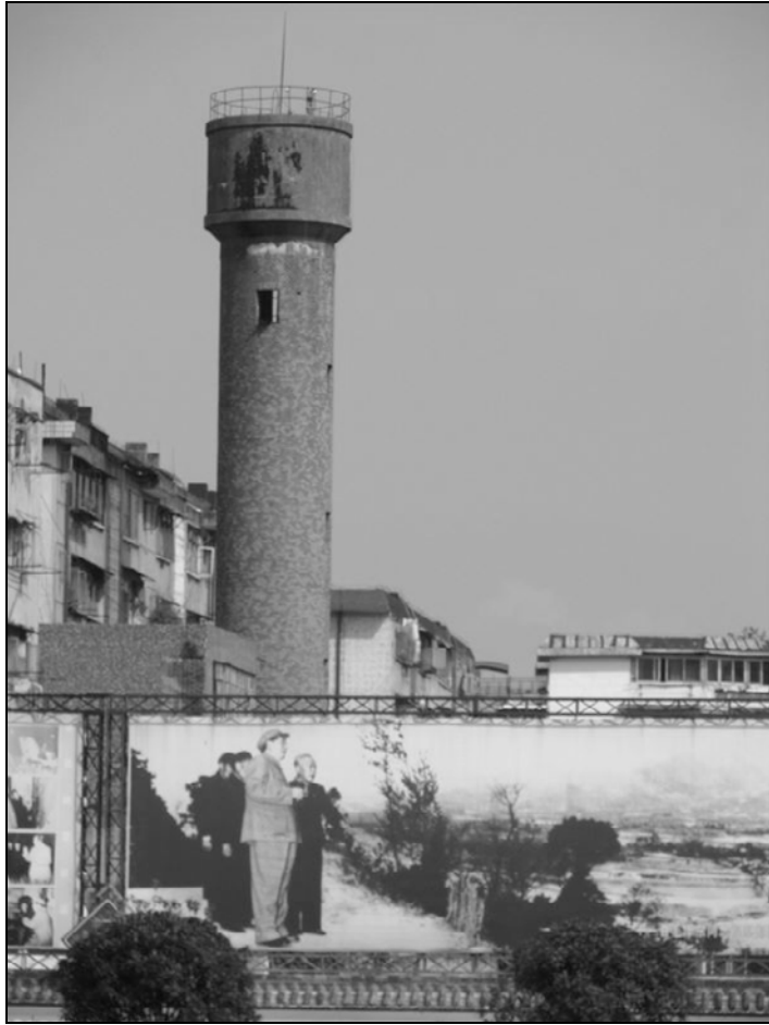
Fig. 5.13. Water tower in Dujiangyan, no apparent damage from exterior view
