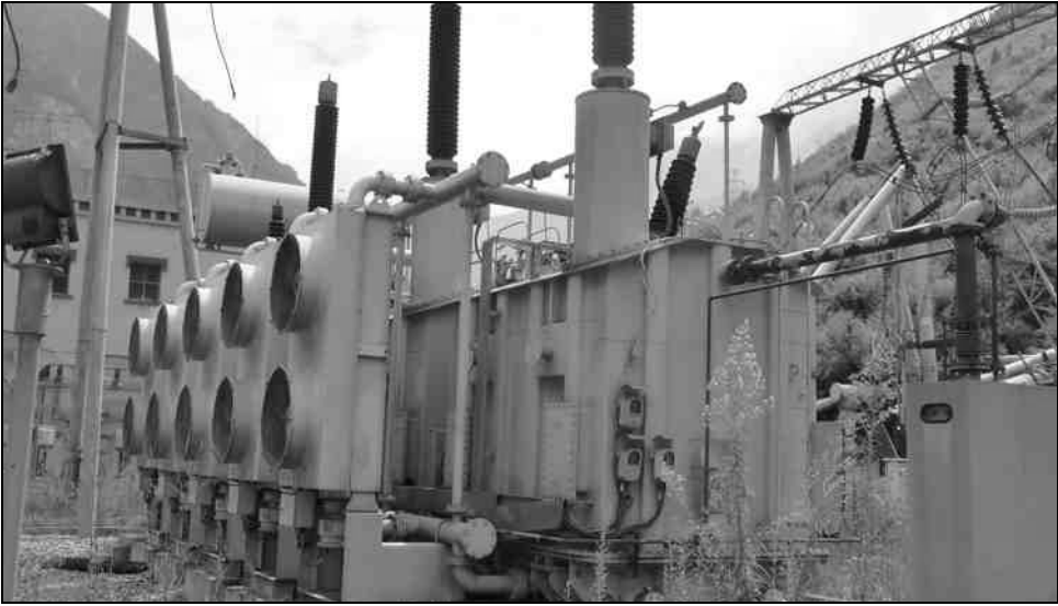
Fig. 4.45. 220/110kV transformer
