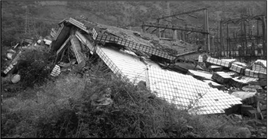
Fig. 4.18. Collapse of caretaker's two story URM residence
