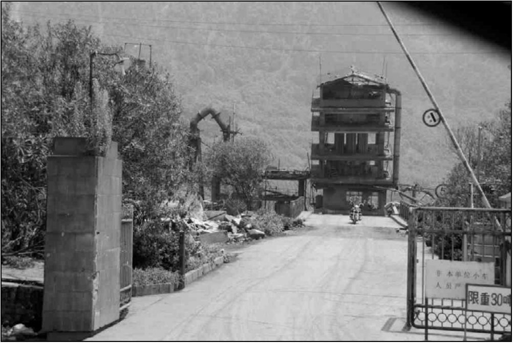
Fig. 9.78. The building of this chemical plant was leaning towards the front door of the plant. Note the debris inside the entrance.
