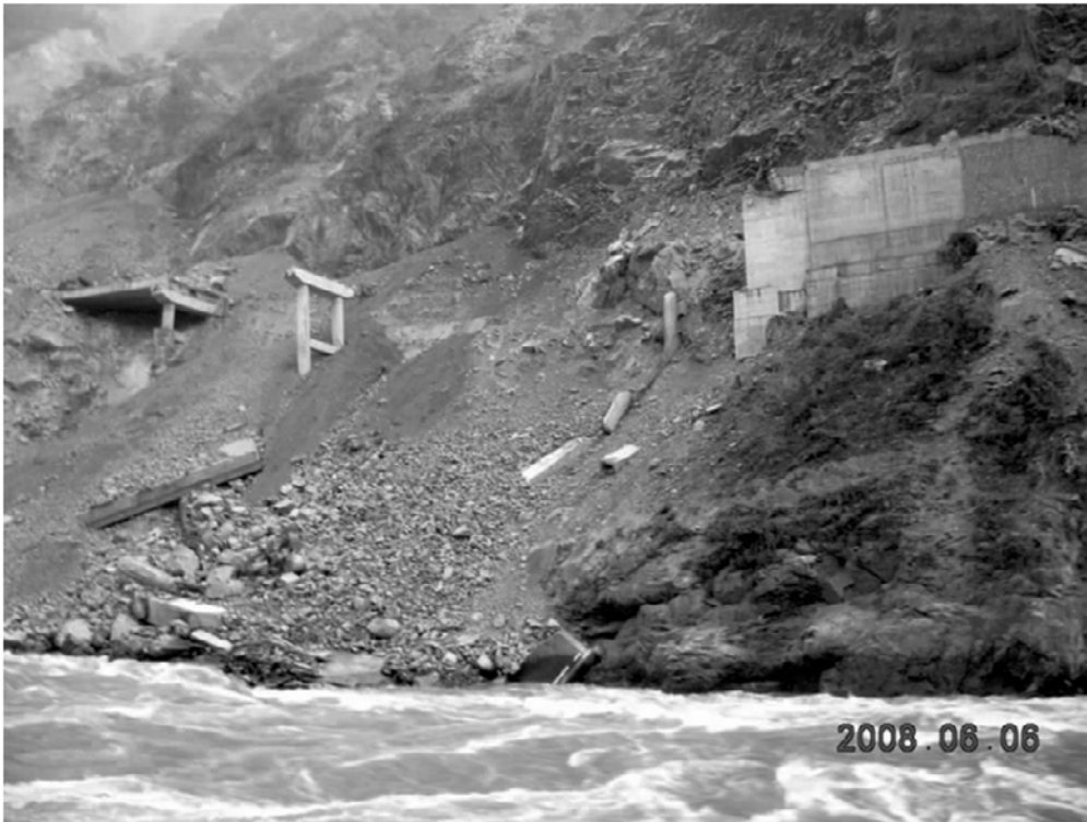
Fig. 3.6. Landslide destroyed a bridge on Duwen Road
