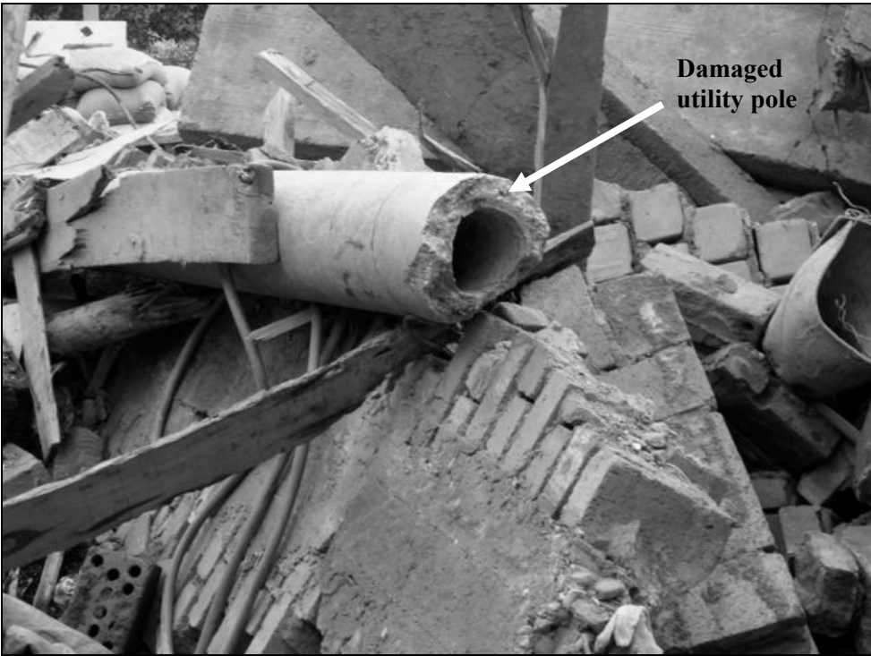
Fig. 6.48. Utility pole damaged by collapsing building
