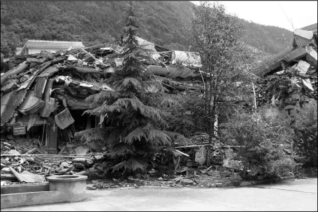
Fig. 9.29. This building pancaked with four floors collapsing to the second floor.
