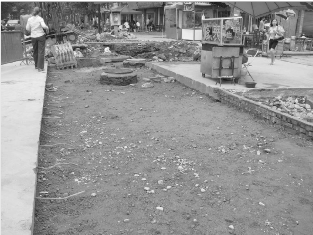
Fig. 5.3. Repair to water and sewer pipes in Dujiangyan
