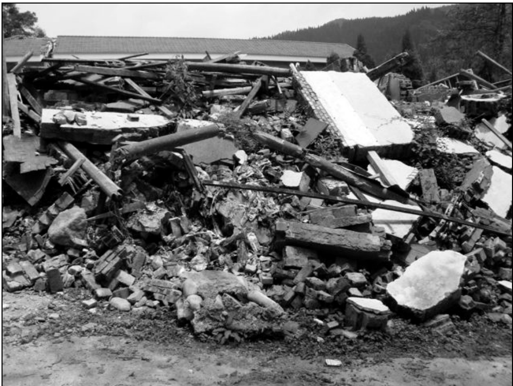
Fig. 9.35. Houses reduced to rubble close to Hongkou town. There were many casualties in this area.
