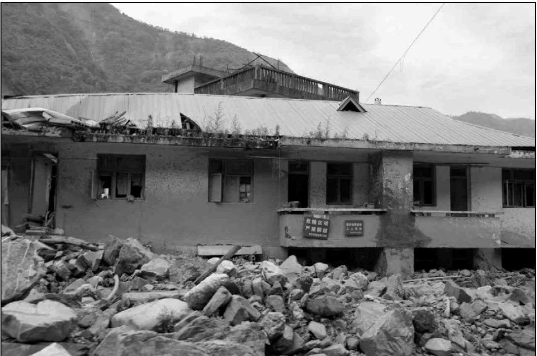
Fig. 9.24. The debris flow carried rocks that did the most damage.
