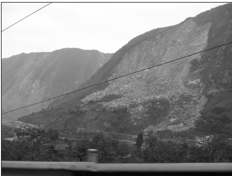
Fig. 10.1. Large landslide blocking road
