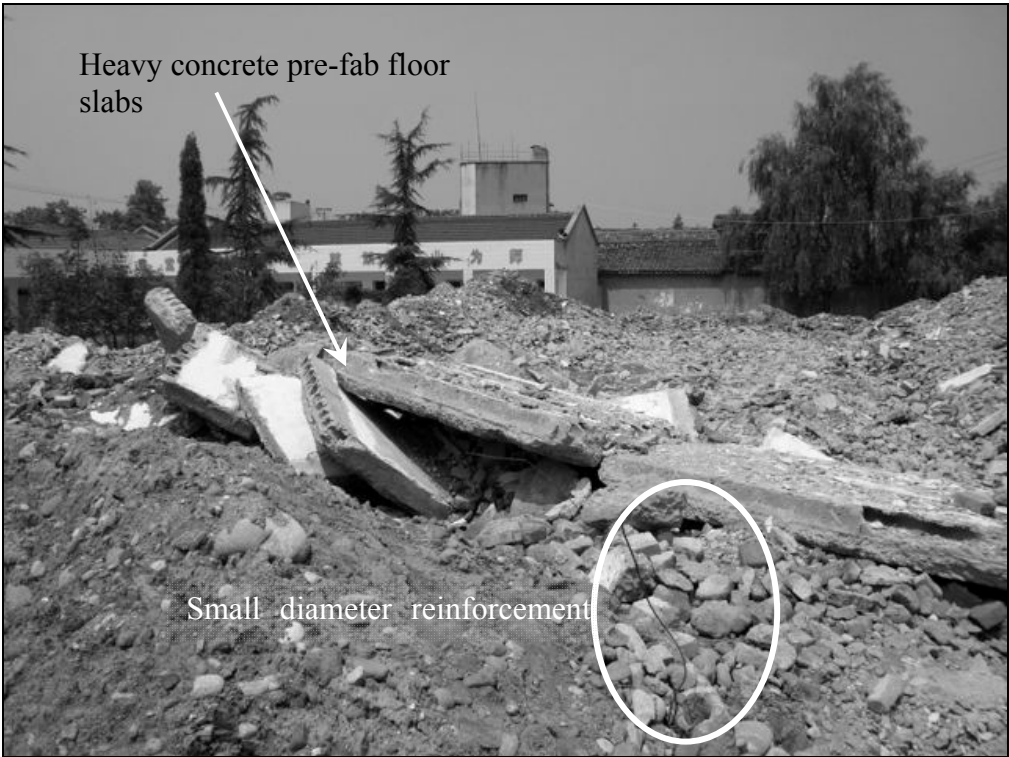
Fig. 9.8. This figure shows the concrete floor slab used. Note the small size reinforcement bar.
