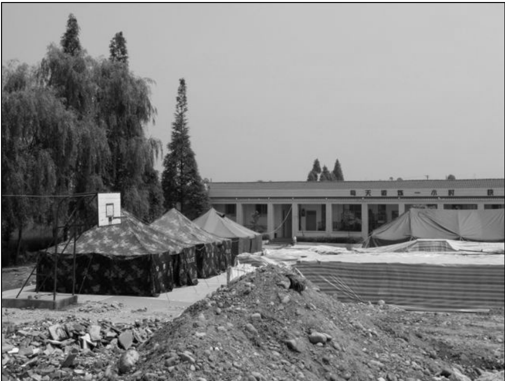
Fig. 9.9. Tents were erected in the school basketball field to store undamaged desks, chairs, and other materials used in classrooms.
