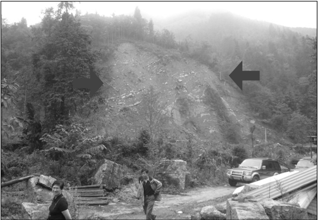
Fig. 5.5. Broken water pipes at either side of a landslide, Shenxigou Village (near Hongkou); landslides cause more damage than earthquakes.
