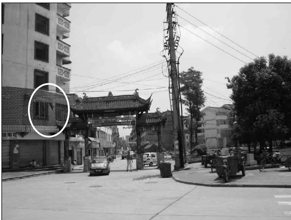
Fig. 9.60. Undamaged gate in Dujiangyan. There were minor cracks on the exterior wall of the building on the left.
