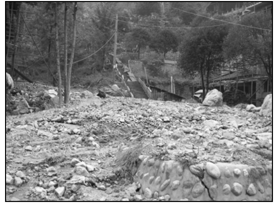
Fig. 10.9. Mud/debris flow blocking road
