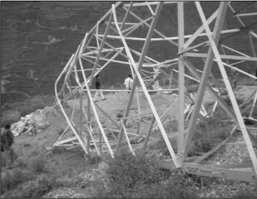
Fig. 4.68. Collapsed Tower, #13, Jiangsang line
