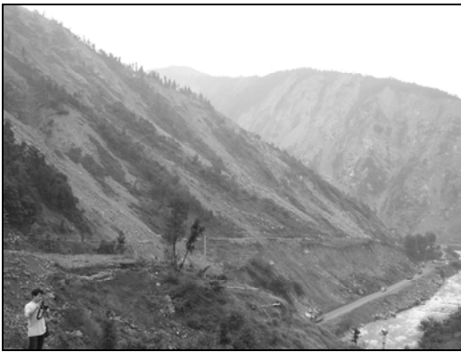
Fig. 10.4. Relocated road below blocked road
