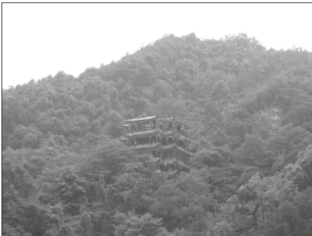
Fig. 9.59. This Li Bing Temple had significant damage but did not collapse.
