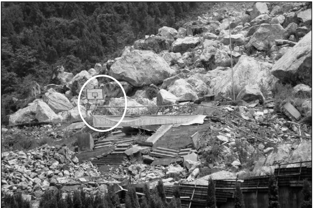
Fig. 9.15. The remains of this a school in Beichuan town are under the rocks. Note the basketball goal on the left hand side.
