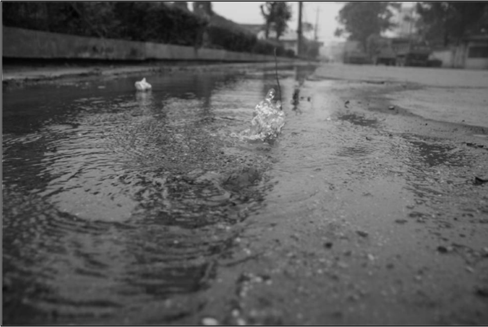
Fig. 5.2. Water leak under road
