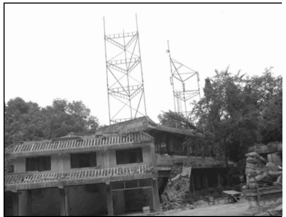
Fig. 6.23. A damaged cell site in Dujiangyan (Courtesy of IEM)
