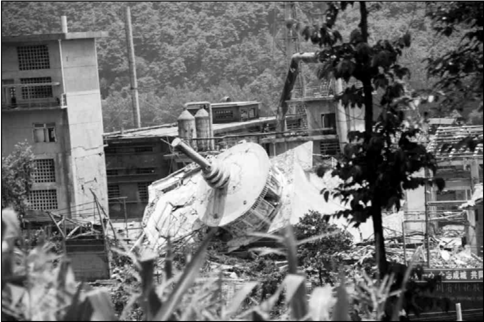
Fig. 9.76. Damage at another building of the fertilizer plant shown in Fig. 9.76.
