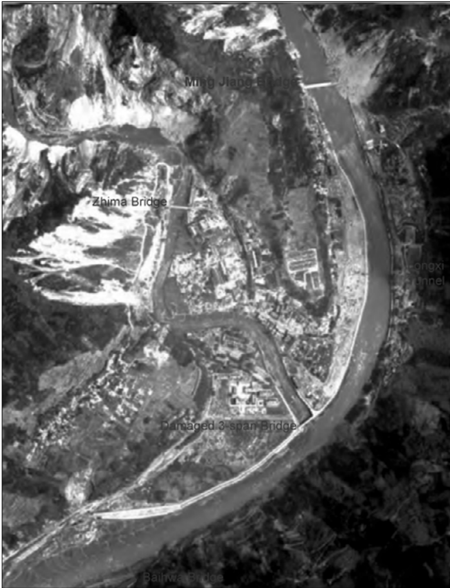
Fig. 3.36. Aerial view of structural damage in Yingxiu Village (Deren Li, 2009)
