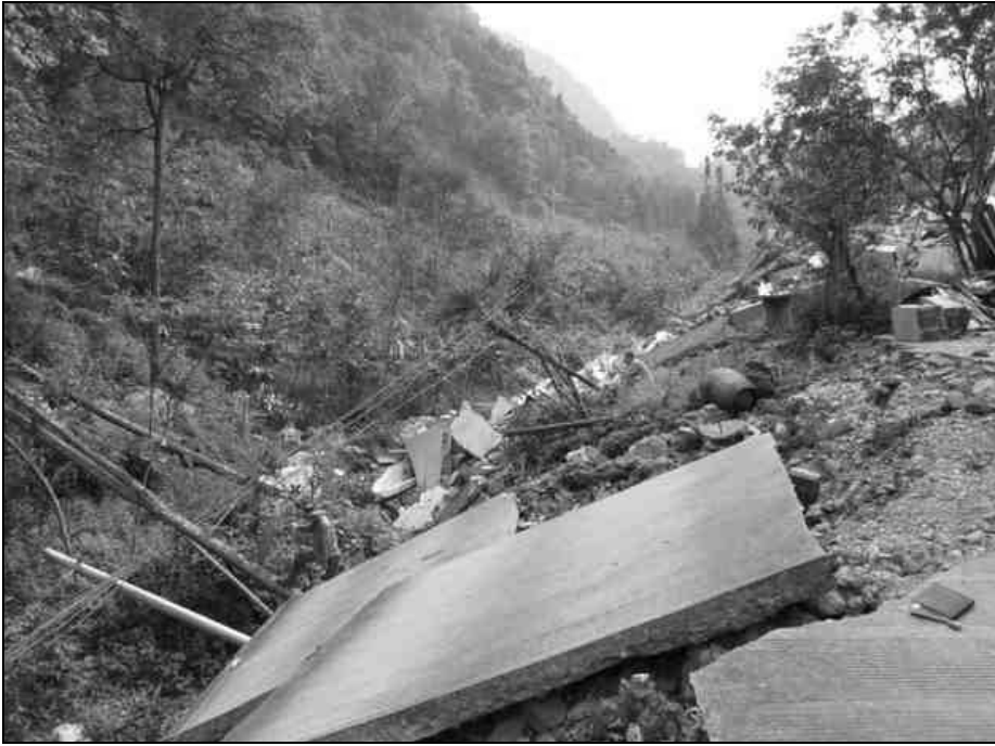
Fig. 4.73. Surface faulting uplift of about 3 m and lateral shift of about 4 m with damaged road and tilted distribution poles
