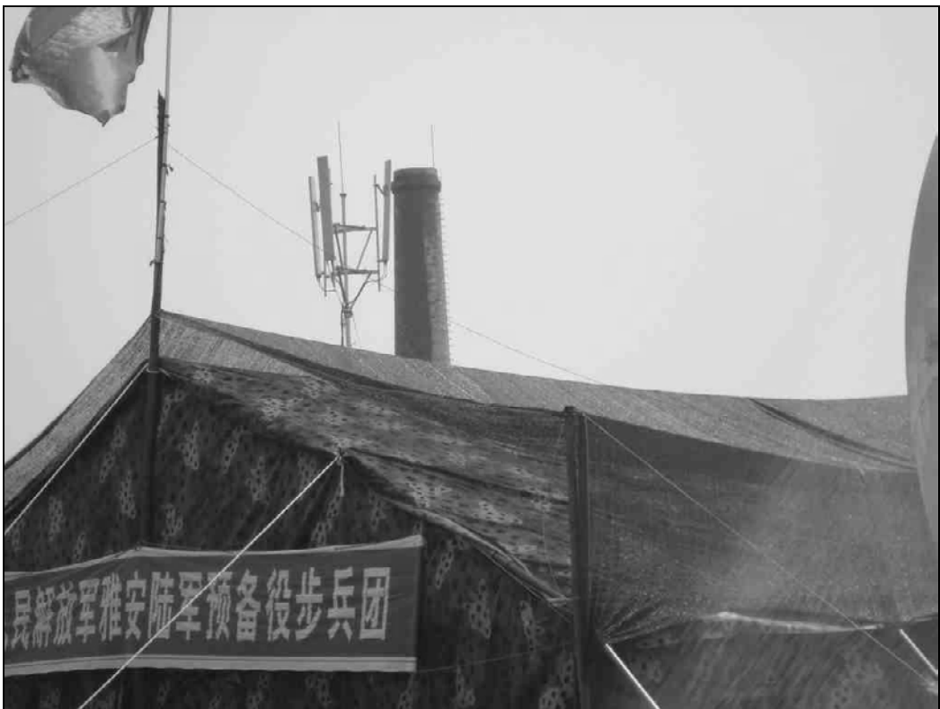
Fig. 6.20. A temporary cell site set up on the military campground
