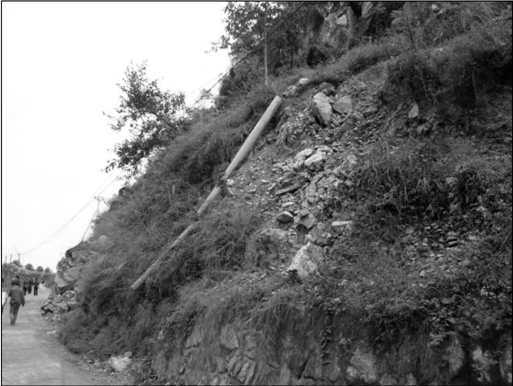
Fig. 6.55 A pole collapsed along the slope and broke into four pieces.
