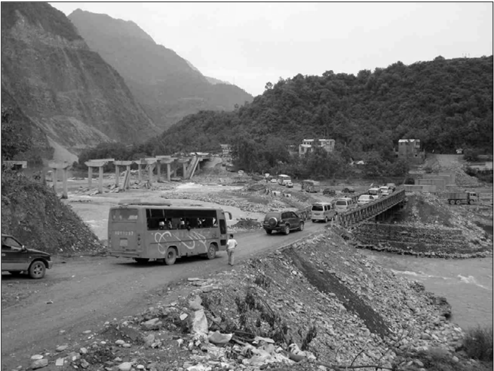
Fig. 3.59. The temporary bridge was wide enough for single-lane traffic
