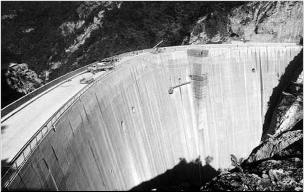
Fig. 8.8. Shapai Dam (Courtesy of IEM)
