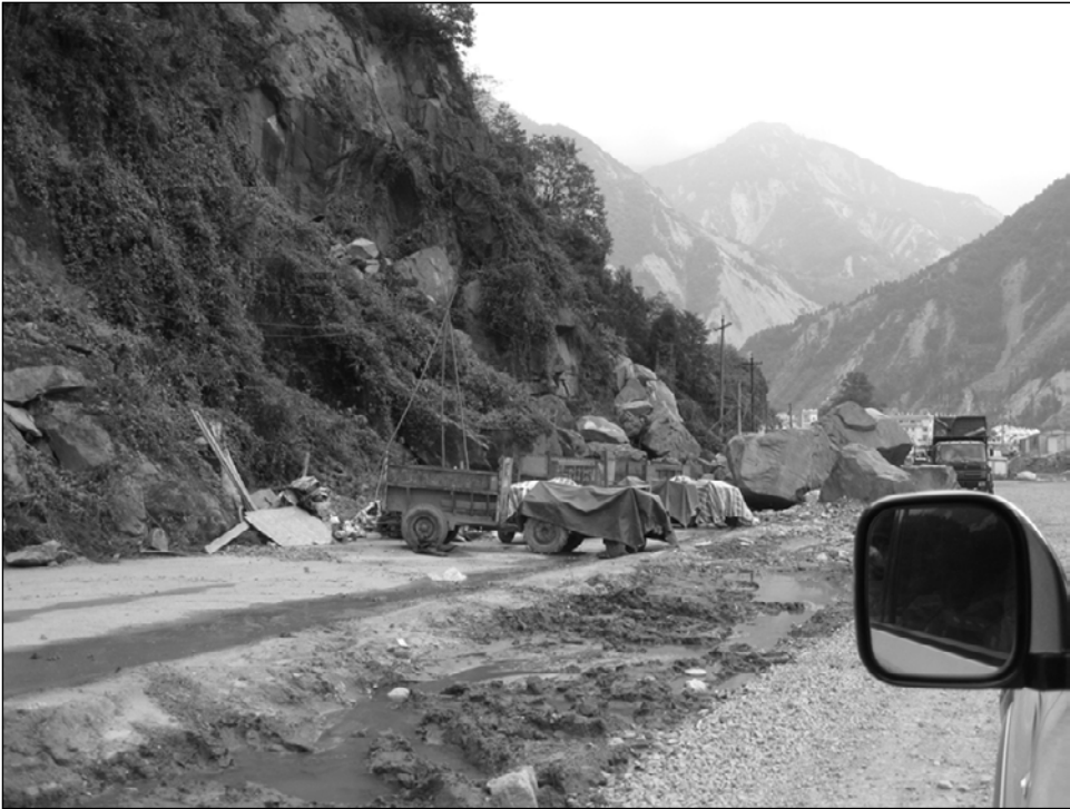
Fig. 3.15. Fallen rocks on Route 213 after the May 12 earthquake
