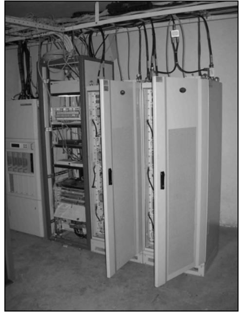
Fig. 6.12. Radio, controller, and transport equipment look quite new
