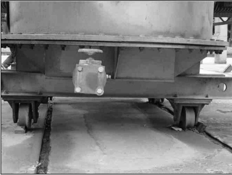
Fig. 4.10. Wheel-mounted transformer
