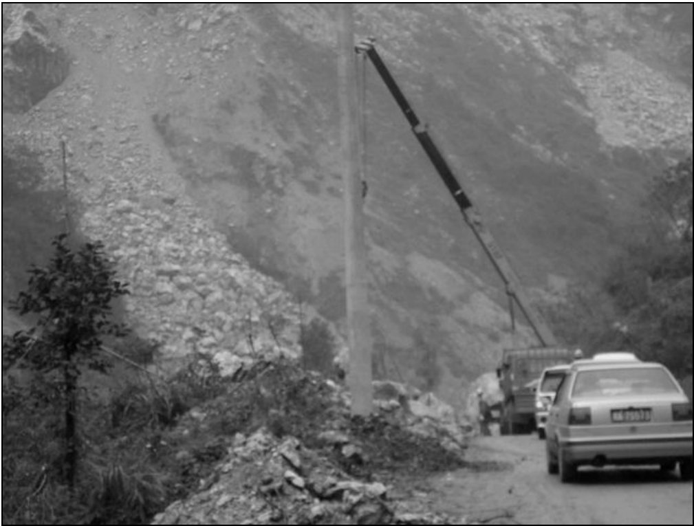
Fig. 6.46. The repair crew installing poles to replace temporary cable
