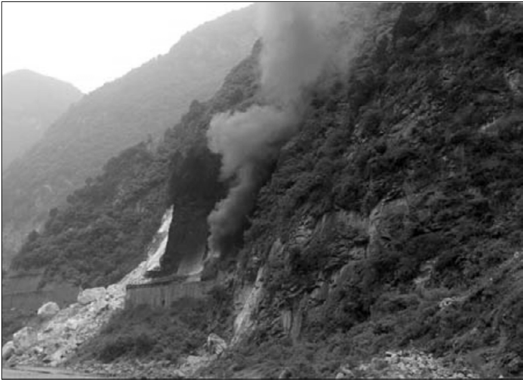
Fig. 3.89. Gasoline tanker train derailed in a tunnel in Xuixian County in Gansu Province and caught fire (Courtesy of Prof. Mei and Dr. Zhang)
