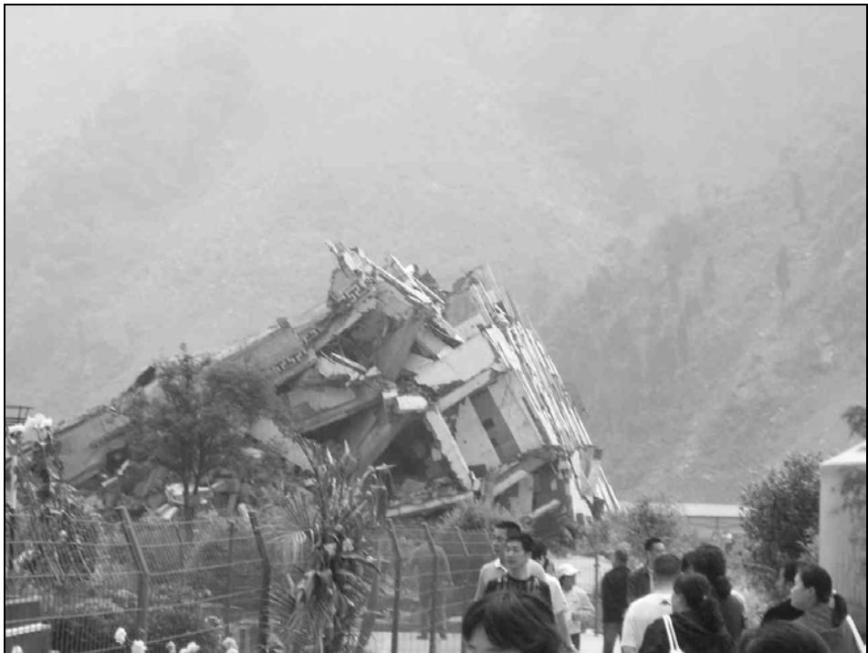
Fig. 9.2. Totally collapsed building Yingxiu, Xuan Kou High School.
