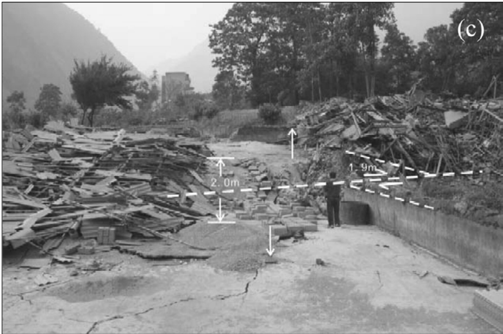
Fig. 3.18. Surface fault damaged a road between Beichuan and Nanba
