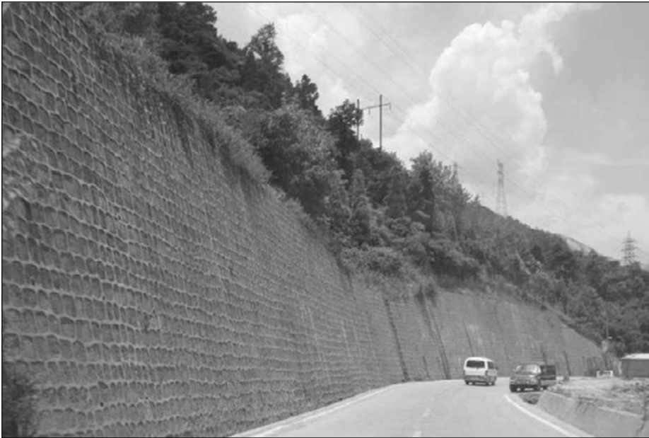
Fig. 3.20. Same type of retaining wall as Fig.3.19 but without damage
