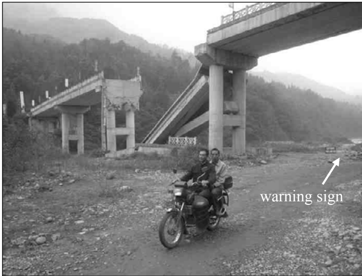
Fig. 3.47. Gaoyuan four-span bridge (Hongkou)
