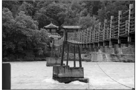
Fig. 3.67. Flexible bridge in the flood management facility
