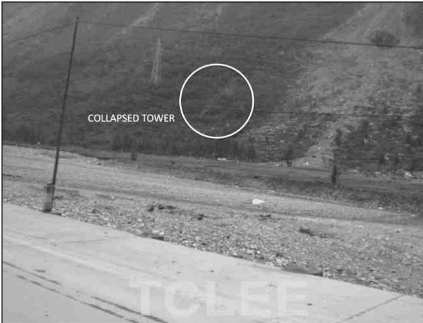
Fig. 4.62. Collapsed 110 kV tower
