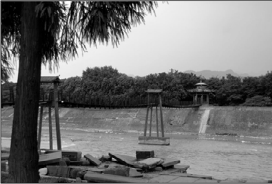
Fig. 3.66. Flexible bridge in the flood management facility
