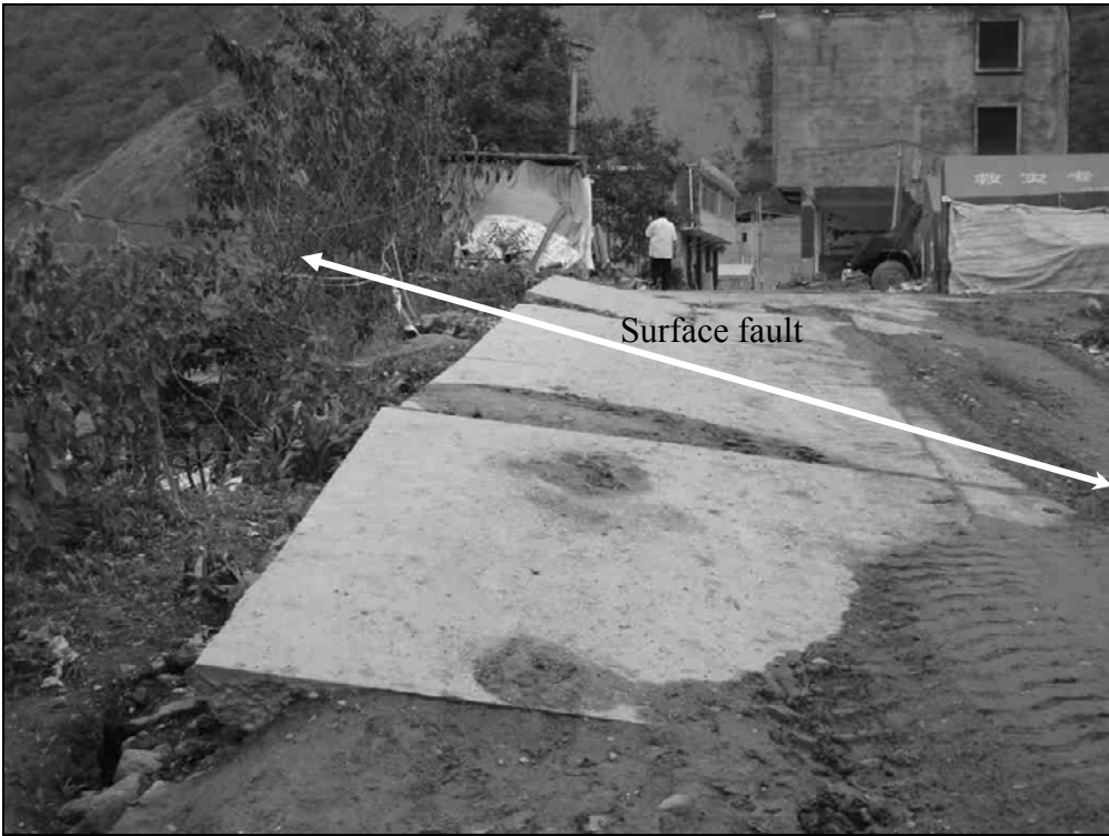
Fig. 9.88. In Hejiaba the surface fault crossed this road in the village. The buildings within 200 m of this surface faulting were damaged and many collapsed.
