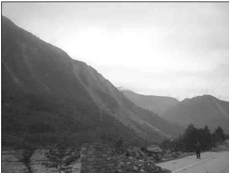
Fig. 4.61. Reconstructed 220 kV tower
