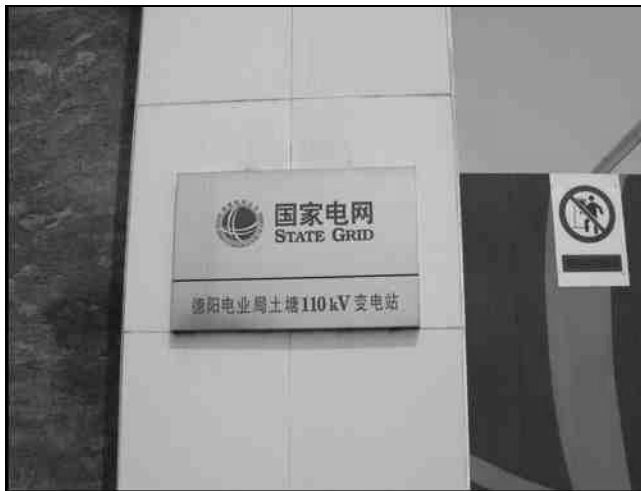
Fig. 4.8. 110 kV substation located between Deyang and Shifang
