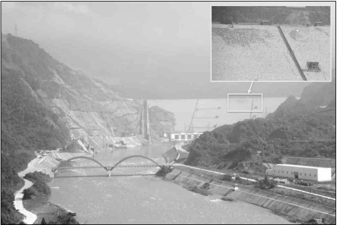
Fig. 8.3. Zipingpu Dam; insert shows surface cracking on the down stream dam face.
