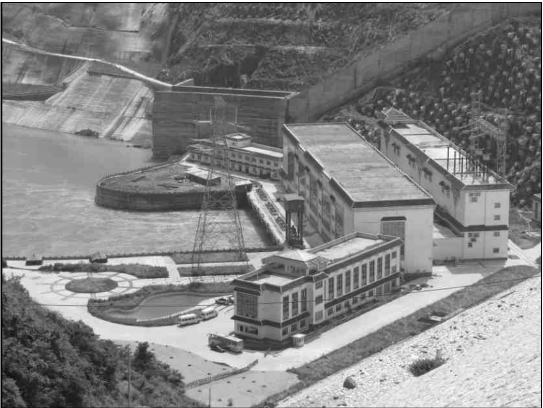
Fig. 4.5. Hydroelectric power plant buildings (Zipingpu Dam) (Courtesy of IEM)
