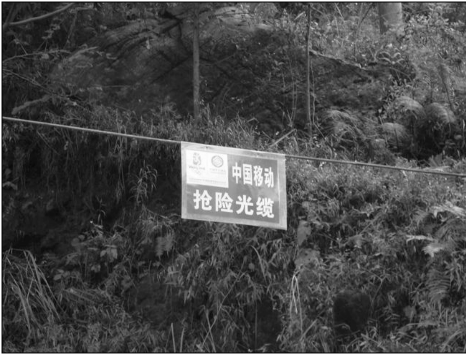
Fig. 6.37. Sign showing a China Mobile emergency response optical fiber cable along the side of the road leading to Yingxiu.
