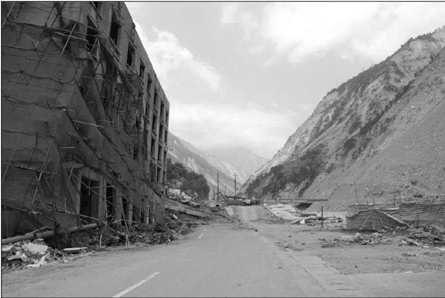
Fig. 3.14. Colocation damage due to collapses buildings blocking roads in Yingxiu
