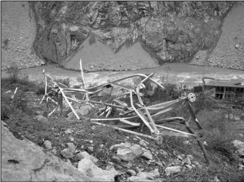
Fig. 4.55. Collapsed tower
