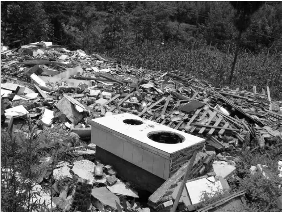
Fig. 2.29 This house was about 30 m from the surface fault show in Fig. 2.28. The stove at the back of the house was the only recognizable appliance.
