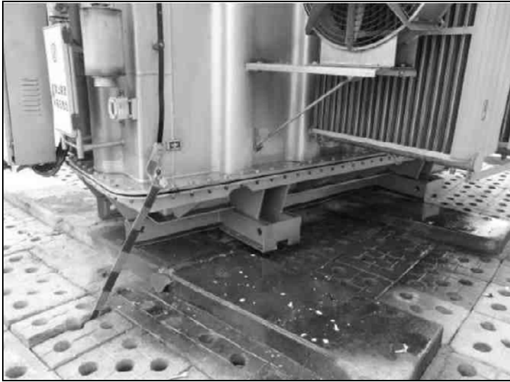
Fig. 4.11. Skid-mounted transformer
