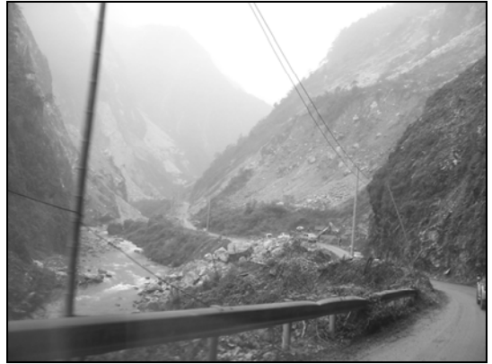
Fig. 10.7. One-way traffic and road clearing
