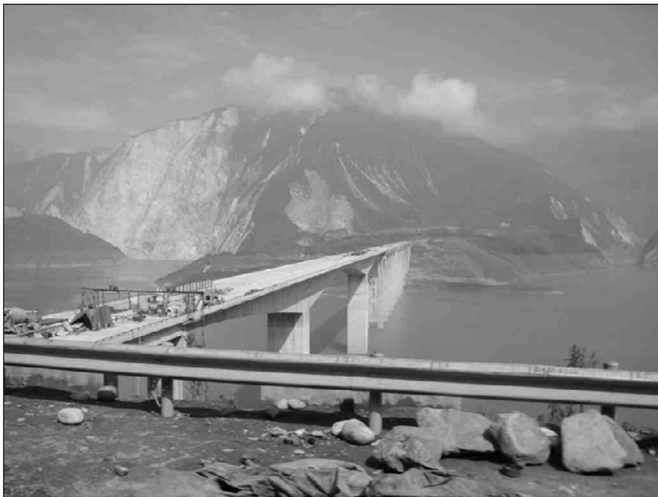
Fig. 3.32. Miaoziping Bridge, heavy equipment on the bridge making repairs
