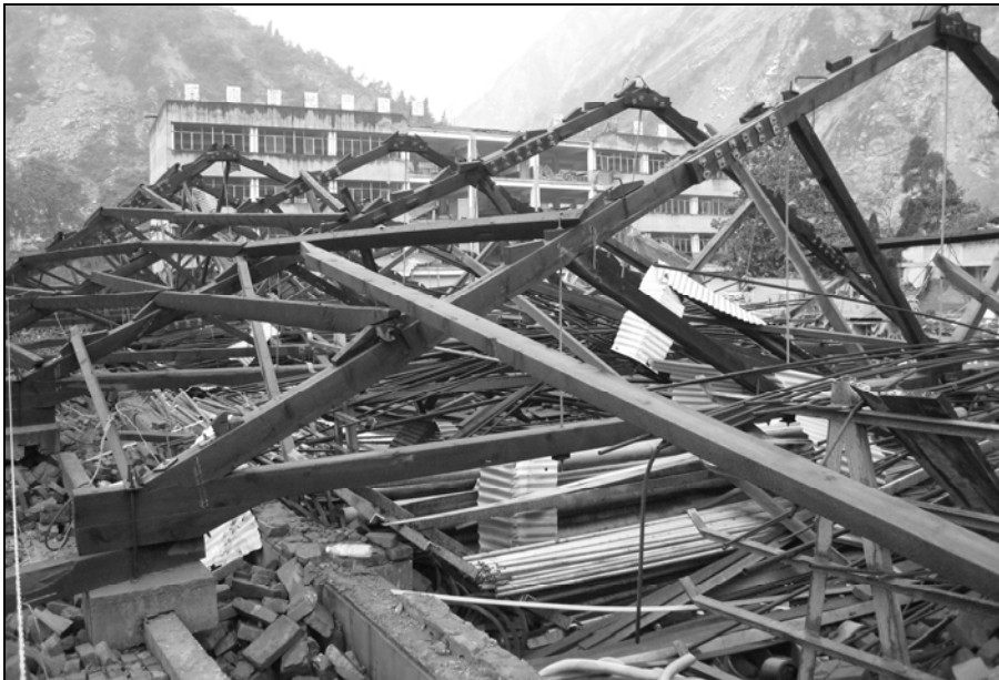
Fig. 5.16. Storage building (Yingxiu)
