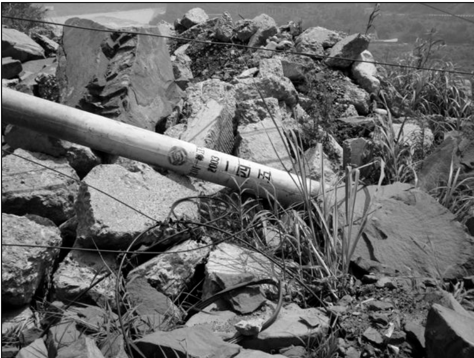
Fig. 6.36. Damaged pole due to rock falls
