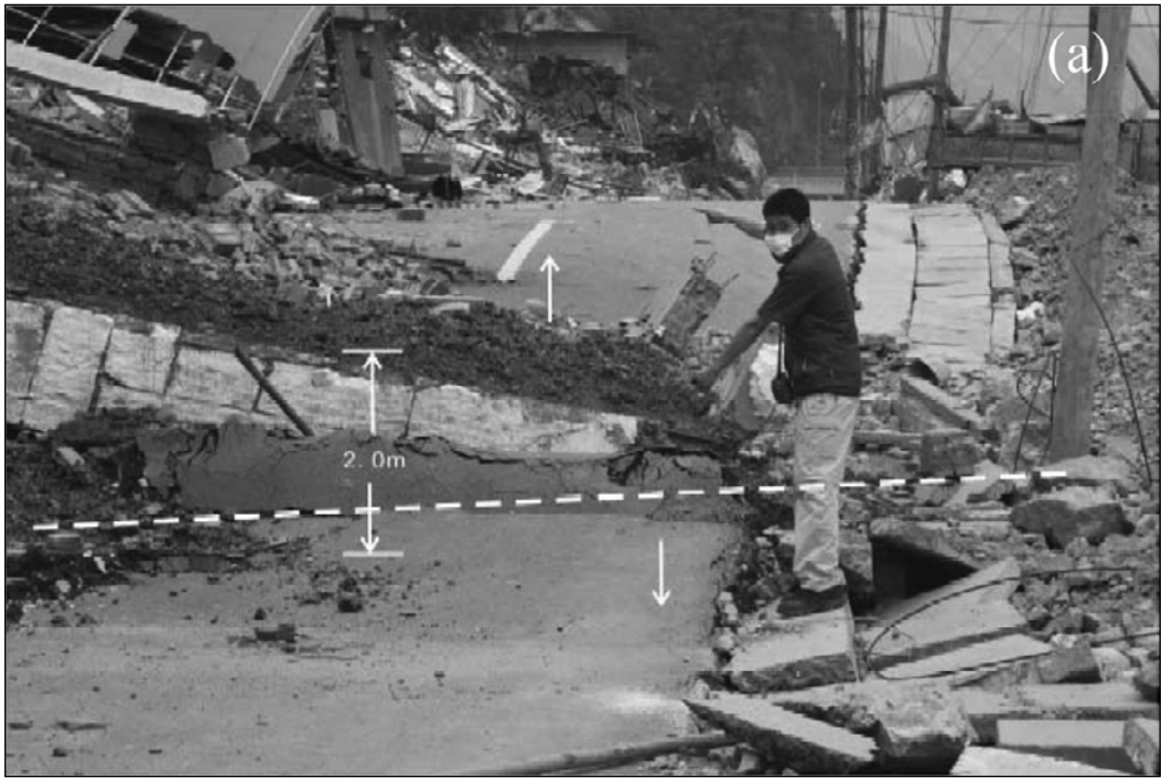
Fig. 3.9a Yingxiu Town near the southern end, with a vertical offset of about 2 m and right-lateral offset of about 0.5 m
