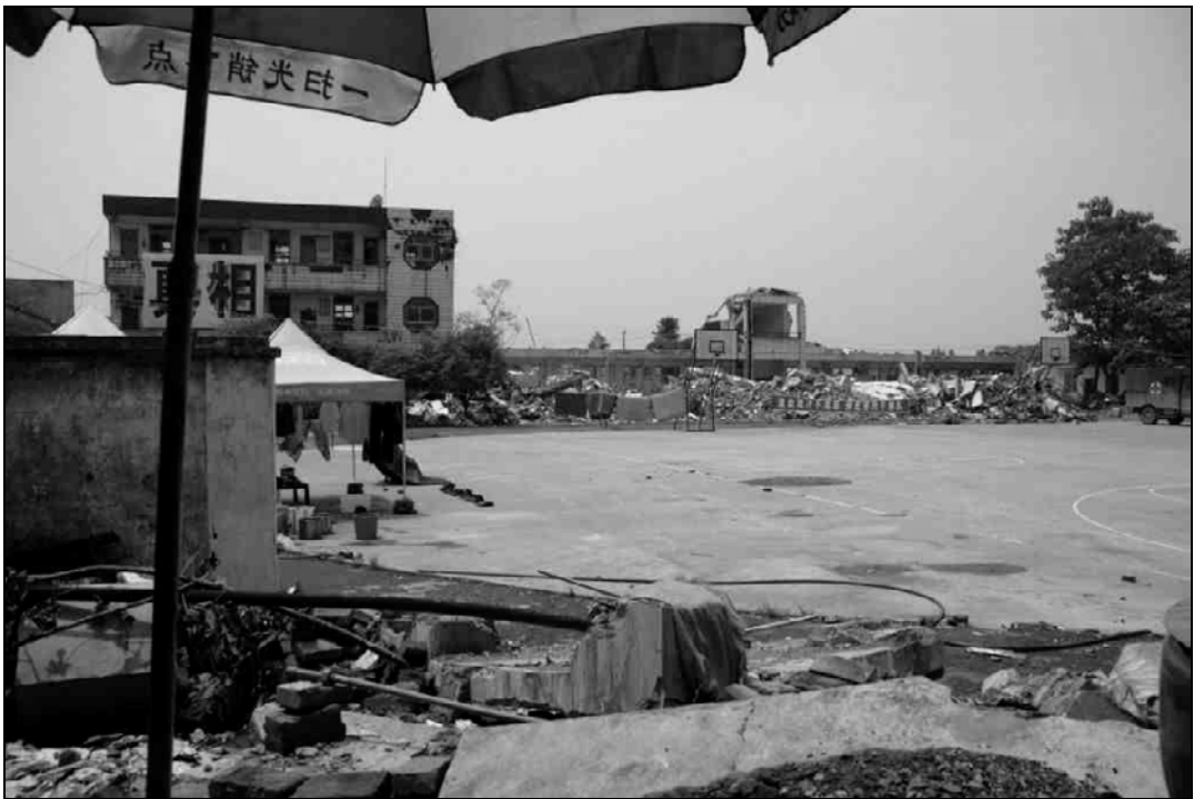
Fig. 9.12. The collapsed three-story classroom building.
