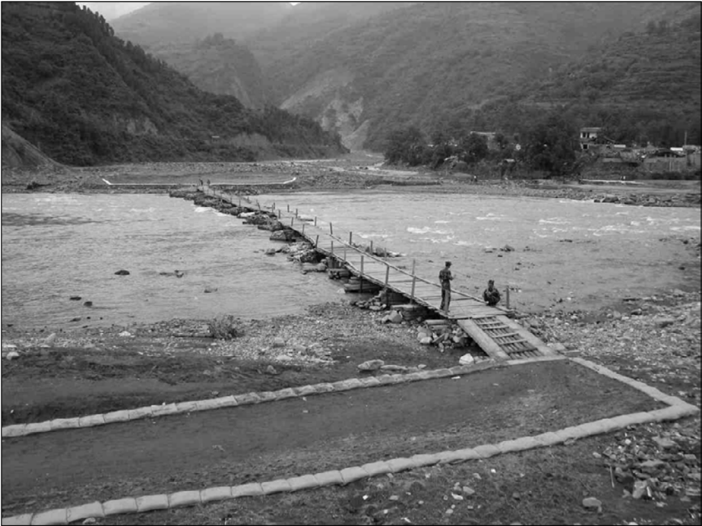
Fig. 3.62. A temporary wooden bridge was built for villagers to cross from Hejiaba to Nanba. Four PLA soldiers were posted on either end of the bridge to guard against vehicle crossing.
