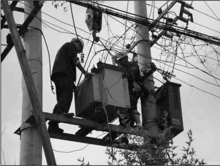
Fig. 4.75. Distribution system transformer (10 kV) being replaced (Hongkou), July 16 2008
