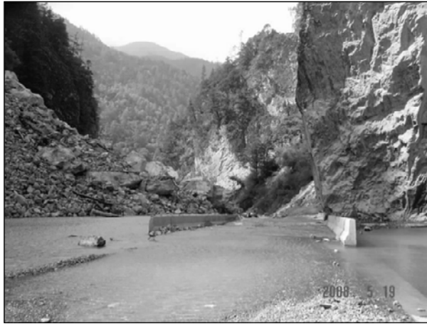
Fig. 3.12. Quake lake closed roads and damaged bridges
