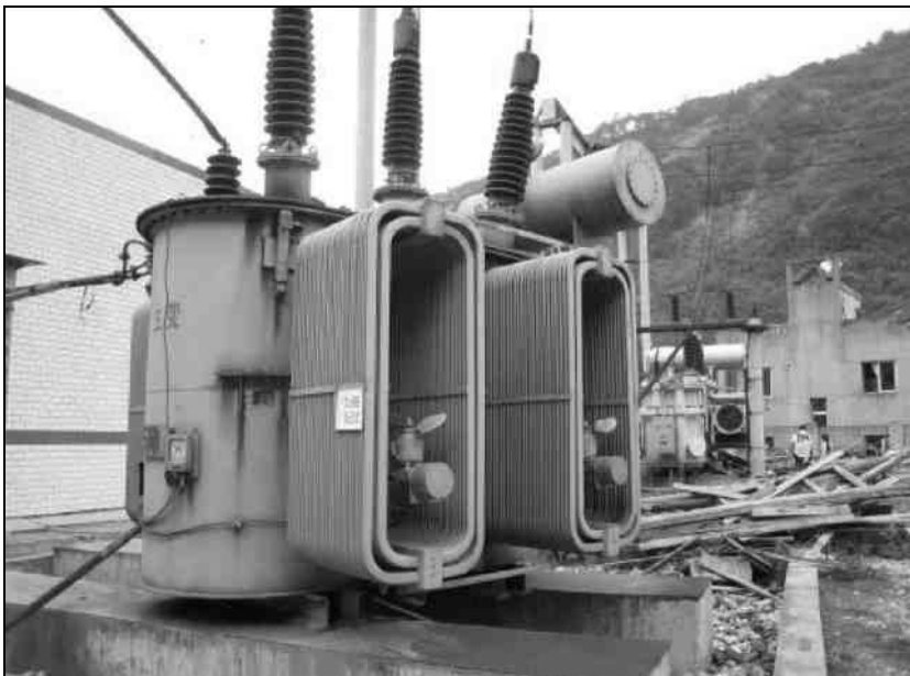
Fig. 4.12. Skid-mounted transformer
