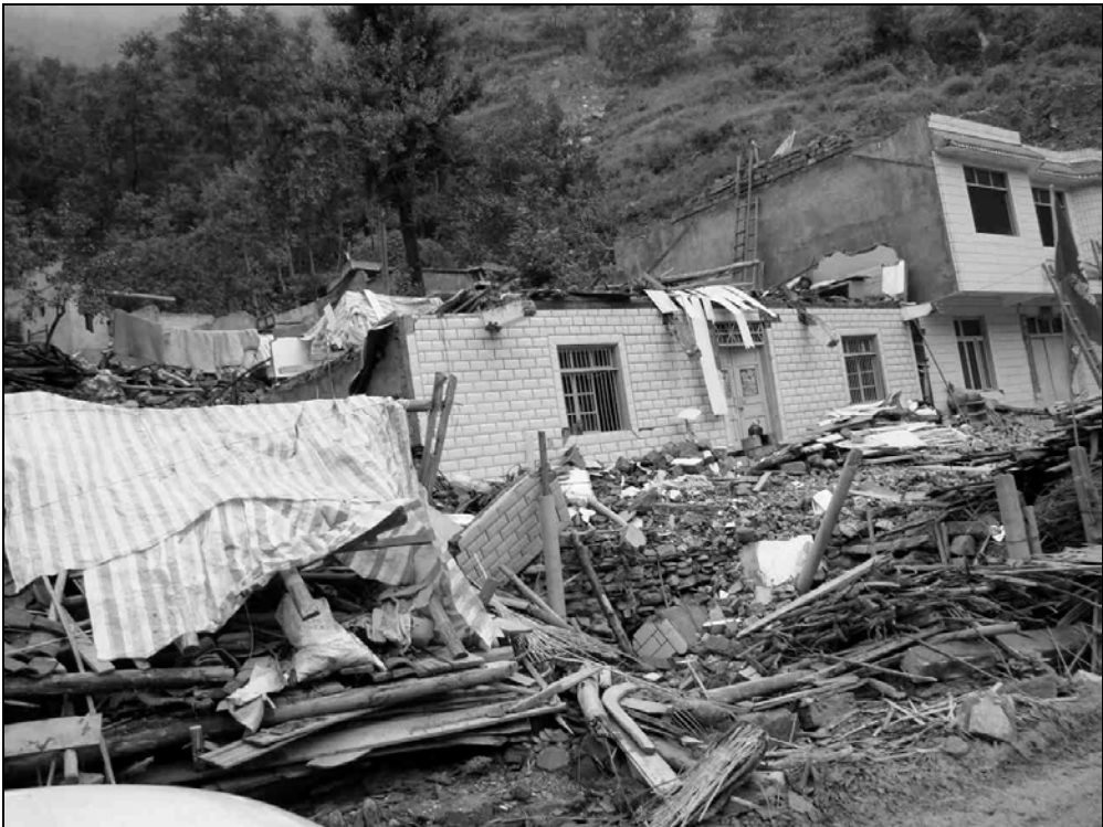
Fig. 9.83. This was a common scene in Nanba. Note the concrete building on the right performed quite well.
