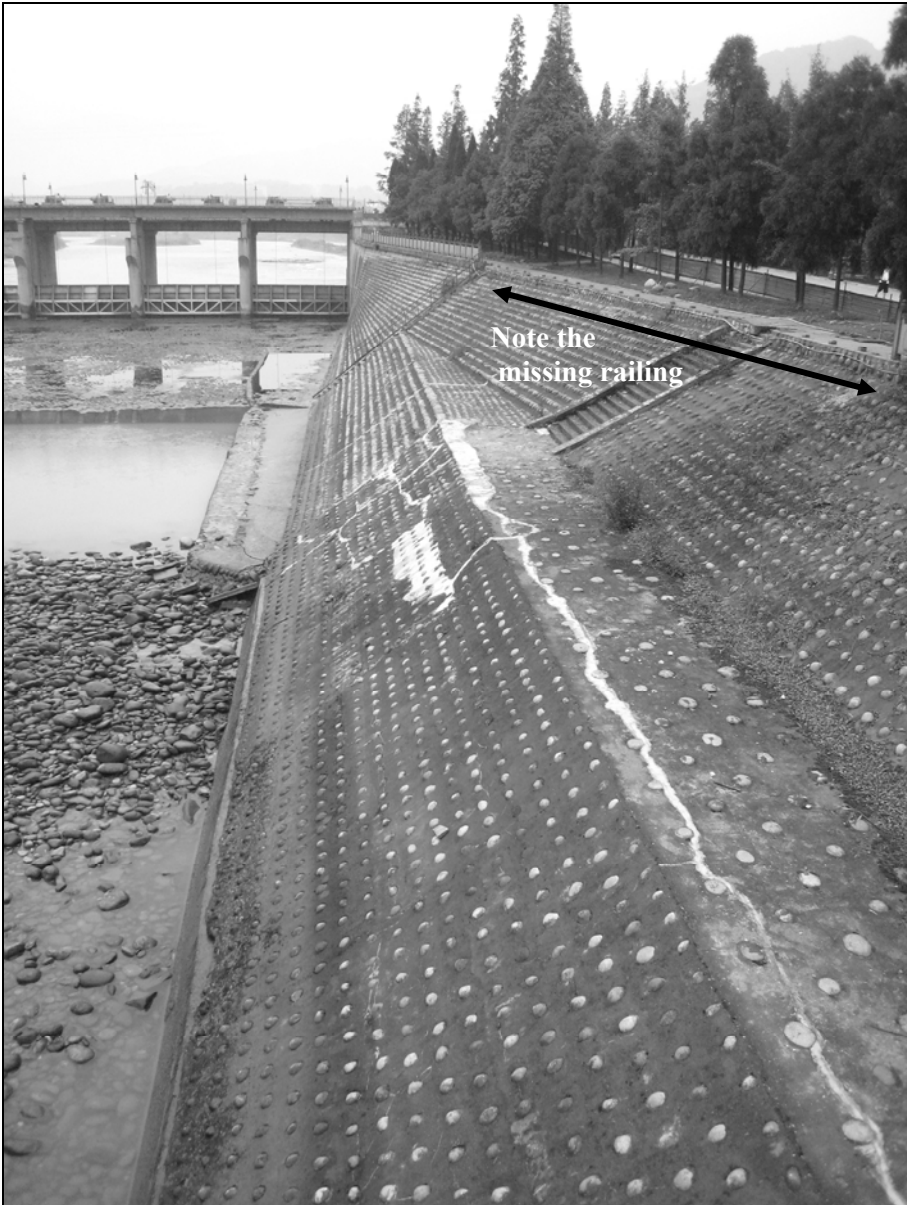
Fig. 5.23. Repairs made to downstream slope protection
