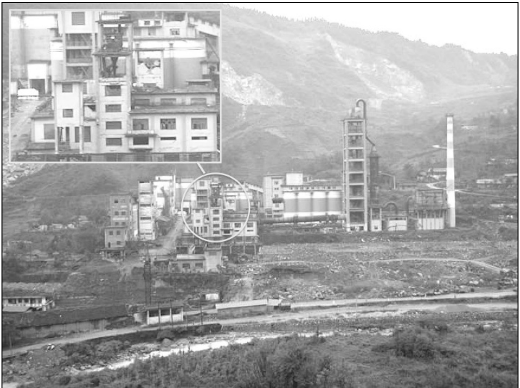
Fig. 9.67. A cement manufacturing facility close to Yingxiu showed very little damage. It was not operating during the team's visit due to road damage.
