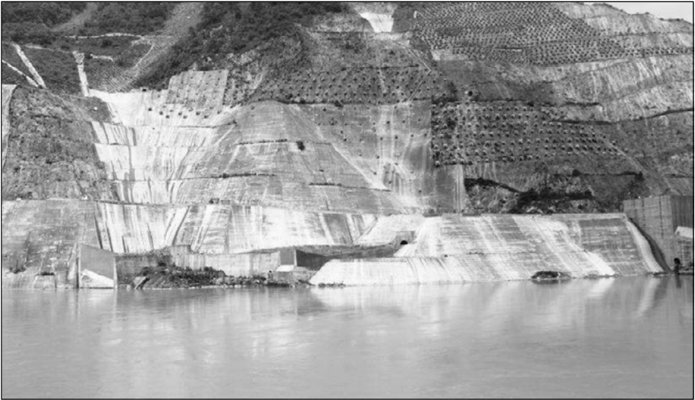
Fig. 3.22. Rock bolts did a good job of securing Zipingpu Dam abutments
