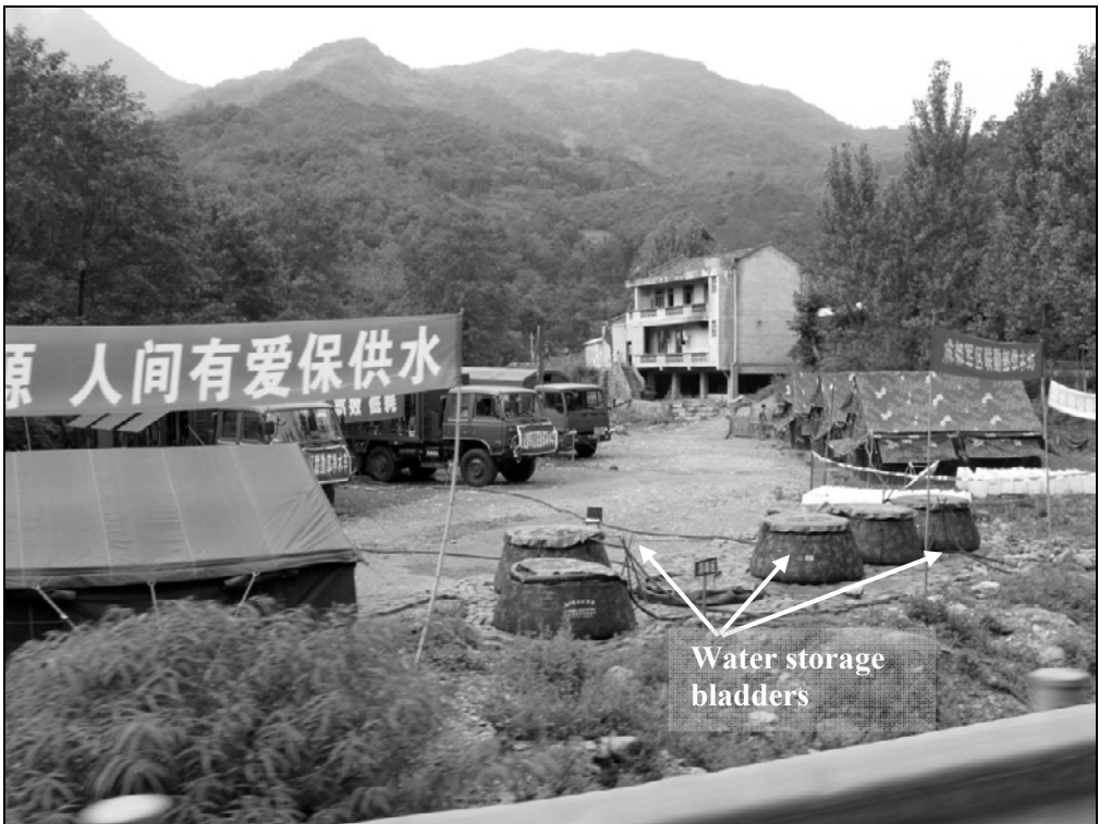
Fig. 5.19. Bladders set up by the People Liberation Army to provide water to local communities
