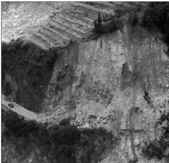
Fig. 3.17. Landslide on Route 213 between Yingxiu and Wenchuan
