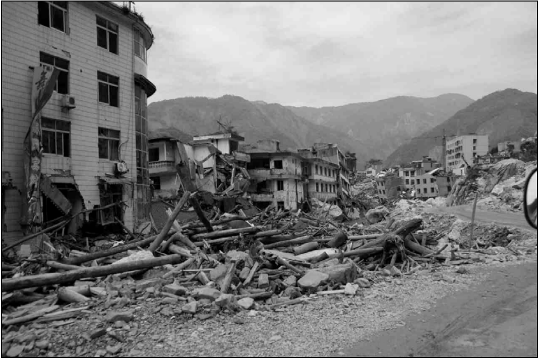
Fig. 9.25. Timber debris flowing from the mountains also caused lots of damage to buildings.
