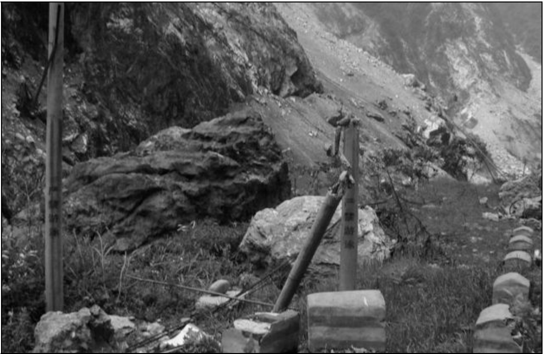
Fig. 6.41. A pole damaged by the rock fall, note that pole on the left was not damaged
