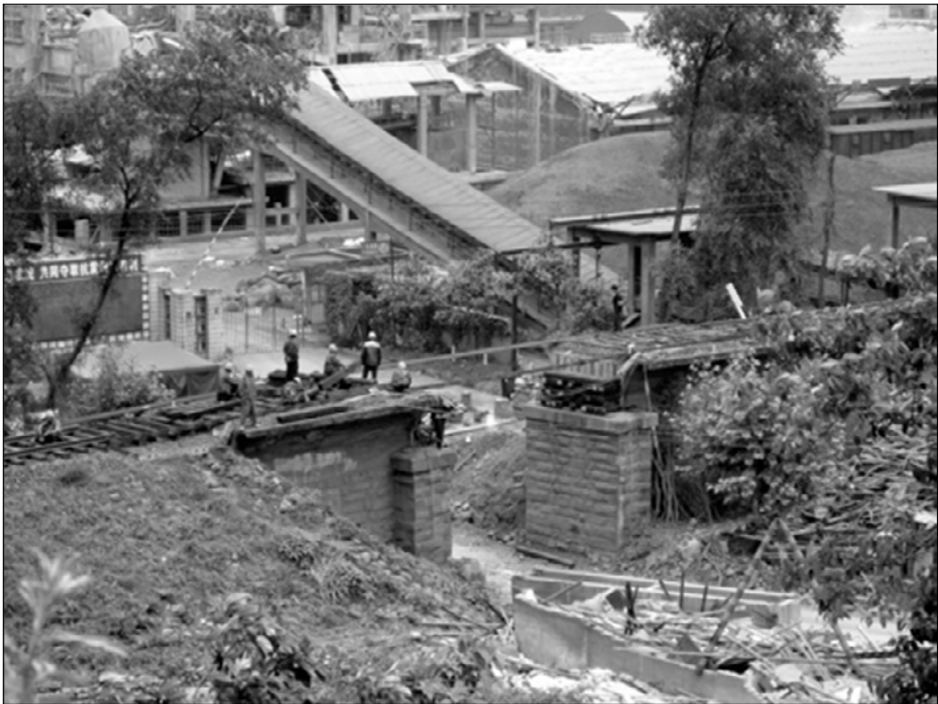
Fig. 3.87. Collapsed railroad bridge in Shifang (Courtesy of Prof. Mei and Dr. Zhang)
