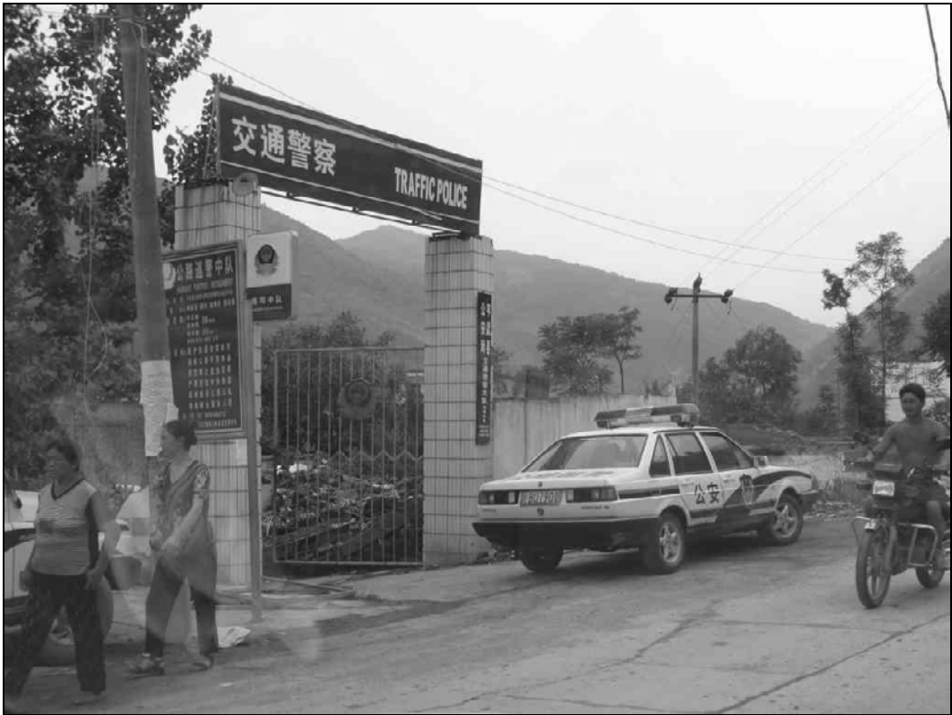
Fig. 9.86. The traffic police office building on the main road in Nanba collapsed, but the front gate remained standing
