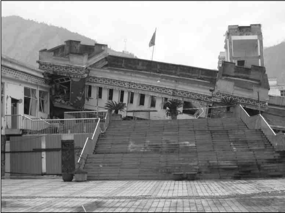
Fig. 9.1. Partially collapsed Yingxiu, Xuan Kou High School.
