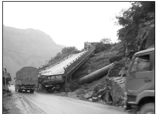
Fig. 10.5. Relocated road at downed bridge
