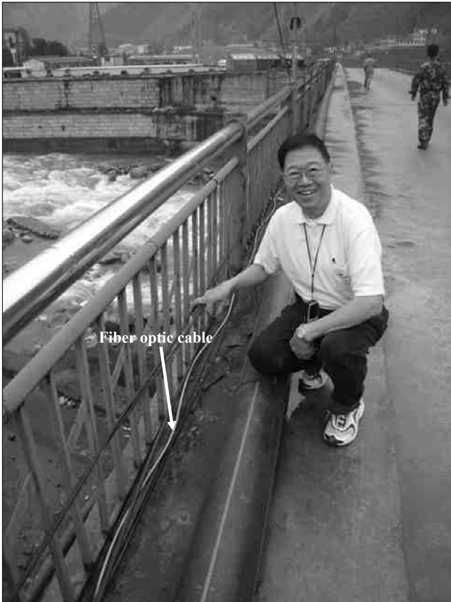
Fig. 3.41. Temporarily rerouted utilities (power, telecommunication, and water) on the three-span bridge, Yingxiu
