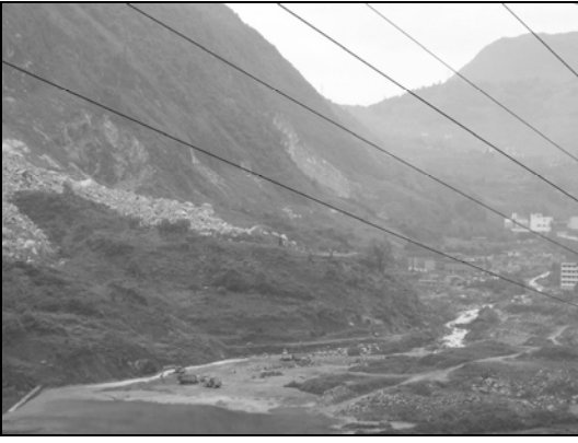
Fig. 10.6. Road clearing below landslide
