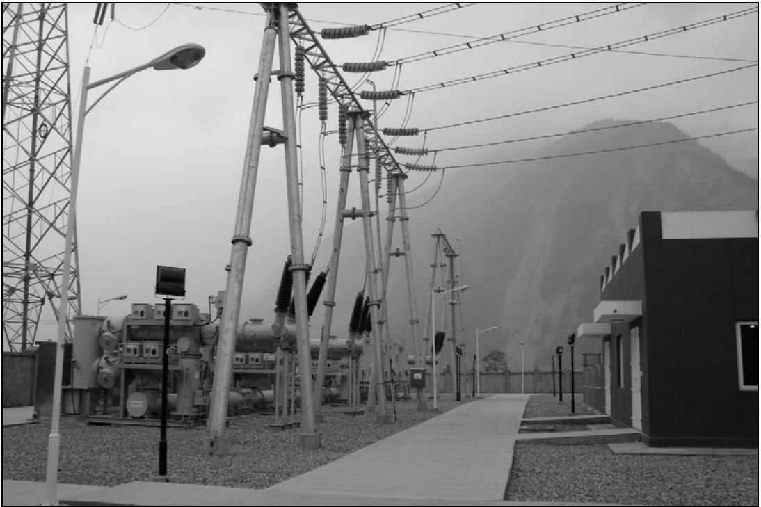
Fig. 4.78 Yingxiu, Ertaihan 220 kV substation rebuilt with one line working.
