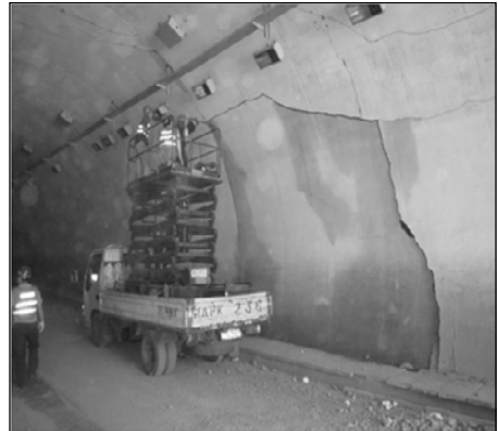
Fig. 3.83. Repairing liner damage (about 15 cm) (Courtesy CRSWRI)
