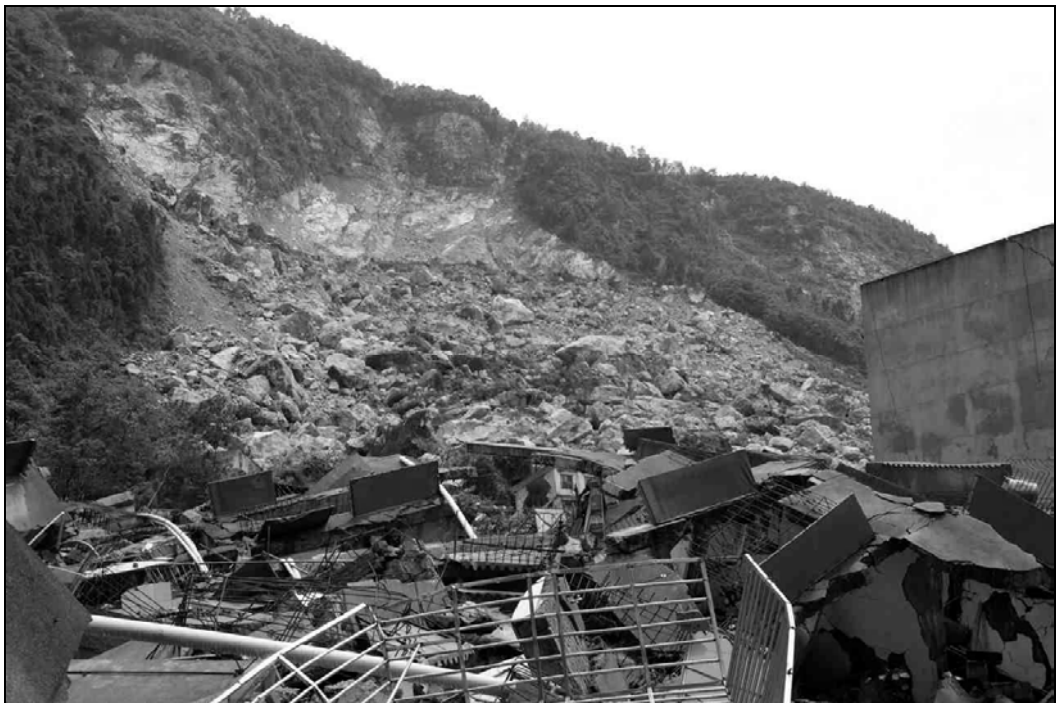
Fig. 9.20. View from a different angle to show the extent of rock fall and the debris of buildings being pushed to the low land
