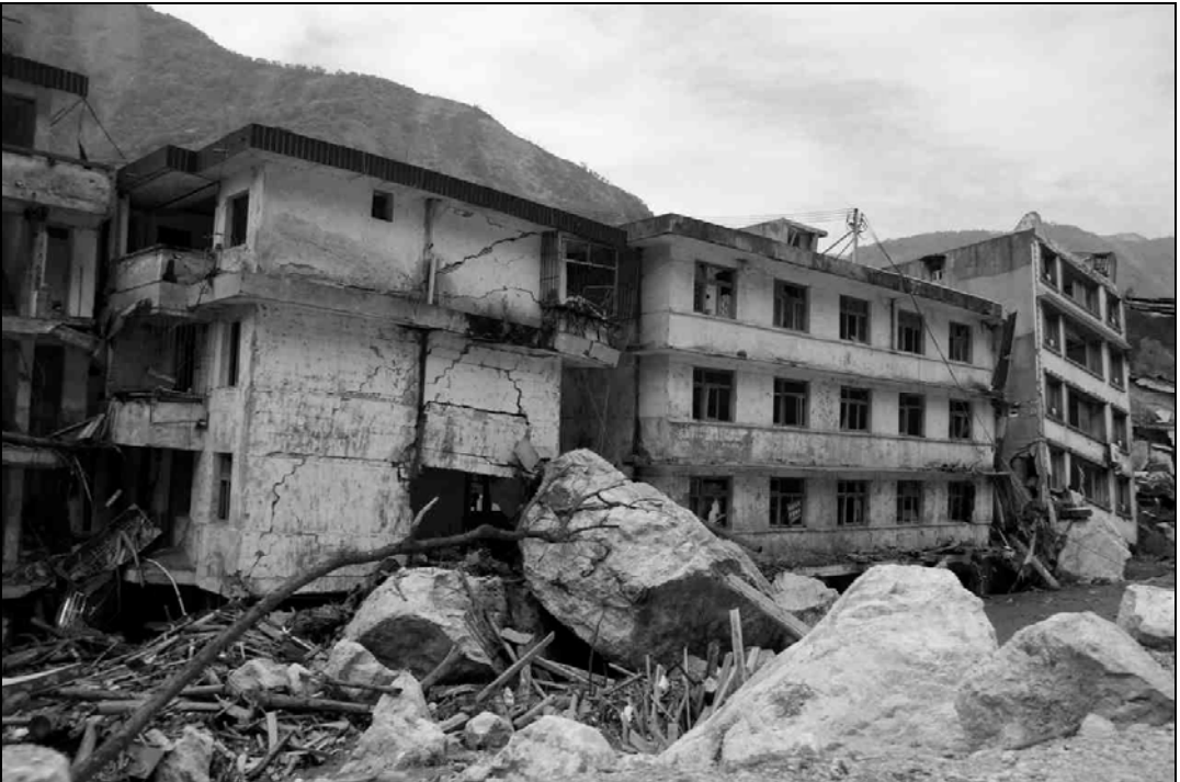
Fig. 9.26. Large boulders from the mountains were also a major cause of building damage.
