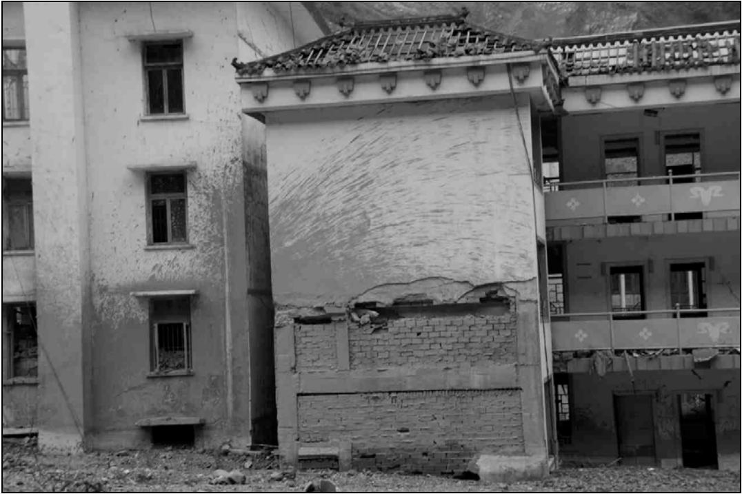
Fig. 9.23. This photo shows the force of the debris flow. The splash shot up two floors.
