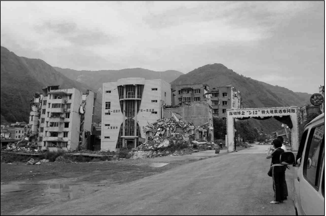
Fig. 9.27. Not all buildings were damaged; here one remained standing while the one next to it collapsed.
