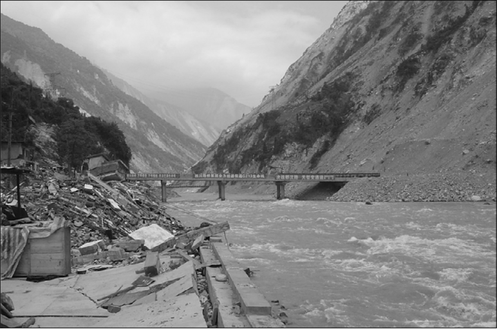
Fig. 3.37. Landslides, surface faulting, damaged Ming Jiang Bridge, and other structural damage in Yingxiu Village
