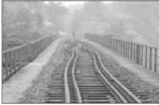
Fig. 3.88. Simple spans moved on their supports (Courtesy of Prof. Mei and Dr. Zhang)
