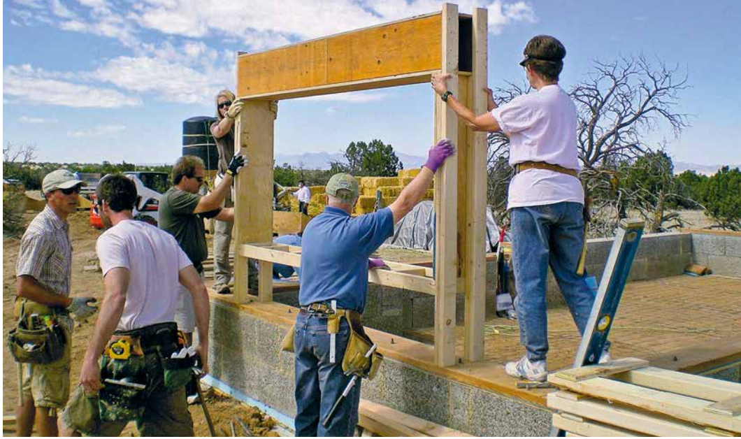
Students installing a window buck.
