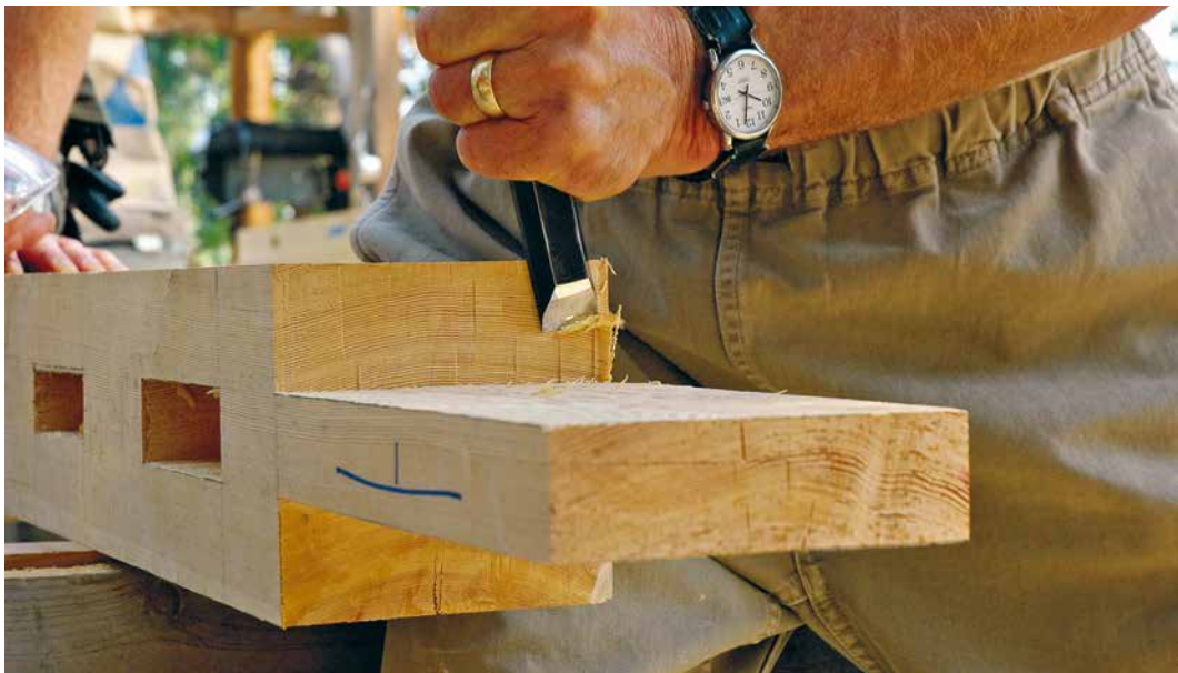
Chisel clean-up of tenon joint.
