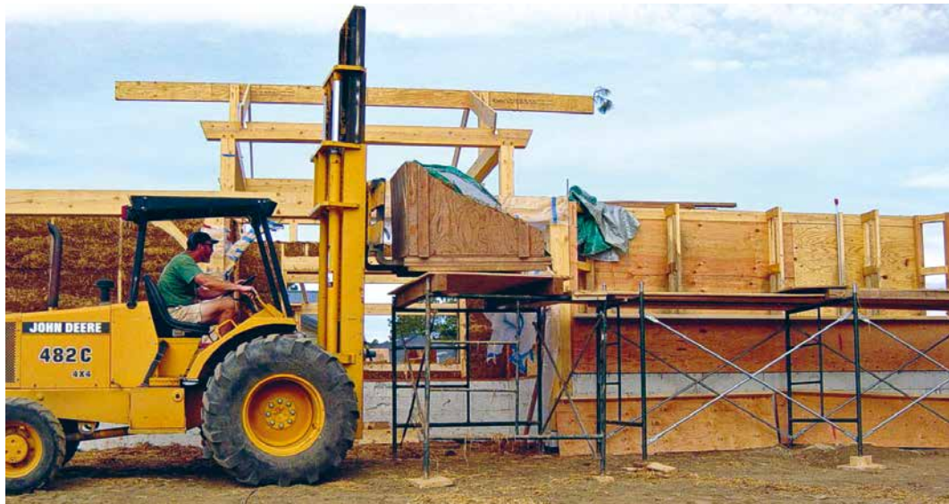
Forklift setting hopper on platform.
