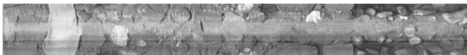
Fig. 5b. Core obtained by the wall of the Chapel in the zone of the right circular staircase
