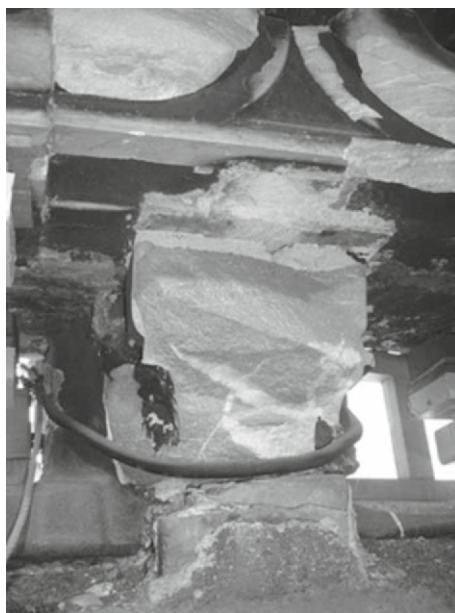
Fig. 19. The partial destruction of a modillion reveals decoration in bas-relief on the intrados of a marble arch even on the part covered by the modillion
