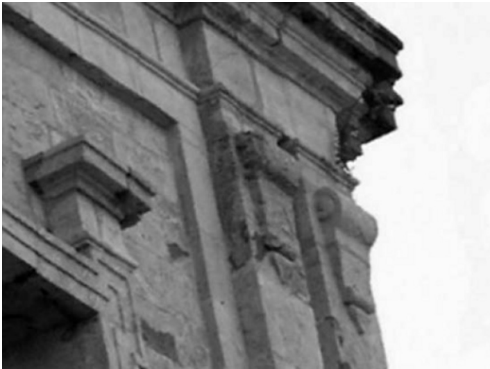
Fig. 16. Brackets on the pilasters of S. Agata, Ali
