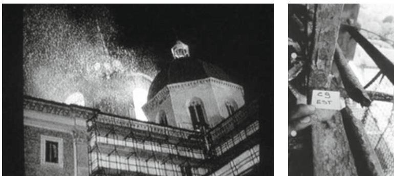
Fig. 9. left, the hot smoke coming out of the windows during the fire; middle, the broken ties
