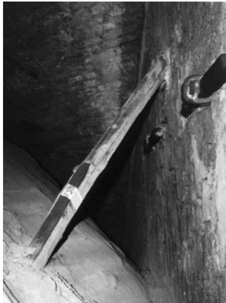
Fig. 16 (left). Inside the double structure, at the extrados of the conical arches of the Serlian window; note that the iron tie-rod passes parallel to but does not touch the main arch, as shown in drawing no. 295/1 (fig. 14)
