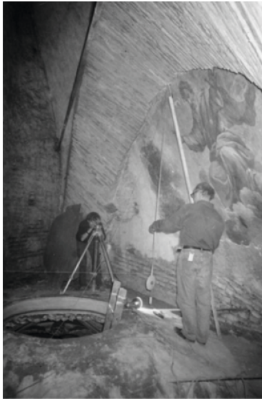
Fig. 20. Inside the hidden space of the conical vaults; note the arch constructed to consolidate the intrados and the iron tie-rod
