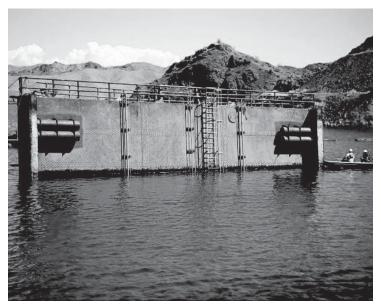
Figure 2-23. Single-piece floating bulkhead being positioned.
