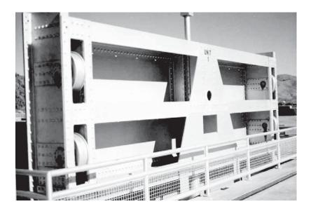
Figure 2-35. Wheel-mounted gate (Courtesy of USBR).
