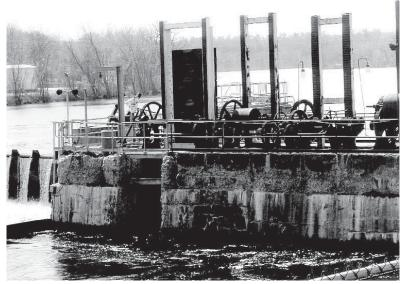
Figure 2-68. Rack and pinion gate operator.
