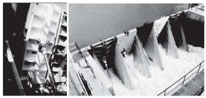
Figure 2-21. Hydraulically actuated wicket gates (Courtesy of USACE).
