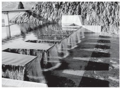
Figure 2-57. Labyrinth fuse gate (Courtesy of USBR).
