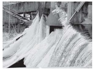
Figure 3-3. Icing of spillway gates.
