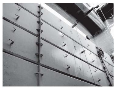
Figure 2-24. Articulated floating bulkhead, installed.
