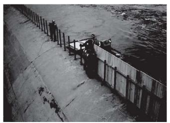
Figure 2-13. Installation of pinned flashboards.
