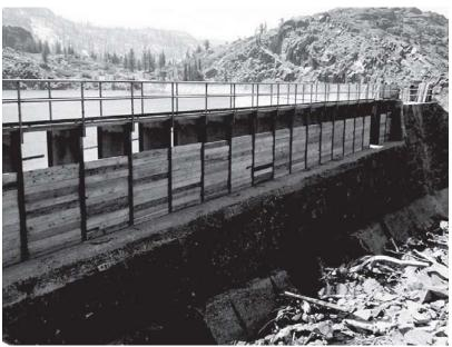
Figure 2-16. Fixed frame flashboards.
