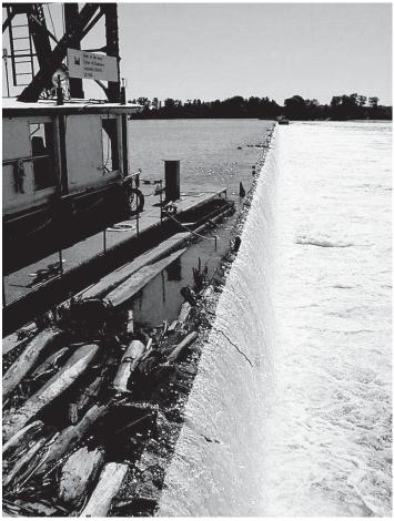
Figure 2-19. Wicket gates (manual placement type) (Courtesy of USACE).
