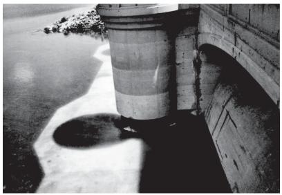
Figure 2-54. Intake with operating cylinder gate (Courtesy of USBR).
