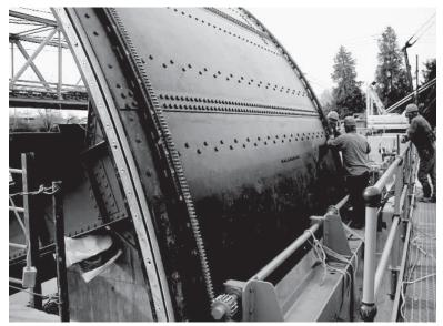
Figure 2-67. Rack and pinion gate operator.
