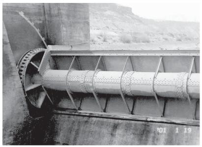
Figure 2-32. Non-submersible roller dam gate (Courtesy of USBR).
