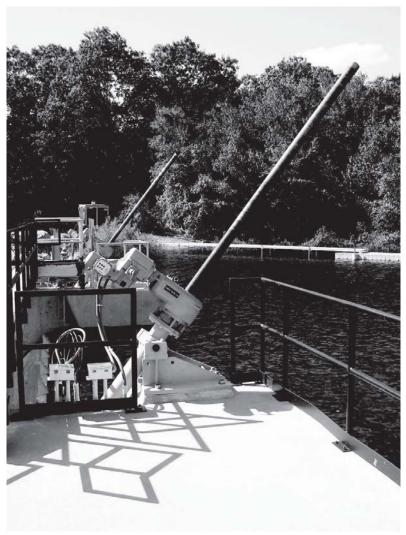
Figure 2-69. Screw stem gate operator.
