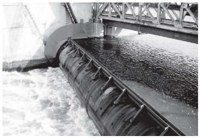
Figure 2-33. Roller dam gate (Courtesy of USACE).
