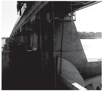
Figure 2-66. Link Chain (Courtesy of USACE).
