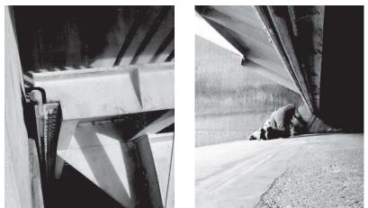
Figure 2-59. Radial gate seals. (Courtesy of HDR Engineering, Inc.)
