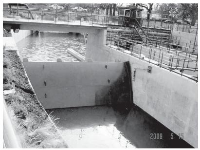
Figure 2-9. Double skinplate torque tube hinged crest gate.
