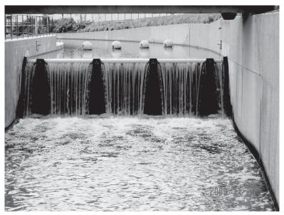
Figure 2-10. Double skinplate torque tube hinged crest gate.
