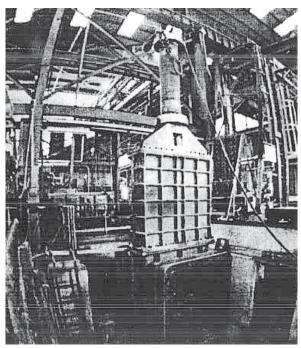
Figure 2-41. High pressure bonneted gate (Courtesy of USBR).
