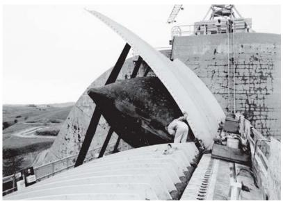
Figure 2-28. Steel-faced inflatable gate (Courtesy of USBR).
