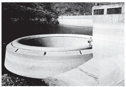
Figure 2-55. Ring gate (Courtesy of USBR).
