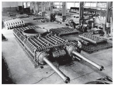
Figure 2-38. Paradox gate (Courtesy of USBR).
