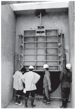
Figure 2-47. Sluice gate outlet work (Courtesy of USBR).
