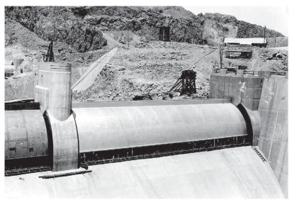
Figure 2-6. Drum gate in raised position (Courtesy of USBR).
