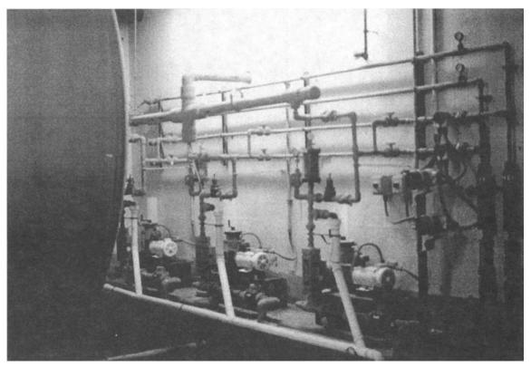
Photo 5.1 Alum sulfate pumps, feeds, and piping.
