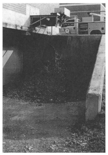
Photo 4.5 Debris screened from water intake.
