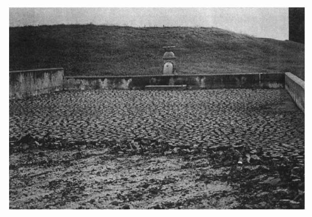
Photo 24.4d Sludge drying bed (process finished).
