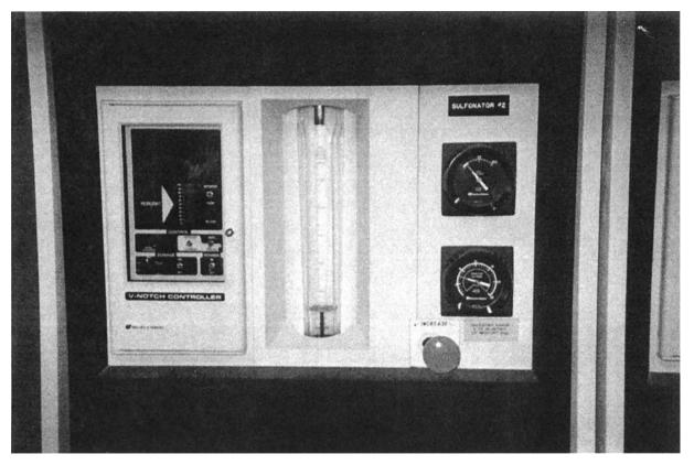
Photo 19.2 Sulfonator control panel.
