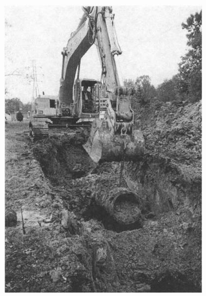
Photo 13.4a Removing broken interceptor pipe.
