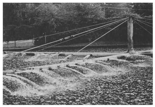
Distributor arm on trickling filter.
