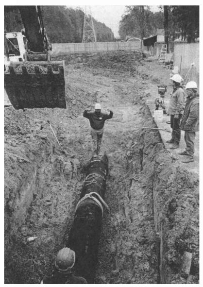
Photo 13.4b Replacing interceptor pipe.
