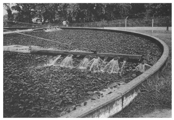
Photo 16.3 Trickling filter.
