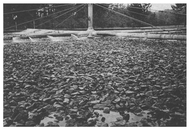
Photo 16.2 Trickling filter media.
