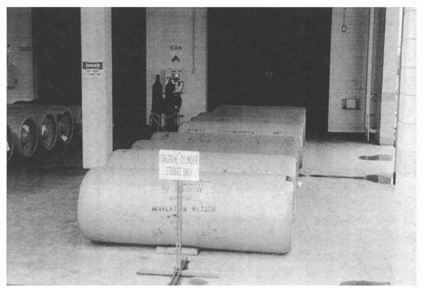
Photo 8.1 One ton chlorine tanks.
