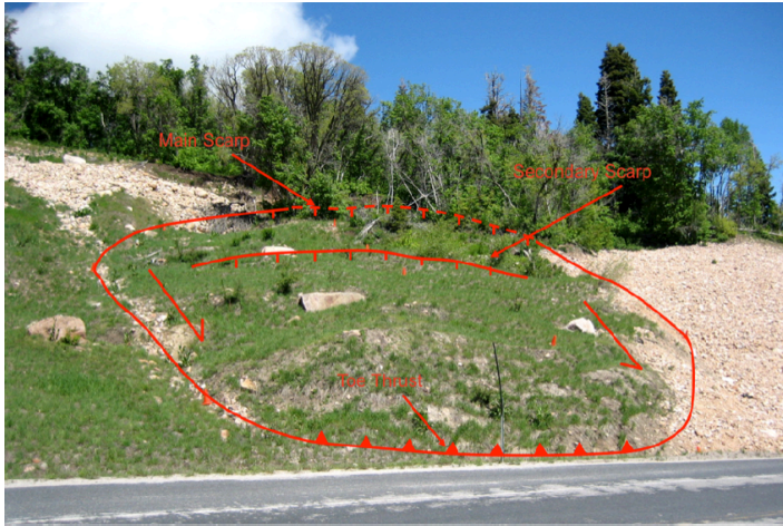
Figure 2. Image of Zigzag Sign landslide.
