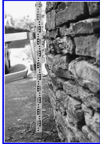
*Figure 6.2* A levelling staff used to assist observation of a bulging section of wall adjacent to a wall that has failed.
