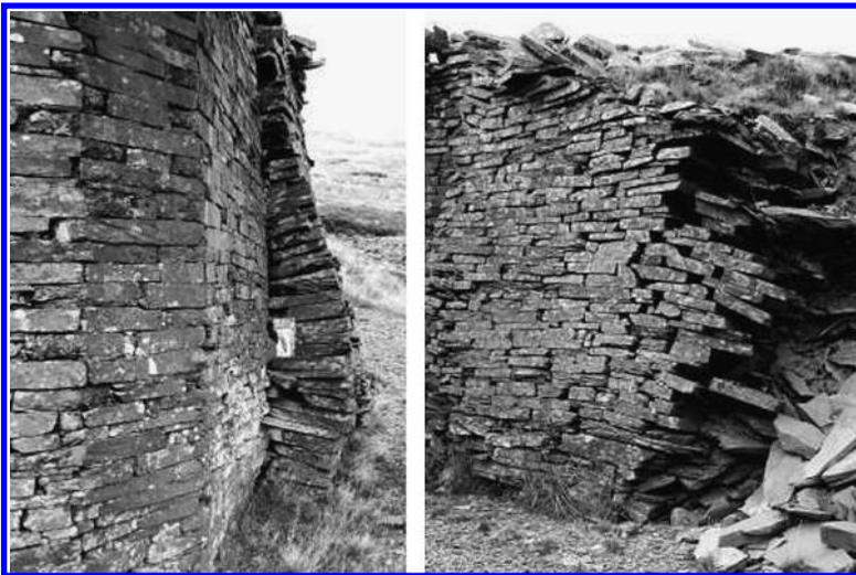
*Figure 6.6* A bulging drystone retaining wall in slate. (Courtesy of Professor William Powrie.)
