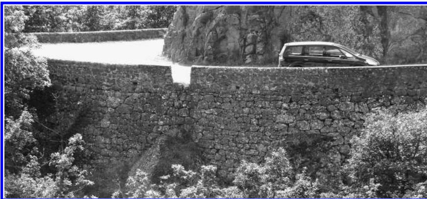
*Figure 1.4* Example of road with drystone retaining wall, Lozère, France.
