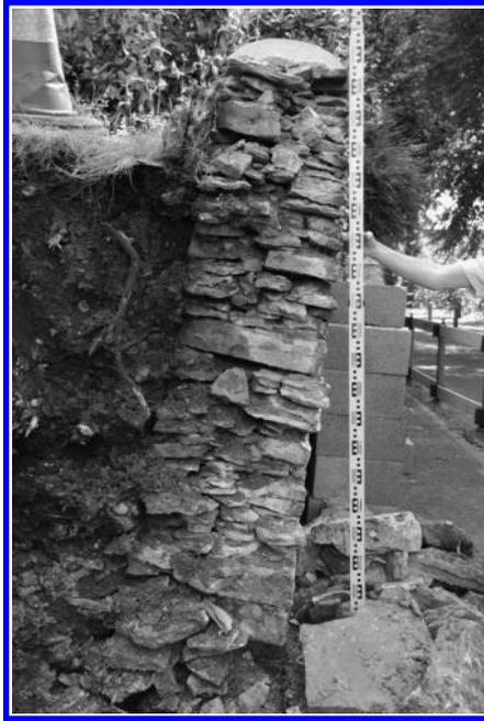
*Figure 6.10* The wall on one the other side of the same failure. The wall has a severe lean but is otherwise intact. Concrete blocks have been placed in front of the wall to prevent it from falling over.
