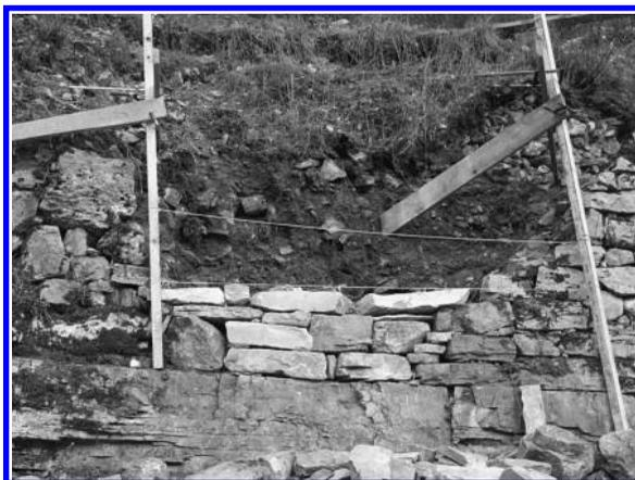
Figure 5.19 Template with a double line (limestone wall at Hauterives, France).
