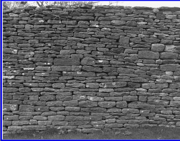
*Figure 1.1* A coursed masonry, limestone wall.
