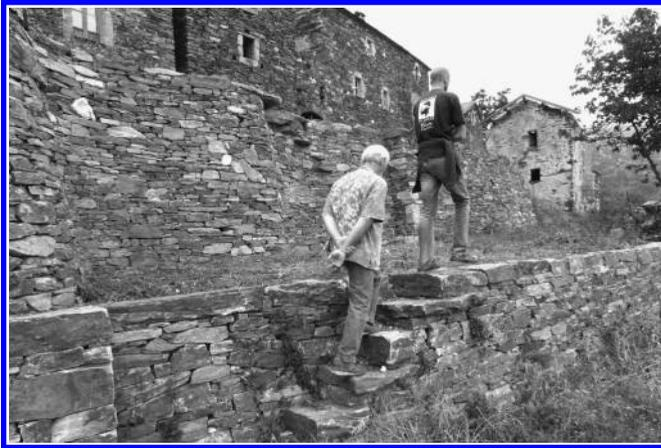
*Figure 1.3* Example of agricultural terrace with drystone retaining wall, Vialas, France.
