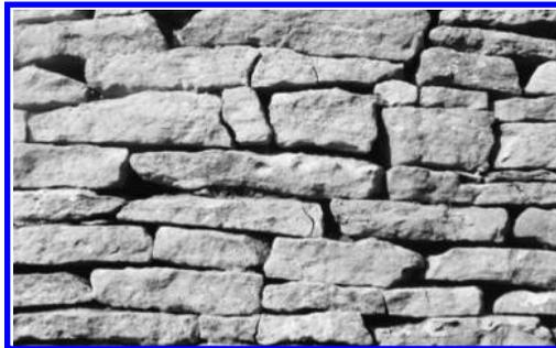
*Figure 6.1* A number of cracks are visible in the stones in this photograph, all of which probably took place as the wall was being built.
