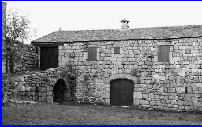
*Figure 1.5* A farmstead in the Cévennes, constructed of granite placed without mortar. Some recent pointing is visible in part of the wall.
