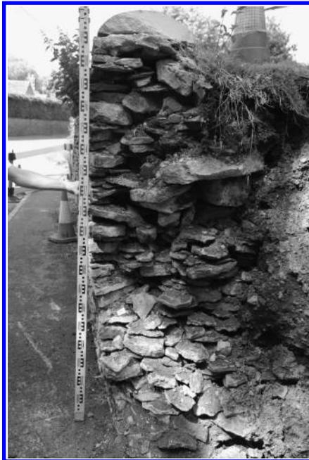
*Figure 6.9* The wall on one side of a failure. Front and back faces can be seen, and the fill between the two has expanded as the front face pulled away.
