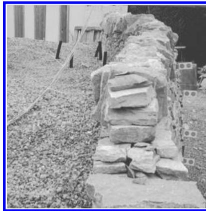
**Figure 3.11** Catenary action. (a) This view is looking down on a line of stones in the face of a wall. Tensile strength along the face enables the stones to resist localised lateral pressure, distributing the load to adjacent sections of the wall. (b) This view is looking along the top of a test wall that was built straight, and is now bulged outward, so catenary action helps to redistribute the concentrated load.
