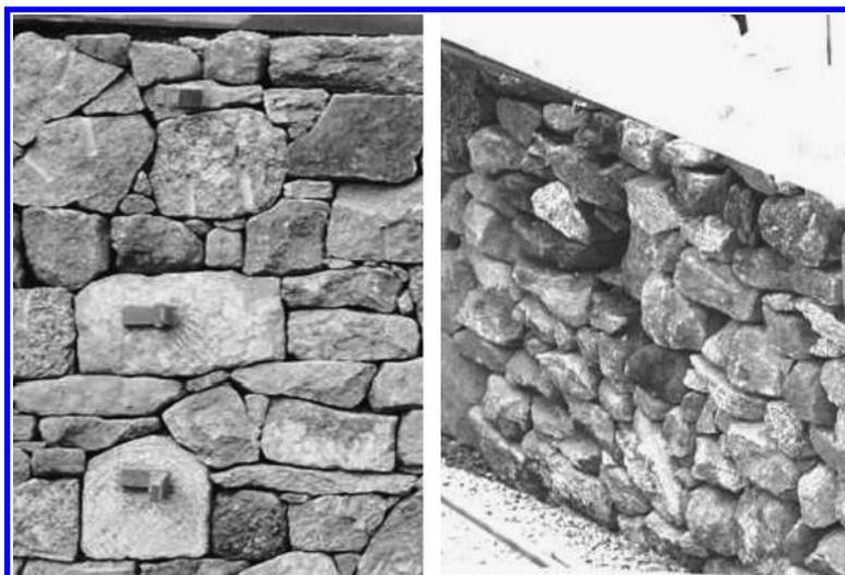
*Figure 3.15* Front and back faces. These two photographs show the front and back face of the same wall. The difference in density of the construction is immediately apparent.
