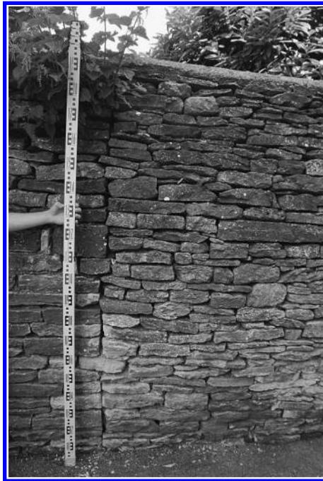
*Figure 6.3* A very poor junction between adjacent sections of a limestone wall.
