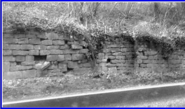
Figure 6.7 A wall adjacent to a highway, in very poor condition with stones falling from the face.
