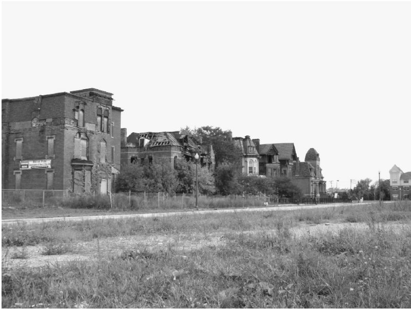
Figure 6.7 Dilapidated housing stock, Detroit (author's photograph)
