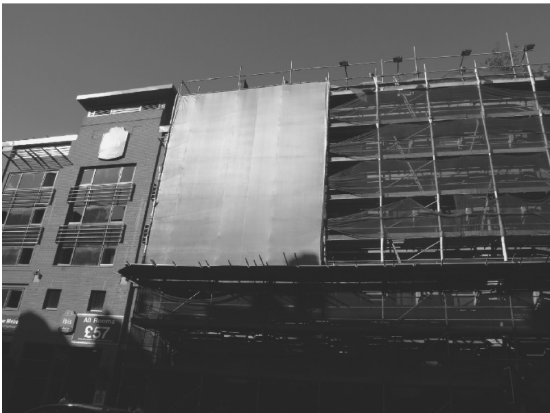
Figure 6.2 Manchester renovation and advertising wrap (author’s photograph)
