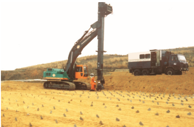
Fig. 4.15 Photo of vertical prefabricated drains installation
