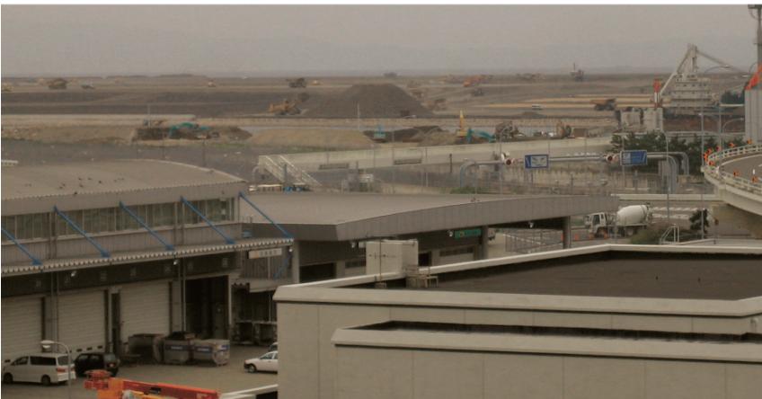
Fig. 6.82 Photos of second phase construction of Kansai International Airport
