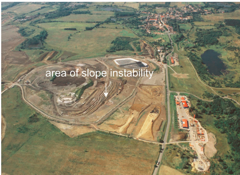
Fig. 8.73 Chabařovice landfill. Aerial view during remediation
