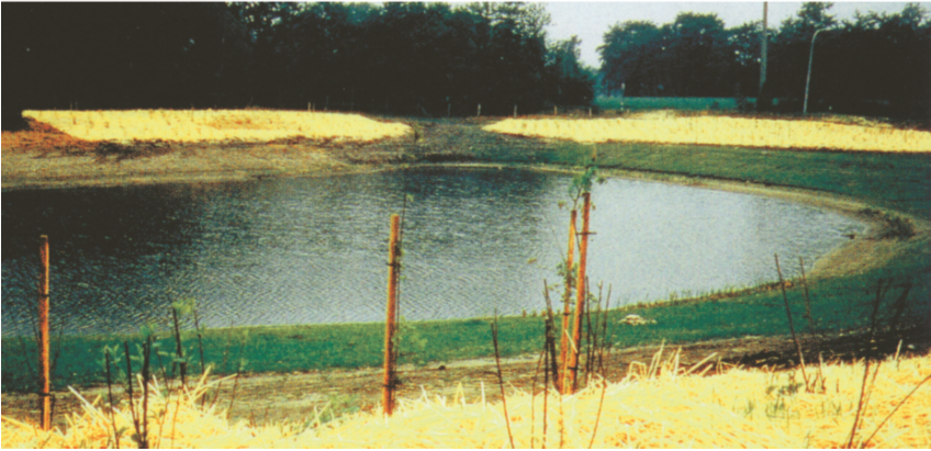
Fig. 6.86 Photo of settling pond near motorway. (a) During construction. (b) In use
