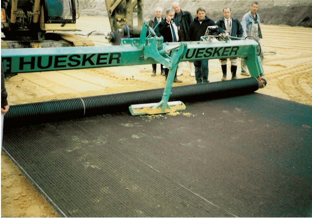
Fig. 3.20 Photo of geogrid installation with certain pretensioning at Gröbers project
