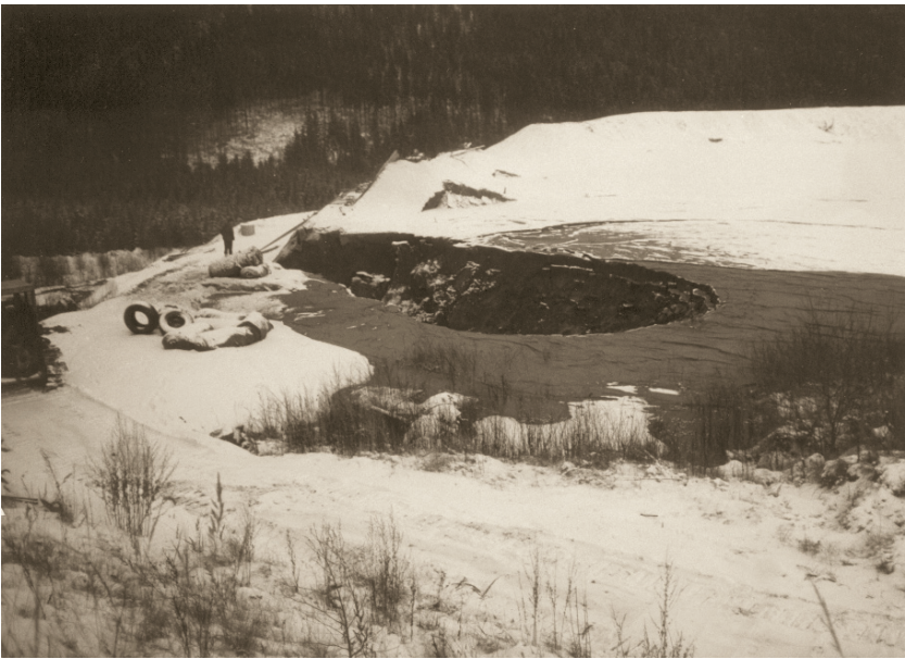
Fig. 8.40 Ditch created by surface water erosion at Zlaté Hory tailings dam. (a) general view. (b) detail of gash
