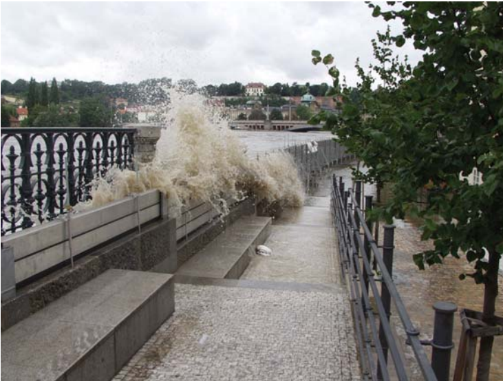
Fig. 7.74 Additional protection barrier applied during heavy floods in Prague (photo courtesy of Hydroprojekt Praha)
