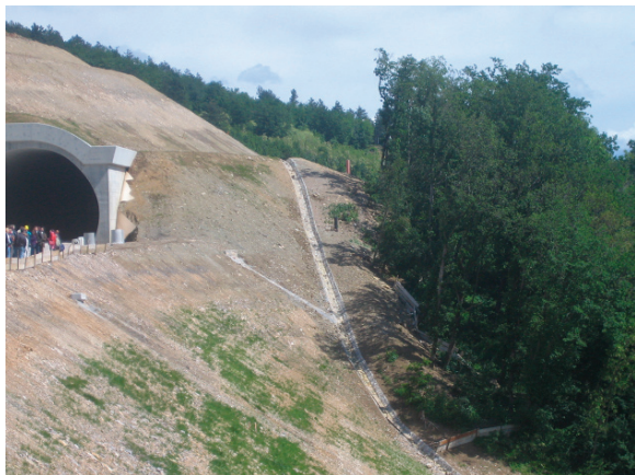
Fig. 5.42 Photo of surface water channel on embankment slope
