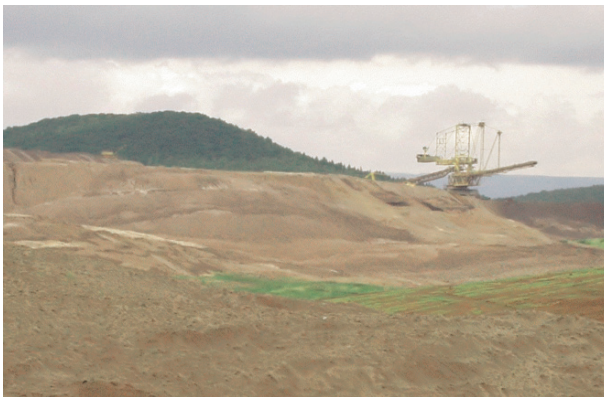
Fig. 8.2 General view on spoil heap during its construction – filling
