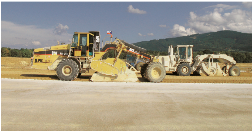
Fig. 4.18 Cutter for production of soil stabilization (Photo Bartozela)
