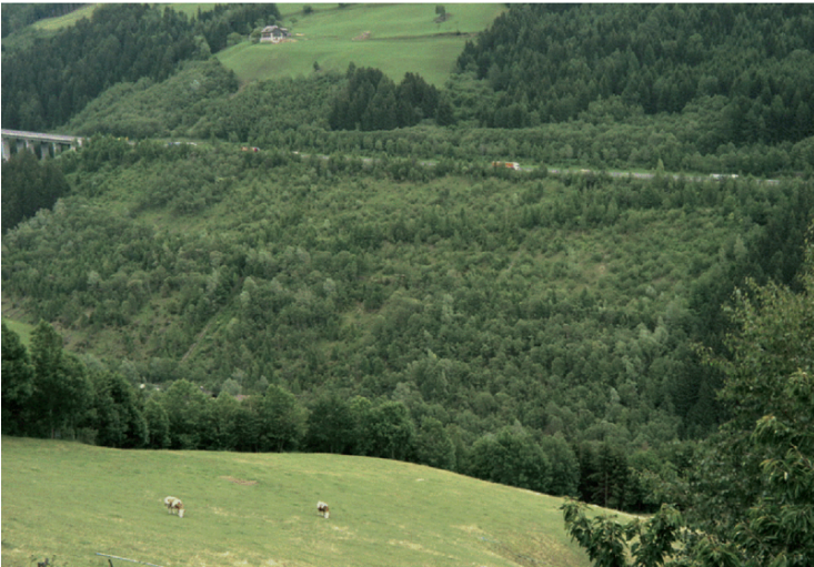
Fig. 6.6 Photo of 100 m high embankment – photo Brandl. (a) Shortly after the end of construction (1979). Slope erosion protection with rhombus-shaped bio-reinforcement (willow branches etc.) that led to stable vegetation. (b) Detail to (a) – the embankment has become part of the natural environment
