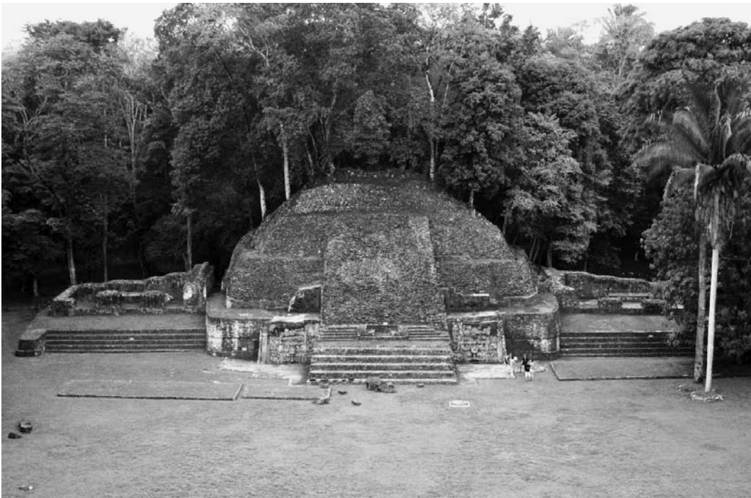
Figure 6.5. Photograph of Structures B4–B6 at Caracol, from left to right (photograph by the author).
