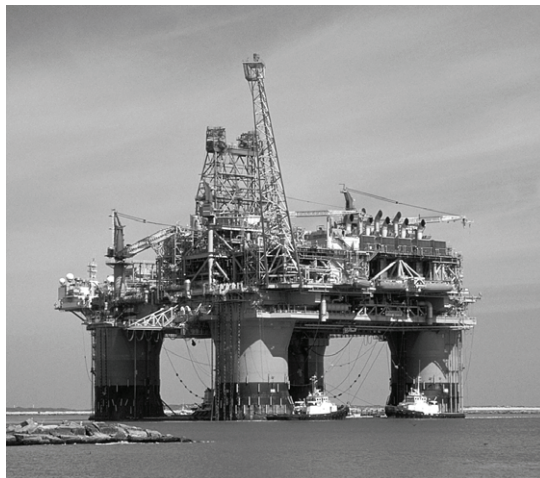
Photo Courtesy of BP © Press Images: Thunder Horse Oil Platform (image highlights the location of a typical pipeline welding job)
