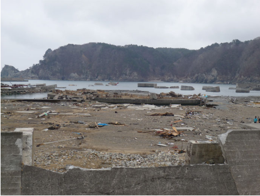
Fig. 5.2 Collapse of a large seawall in Taro district of Miyakoshi City, Iwate Prefecture, after the 2011 Great East Japan Earthquake (Photo by K. Yamori)
