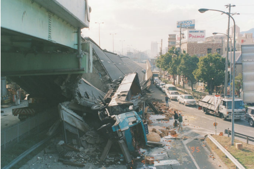
Fig. 5.1 Collapse of elevated expressway in the Great Kobe Earthquake in 1995
