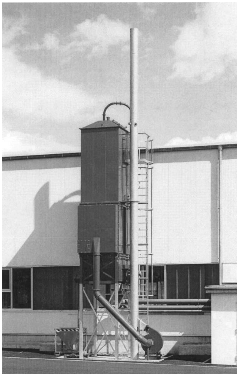
FIG. 4 Exhaust gas absorption unit for fluorine pretreatment of plastic parts. (Courtesy of Fluor Technik System GmbH, Lauterbach, Germany.)
