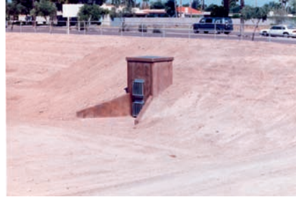
(b) Outlet structure for pond
