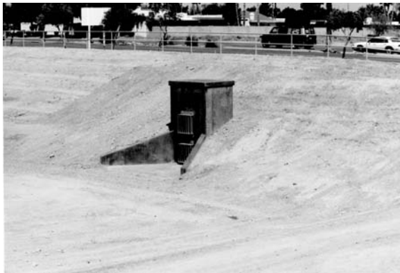
(b) Outlet structure for pond
