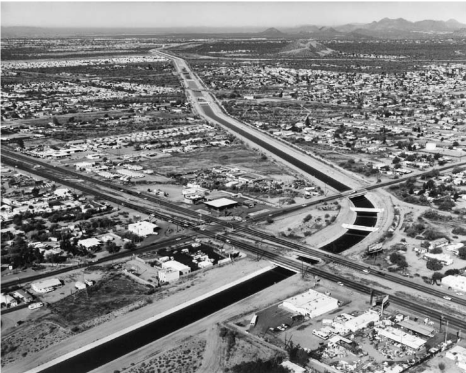
Figure 3.14 Central Arizona Project aqueduct through residential area in Scottsdale, Arizona (See also colour plate 6)
