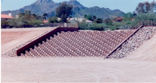
(a) Intake structure to detention pond
