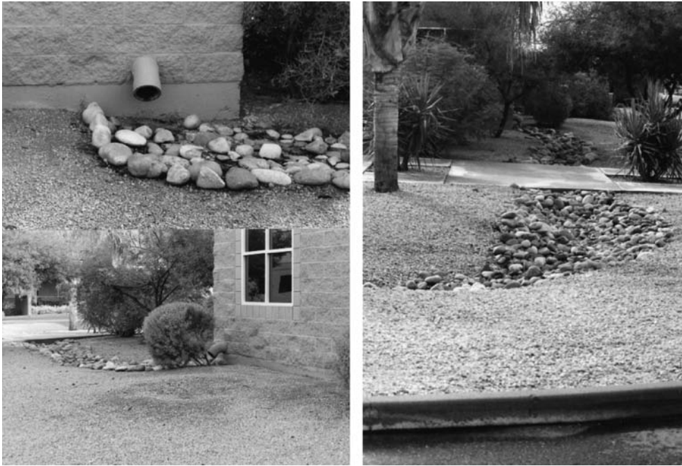
Figure 4.2 Showing rooftop drainage flowing into infiltration bed (photos by L.W. Mays) (See also colour plate 7)
