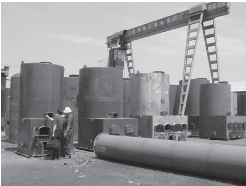
Plate 6.1 Yang Wenzhu's 'Xinzhou Welfare Boiler Plant of Shanxi Province' located in the centre of Yuanping City
