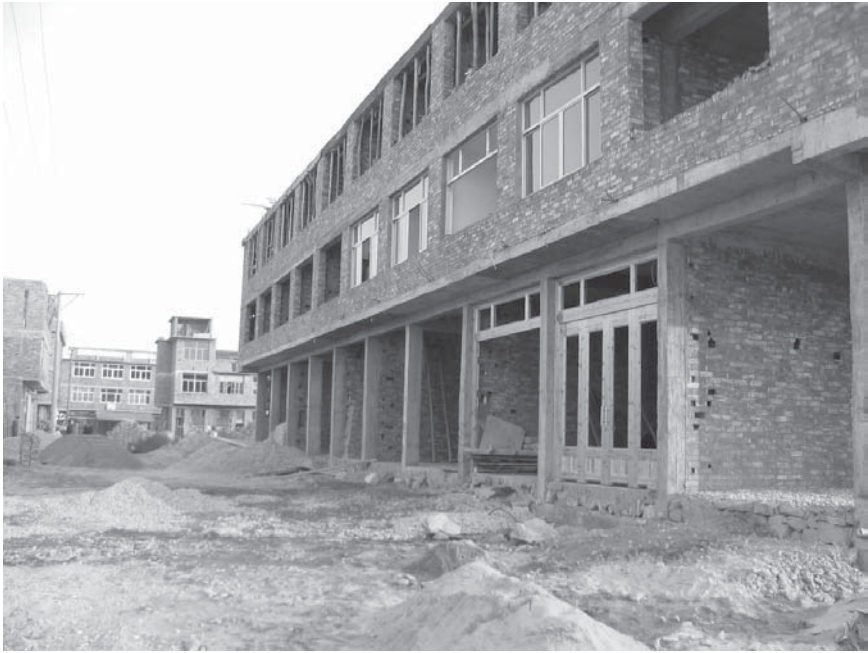
Plate 4.3 New houses under construction for immigrants in Xiangdong village
