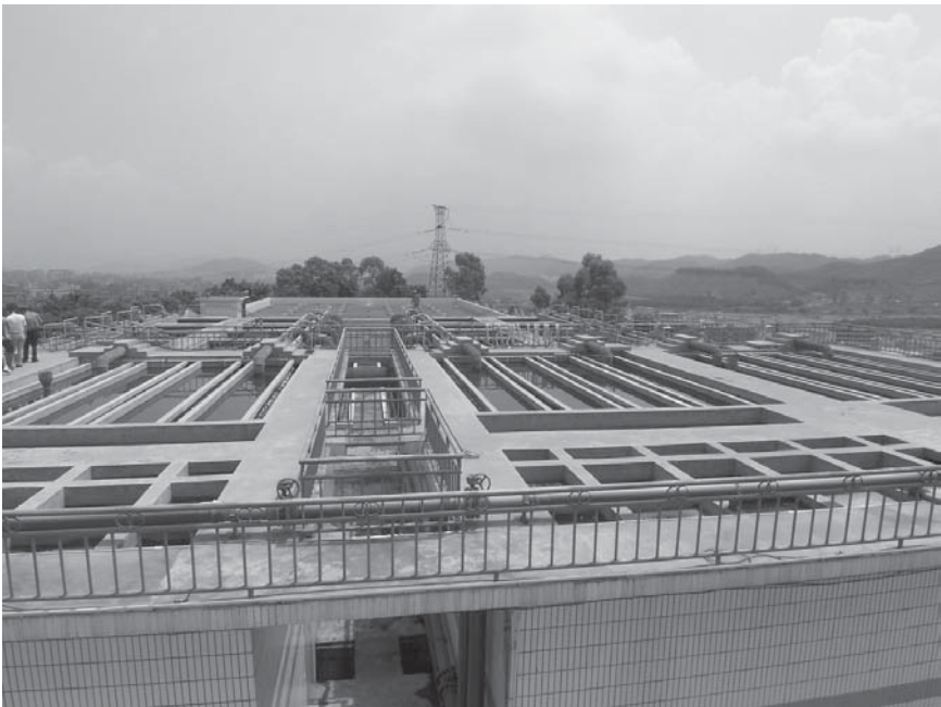
Plate 7.3 The usage rights in one of the sewage treatment plants has been transferred to a local entrepreneur through contract arrangements
