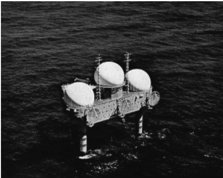
Figure 1.1 Texas Tower 2, off New England (photo courtesy US Coast Guard).
