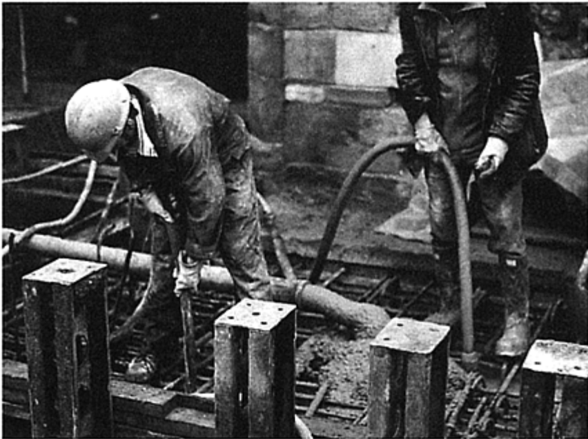
Figure 1.2 Compaction with poker vibrations ( Photo Courtesy of Ove Arup Partnership ).
