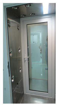
Fig. 7 Air shower; isolates classified processing area from other unclassified spaces (e.g., support room, gowning, and scrubbing area)
