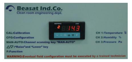
Fig. 6 Automated clean room environmental controls for air pressure, humidity, and temperature
