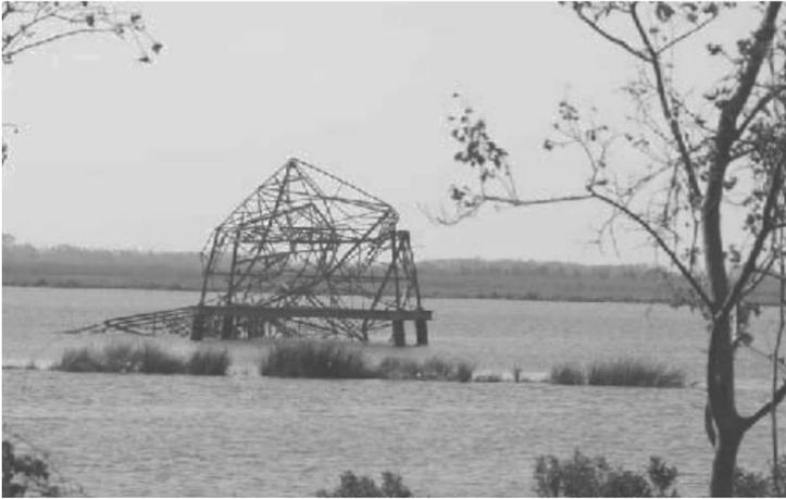
*Figure 4.1.17 Electrical Transmission Tower – Hurricane Rita
