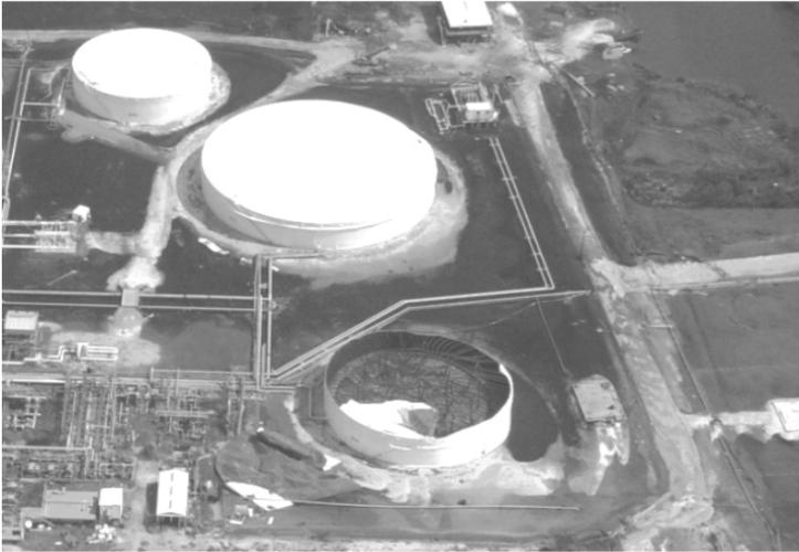
*Figure 4.1.9 Tank Damage - Hurricane Katrina
