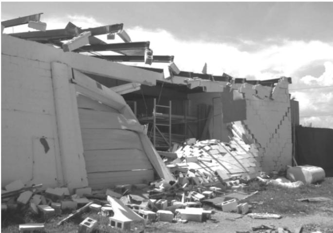
*Figure 4.1.3 Building with Masonry Infill – Hurricane Charley*
