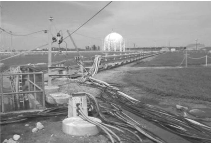
*Figure 4.1.5 Cable Tray Damage – Hurricane Frances
