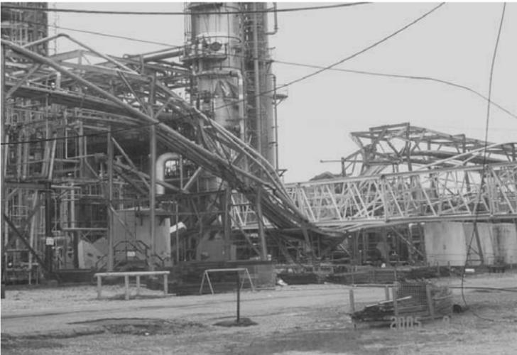
*Figure 4.1.20 Crane Boom across Pipe Rack – Hurricane Rita
