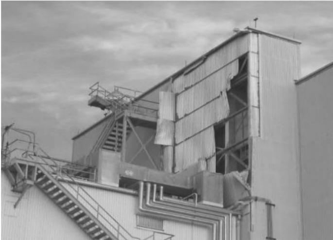
*Figure 4.1.6 Cladding Damage – Hurricane Frances
