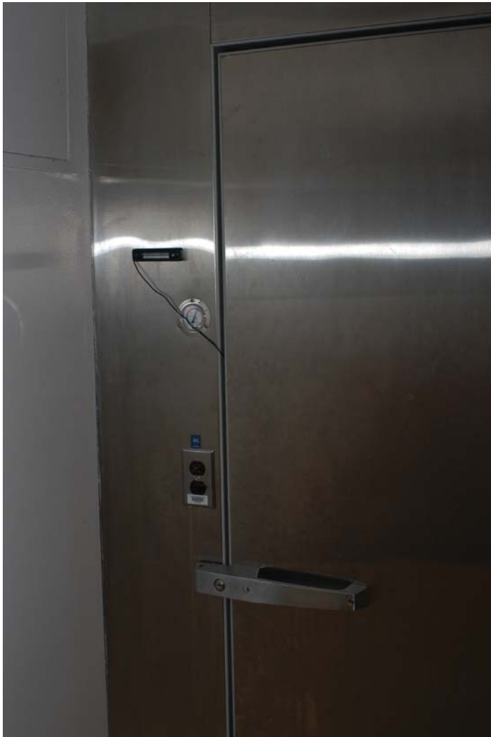
FIGURE 3.7 Lockable cooler. Bodies should be kept in a lockable cooler, and a registry of all valuables should be maintained. All activity in and out of the cooler should be logged. Cooler temperature is kept between about 38 and 42°F.
