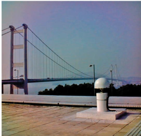
Figure 9.11 A GPS reference station on the roof of a storage building (from [5]) (Reproduced with permission from Taylor & Francis).
