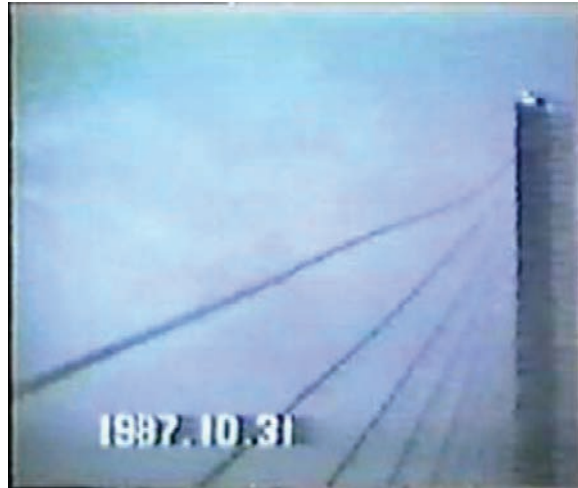
Figure 1.15 Rain-wind-induced vibration of stay cable (Source: Wind Induced Vibration of Cable Stay Bridges Workshop April 25–27, 2006 St Louis, MO FREYSSINET LLC ( http://www.modot.org/csb/documents/24-New-DevelopmentsinCableStayVibrationSuppression.pdf )).
