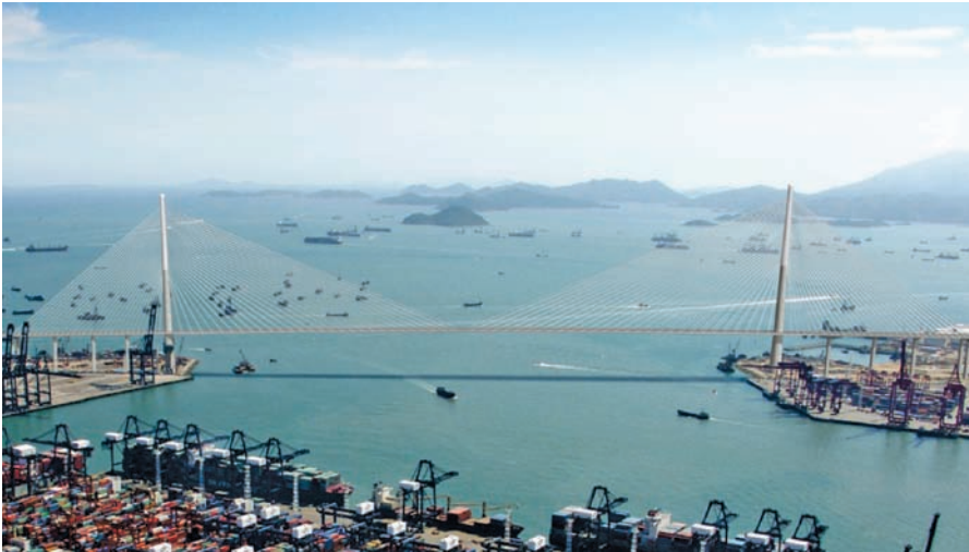
Figure 15.9 Stonecutters Bridge in Hong Kong.
