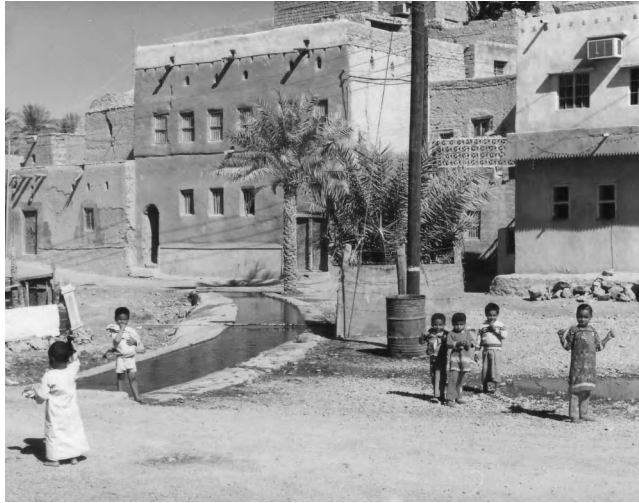
Figure 1.1 Open section of falaj (qanat) running through a village in northern Oman. Photo by Bruce Misstear
