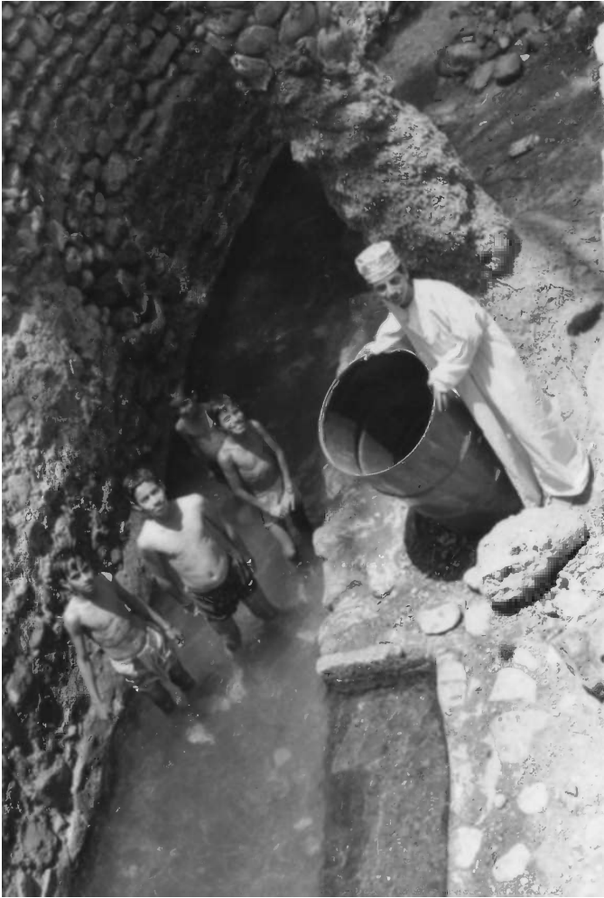
Figure B3.7(ii) The sharia section of a falaj, where the water first appears at the surface at the head of the village. Photo by Bruce Misteer
