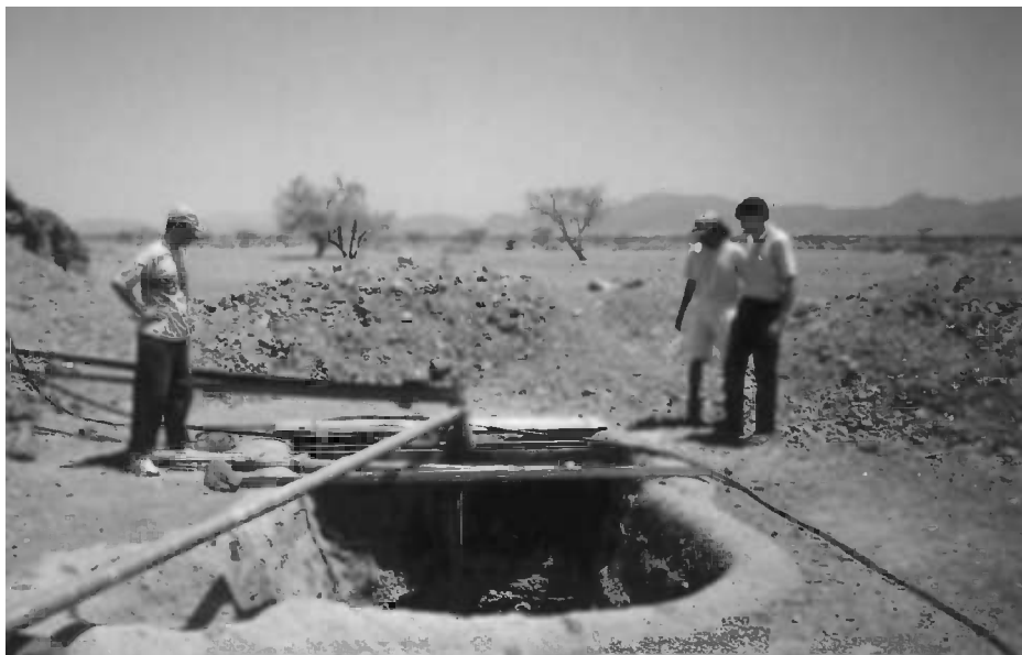
Figure 2.9 Examining a hand-dug well in northern Oman. The well is fitted with a belt-drive turbine pump. Note the excavated spoil material piled up behind the well, which can give a useful indication of the well geology. Photo by Bruce Misteear
