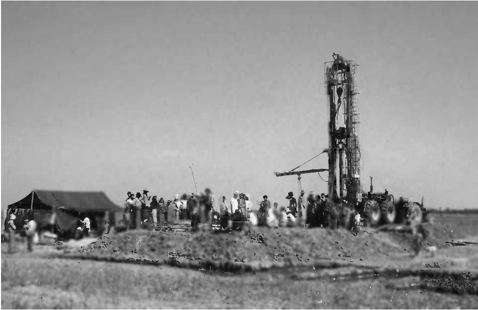
Figure 5.15 Tractor-mounted rotary rig raised above the ground surface in order to provide the necessary hydrostatic pressure for reverse circulation drilling. The target aquifer in this area of central Myanmar had a potentiometric surface only about 1–2 m below ground level. Photo by Bruce Misteear
