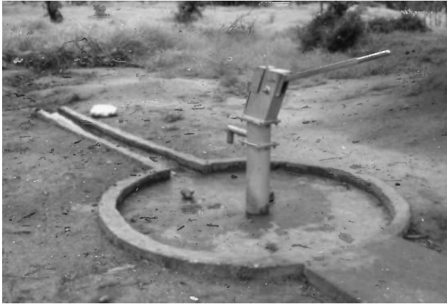
Figure 3.9 Concrete apron and drainage channel around a hand-dug well, Lower Nile province, Sudan. Photo reproduced by permission of Laurence Gill
