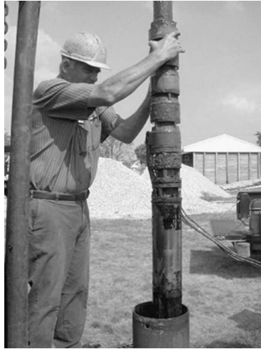
Figure 9.10 Biofouled submersible pump removed from a carbonate aquifer well, Ohio, USA. Iron oxide deposits are visible on the pump bowls, while a black iron sulfide slime can be seen on the motor. Reproduced by permission of Stuart Smith, Smith-Comeskey Ground Water Science LLC www.groundwatersystems.com
