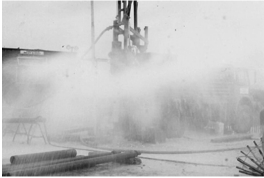
Figure 5.26 Vigorous well development using air-left pumping, eastern England. Photo by Bruce Misstear
