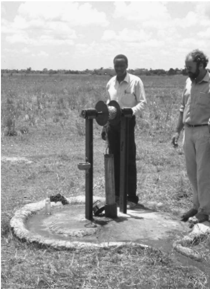
Figure 3.23 Bailer tube used in a rural Kenyan drilled well. Photo by David Banks
