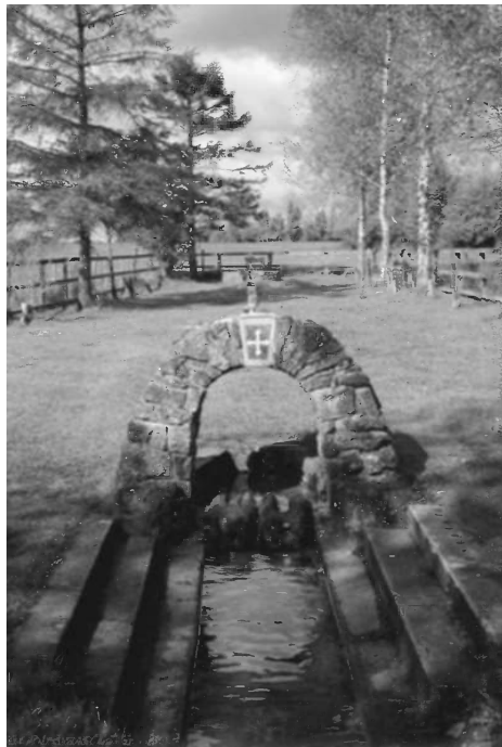
Figure B3.6(iii) St Brigid's well, County Kildare, Ireland. The well is located at the rear of the fenced area, behind the arch adorned with the white cross. The well is constructed around a small spring in a gravel aquifer and its discharge is channelled through two hollowed stones under the arch. The tree with the votive offerings shown in Figure B3.6(ii) is the second large tree from the left at the top of the picture. Photo by Bruce Misstear
