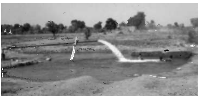
Figure 1.7 Flowing artesian well, northern Myanmar. The well was drilled into a strongly confined sandstone aquifer. Children are enjoying the 'swimming pool' created by the discharge until such time as the well is capped. Photo by Bruce Misstear
