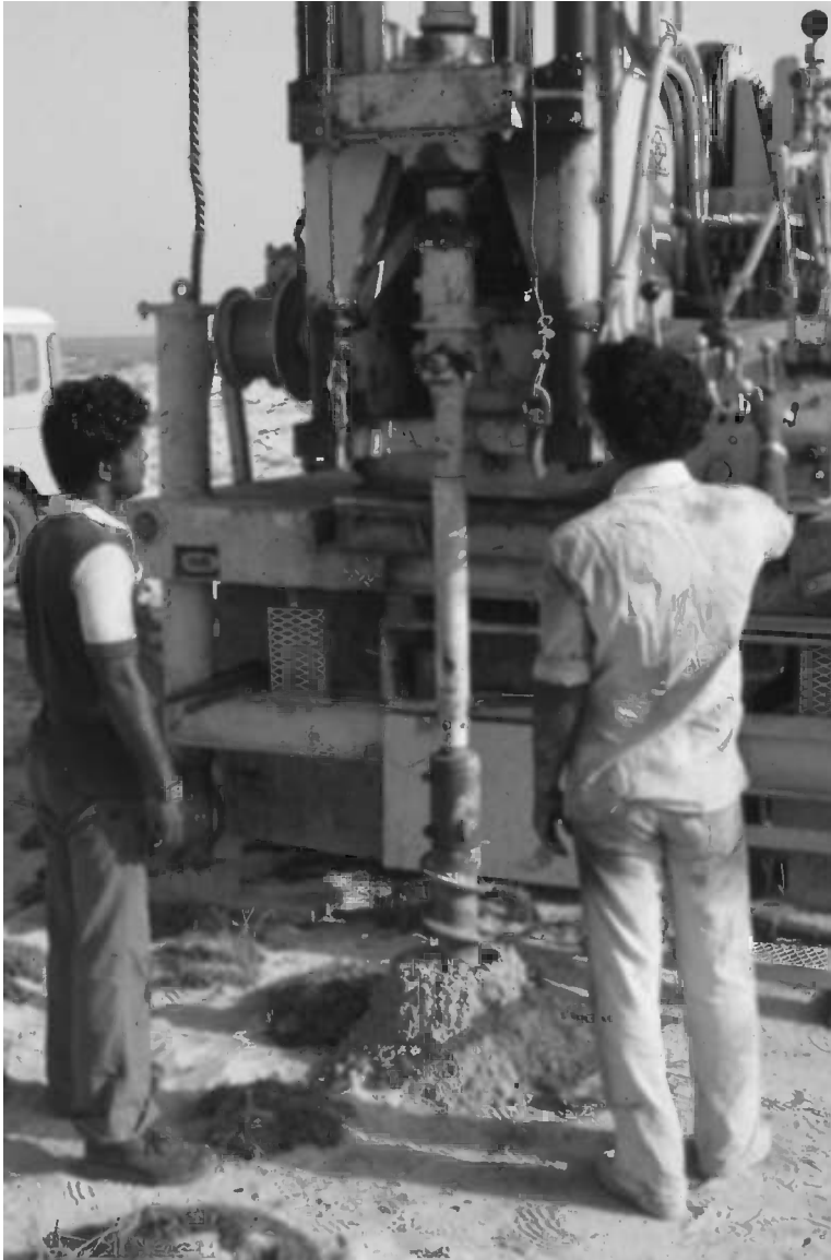
Figure 5.20 Hollow-stem auger drilling, Saudi Arabia. Photo by Bruce Misstear
