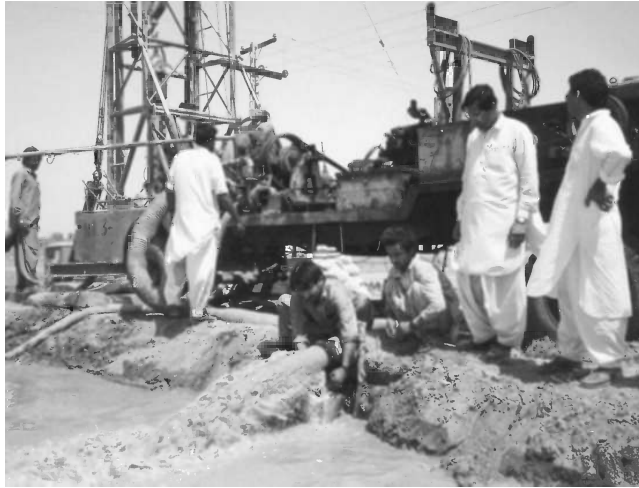
Figure 6.5 Collecting formation samples from reverse circulation drilling in Sind province, Pakistan. Photo by Bruce Misstear
