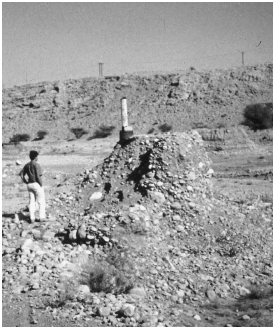
Figure 2.8 The remains of a well located in a wadi in northern Oman. The original wadi surface is preserved as a remnant mound around the top of the well casing. From the height of the hydrogeologist standing nearby, we can see that the wadi floor has been lowered by about 2 m due to erosion from the occasional, but violent, floods that occurred in the 20 year period between well construction and when this photo was taken. Photo by Bruce Misstear
