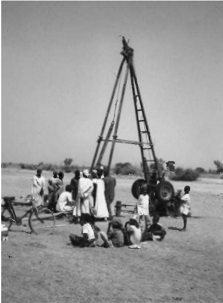
Figure 5.6 Light-percussion rig, northern Nigeria. Photo by Bruce Misstear
