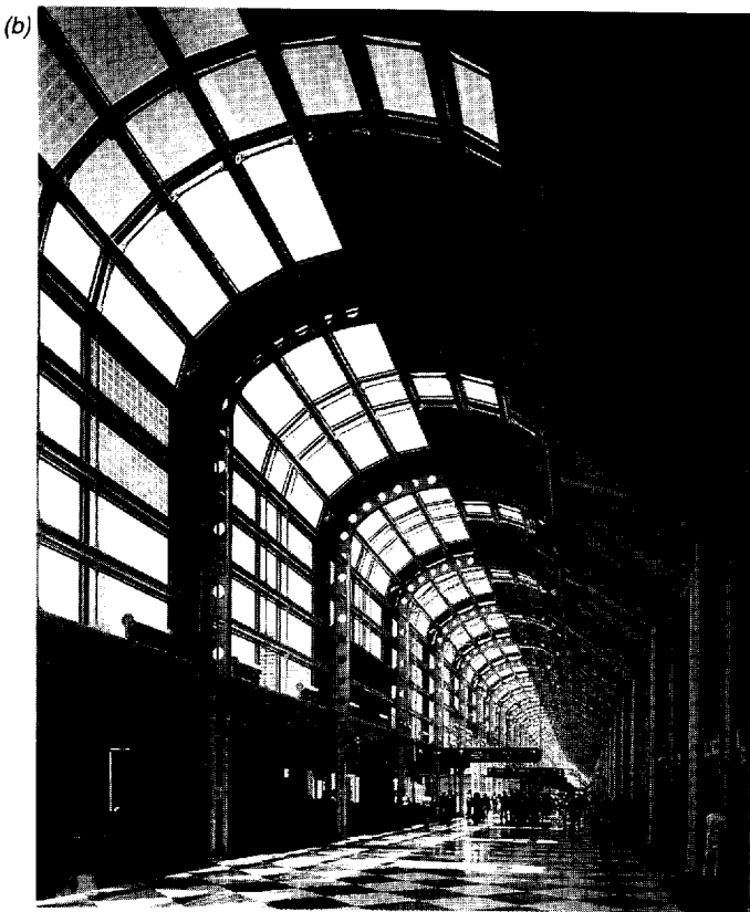
P.2 Chicago O'Hare United Airlines Terminal: (a) passenger tunnel; (b) departures concourse. Architects: Murphy & Jahn, New York.
