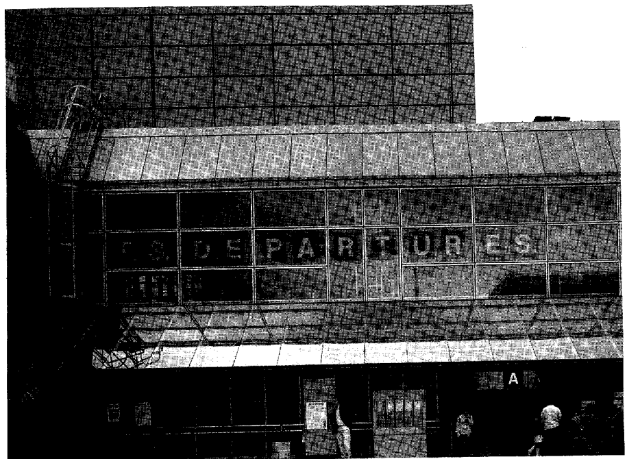
27.21 Exterior. Client: Heathrow Airport Ltd. Architects: D. Y. Davis Associates Ltd, Richmond, Surrey.
