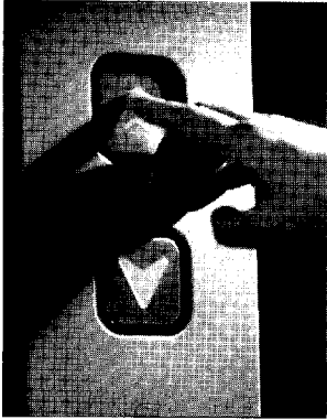
22.11 Lift buttons, easily seen, felt, understood and used. Figures 21.1–21.11 from Heathrow Terminal 4 . Architects: Scott Brownrigg & Turner, Guildford.
