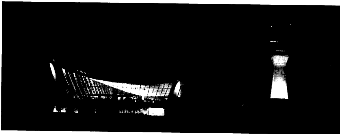
8.2 Washington Dulles by day and by night. Courtesy of US Department of Transportation.
