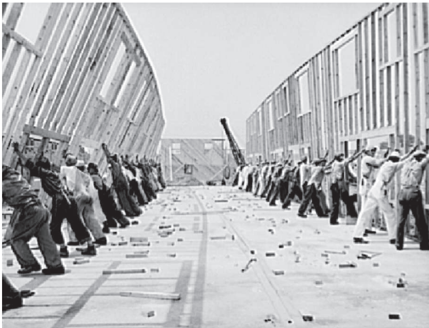
Fig. 2 Raising the framed walls of the balloon frame. 1941. (Alfred T. Palmer, photographer, 1941, Library of Congress, Prints & Photographs Division, FSA/OWI Collection, LC-USE6-D-000861.)
