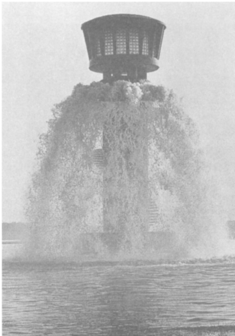
Inlet aerator discharging 200 MI/day to Grafham Reservoir of Anglian Water, UK
