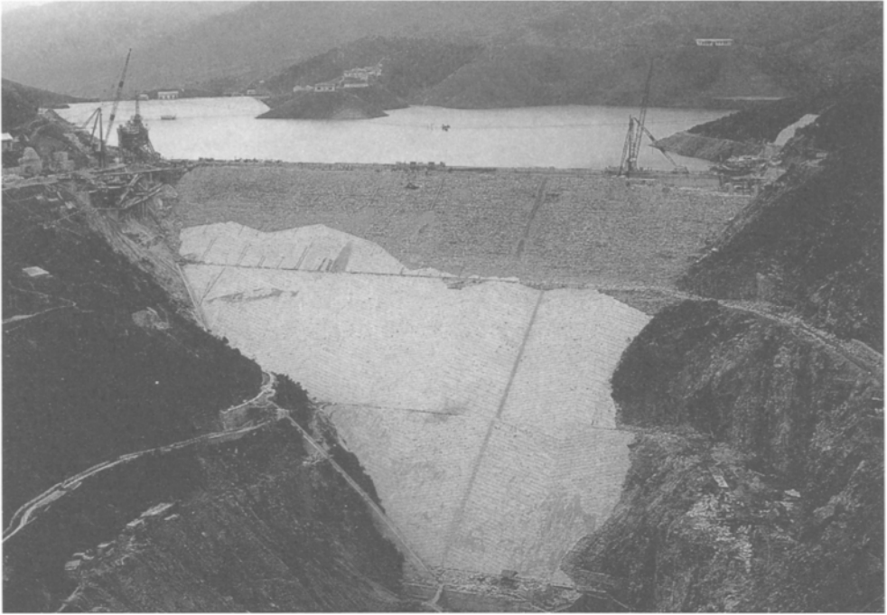
The 85 m high Gorge dam of the Shing Mun water scheme for Hong Kong, comprising a concrete block diaphragm upstream, supported by a concrete thrust block and a downstream rockfill embankment, completed 1936. (Engineers: Binnie & Partners)
