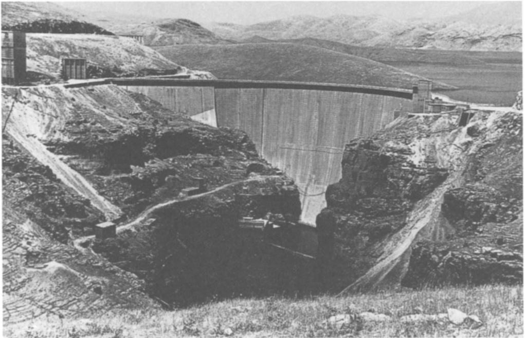
The 116 m high concrete arch dam at Dokan, Iraq, completed in 1959. (Engineers: Binnie & Partners)
