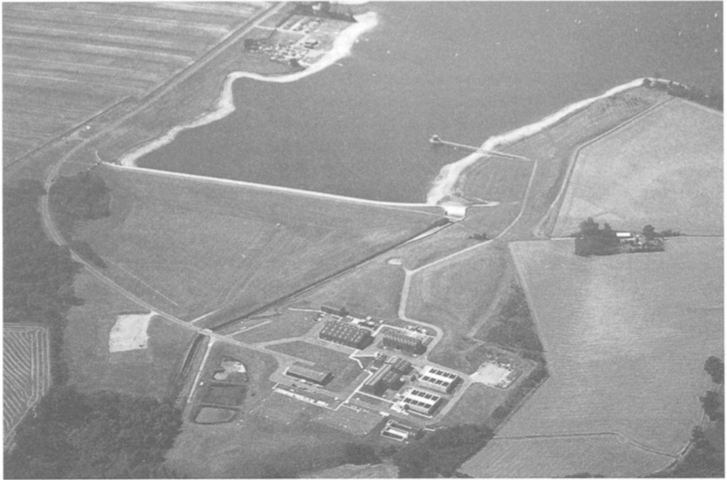
Alton reservoir formed by 24 m high earth dam, with 46 MI/day treatment works in foreground built 1987 for Anglian Water, UK. (Engineers: Binnie & Partners)
