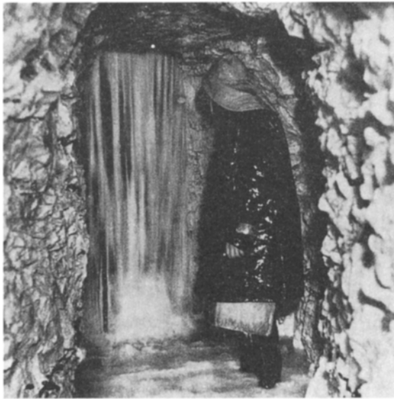
A good water-yielding fissure encountered in a chalk adit. (Contractors: George Stow & Co. Ltd., Slough, UK)
