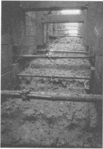
Puddled clay filling to a dam cutoff trench A pugmill producing puddled clay
