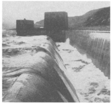
Illustration of wave spray overtopping the crest of a dam during storm conditions and wave discharge to spillway. Loch Quoich dam of the North of Scotland Hydro-Electric Board. (Photos: Richard Costain)
