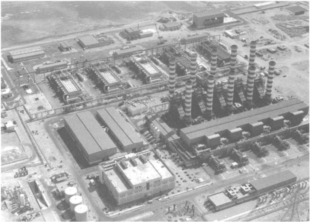
A combined 150 Ml/day five-stage seawater flash distillation plant with 608 MW output, Ras Abu Fontas, Qatar, 1999. (Engineers: Mott MacDonald, Brighton UK. Contractors: Weir Westgarth and ABB, UK)
