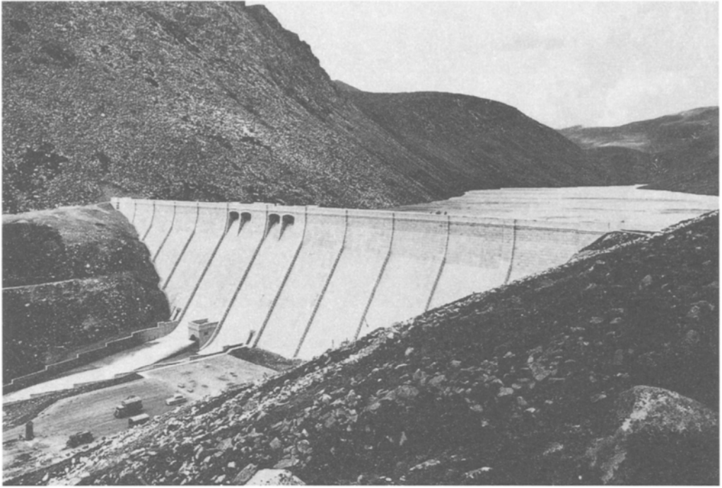
Upper Silent Valley 38 m high concrete gravity dam, with precast concrete block facing, built for Belfast 1957. (Engineers: Binnie & Partners)
