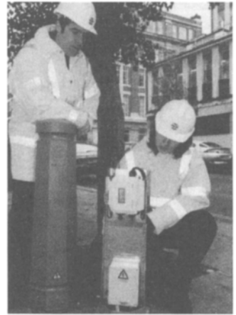
For district metering an AquaMaster can be buried directly in the ground with the electronics housed in a street bollard as illustrated above
