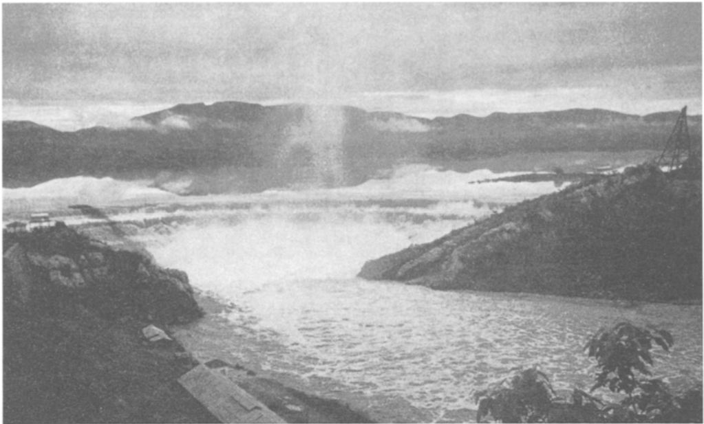
Oros earth dam, Brazil, overtopped by flood during construction 25 March 1960. (Photo: Water & Water Engineering)
