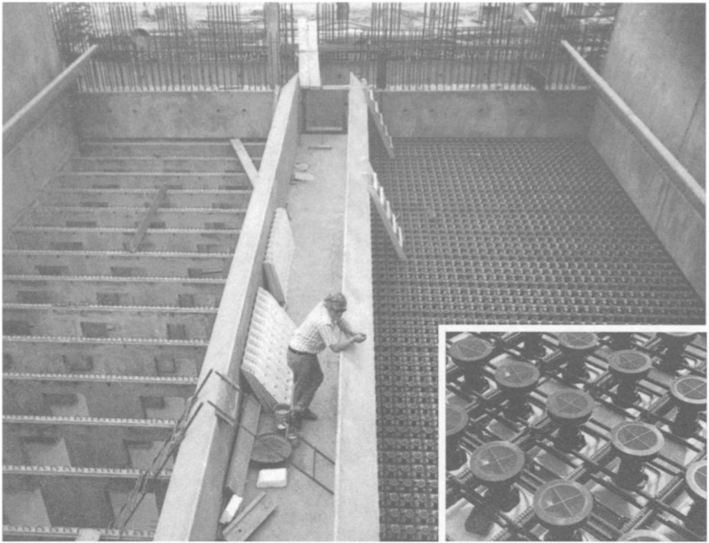
A plenum floor for a rapid gravity filter under construction (see Fig. 7.14). Left shows dwarf walls constructed for supporting pre-formed plastic formwork for the underside of the filter floor. On the right, nozzle bushes (with sealing caps) are shown inserted into pre-formed holes in the floor formwork with a matrix of rebar reinforcement in place. The floor is then concreted flush with the sealing caps, and after curing, the sealing caps are removed and the nozzle stems and domes screwed in to a uniform level. (Paterson Candy Ltd., Isleworth, UK)
