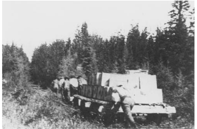
Before Bob Starratt took over, sheer "bull" muscle power was used at the Hudson's Bay Company log tramway on the Root Portage between Lac Seul and Lake St. Joseph. These men pushed a flatcar, with tireless wheels, and loaded with crates of four-gallon cans of gasoline, over portage poles.
