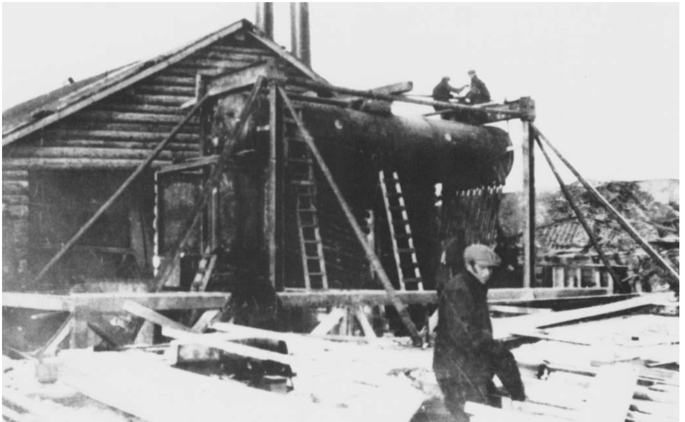
Workmen install a steam boiler at the Howey mine at Red Lake in 1927. That summer Howey sank a 200-metre three-compartment mining shaft 2 metres by 5 metres with a steam-powered mining plant, consisting of two 60 horse-power Inglis locomotive-type
