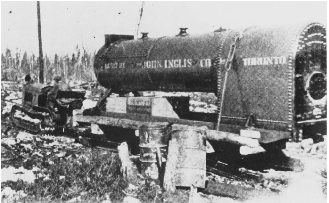
It took two Fordson tractors to haul this 60 horse-power Inglis steam boiler from Hudson to the Howey
