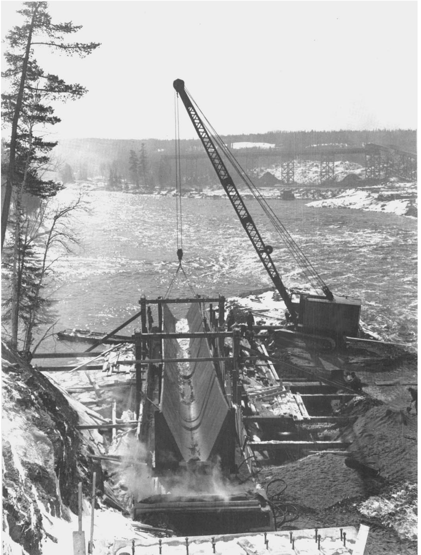
Construction of a flume at Pine Portage.
