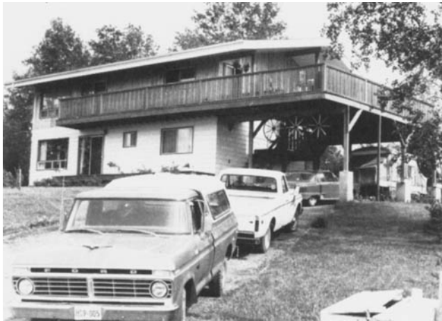
This 1980's suburban-style house, with a spacious top deck and feeling of almost stately stability, shows how far modern Red Lake (population well over 2,000) has advanced from the helter-skelter, gold rush days. With its fine hospital, schools, airport and two richly productive gold mines, it's now the sort of town where young and old miners like to settle down.
