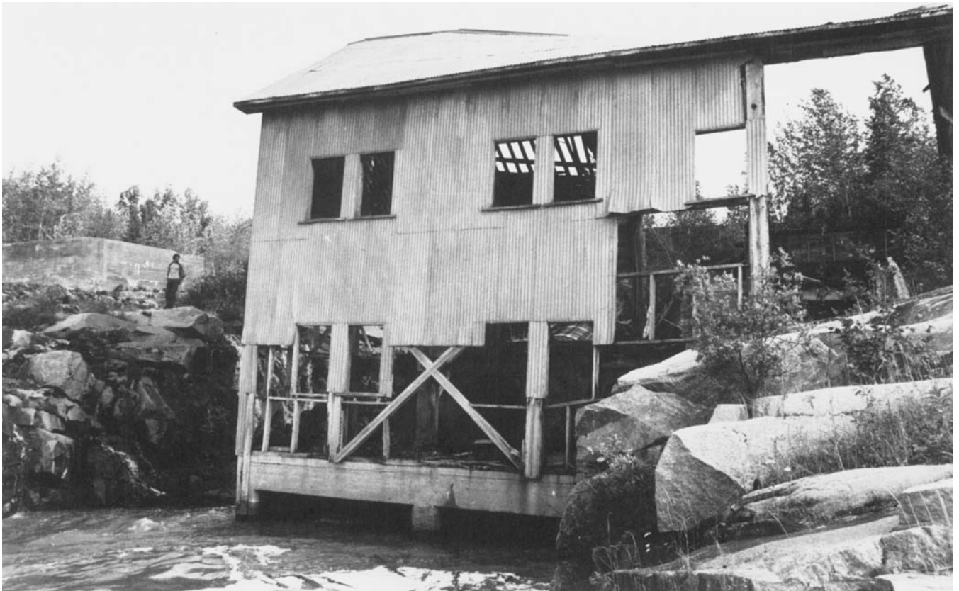
Power Plant for the Berens River Gold Mine on Northwind Lake. This mine (open from 1939-48) was one of a few to generate its own hydro-electric power.
