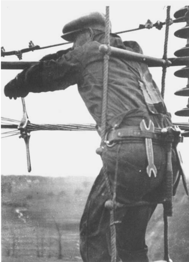
Repairing the lines in 1932.
