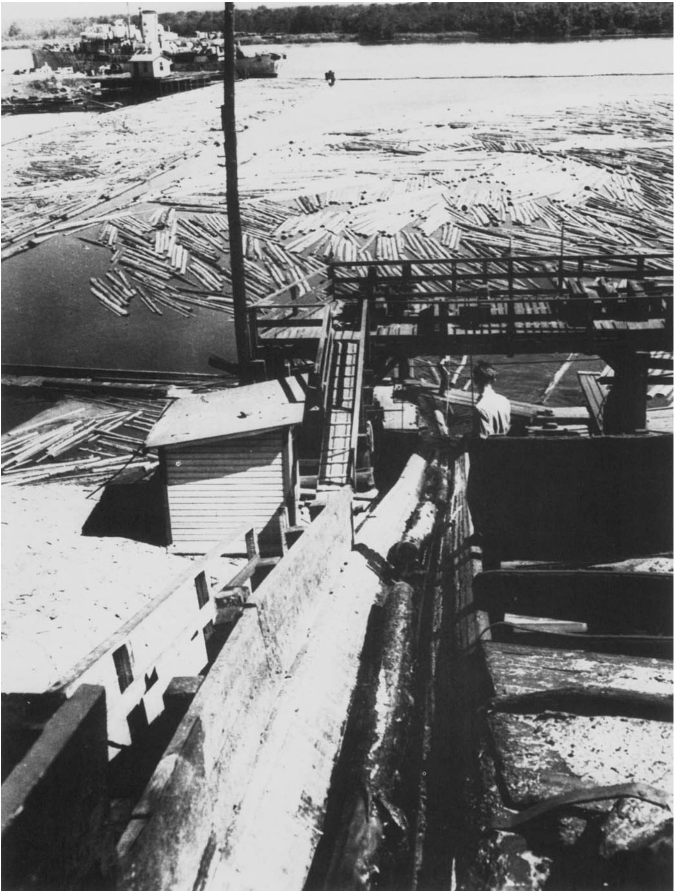
A jack ladder — a form of escalator — carried logs from the boom in the Kamanistiquia River into the
