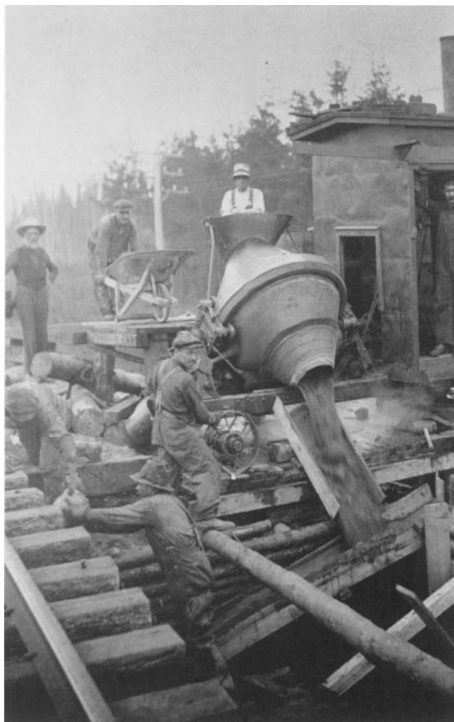
Laborers were paid $1.25 per day to pour concrete for this CPR track underpinning near Nipigon at the turn of the century.
