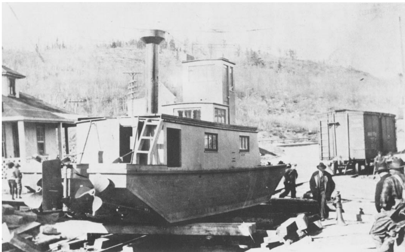
Logging alligator in makeshift drydock, Chapleau 1919.
