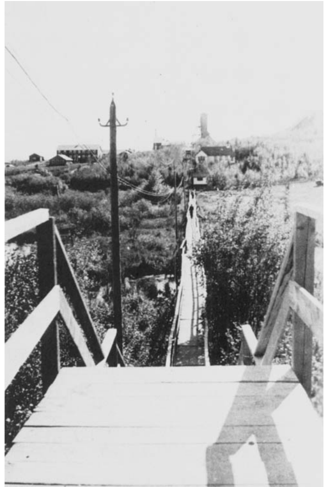
This "Duck Walk" crossed the swamp in the foreground over to Howey Mine. In front of the mine are the Catholic Church and the Provincial Police Station.
