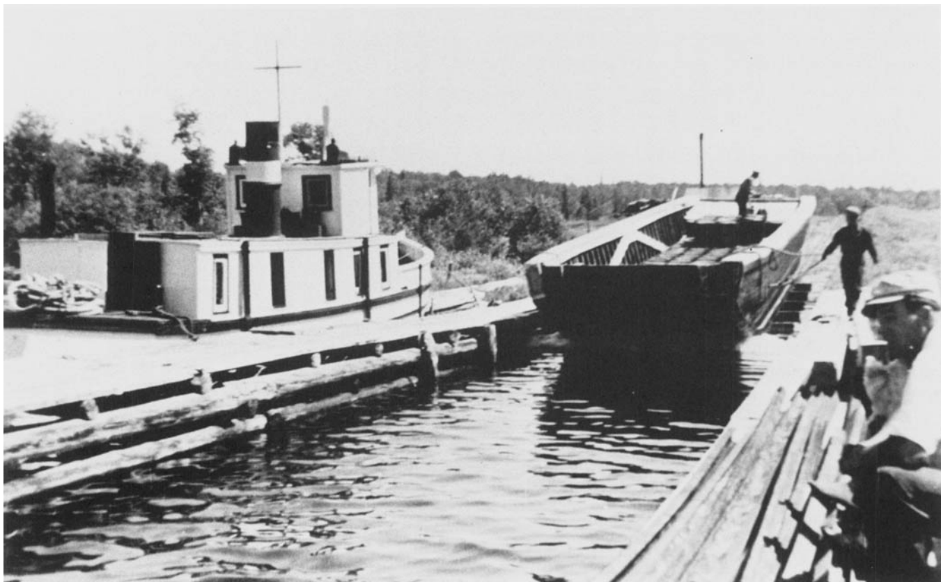
The barges of freight used to be steam-winchd over land at Sam's Portage — one of four portages between Ear Falls and Red Lake — using this marine railway.
