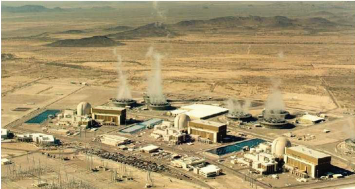
Palo Verde Nuclear Generating Station. SOURCE: Photo courtesy of Henry Day.
